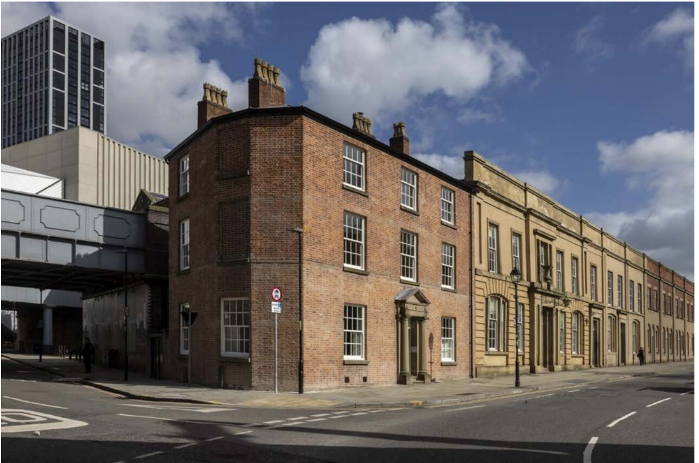
The Station Agent's House in 2024, on the corner of Liverpool Road and Water Street. The 1830 Coach Offices/Passenger Building runs alongside it to the right; to the left, the 1905 replacement for George Stephenson's Water Street road bridge is a continuation of the Irwell viaduct, and carries the track to the former high-level passenger platform behind the house.
