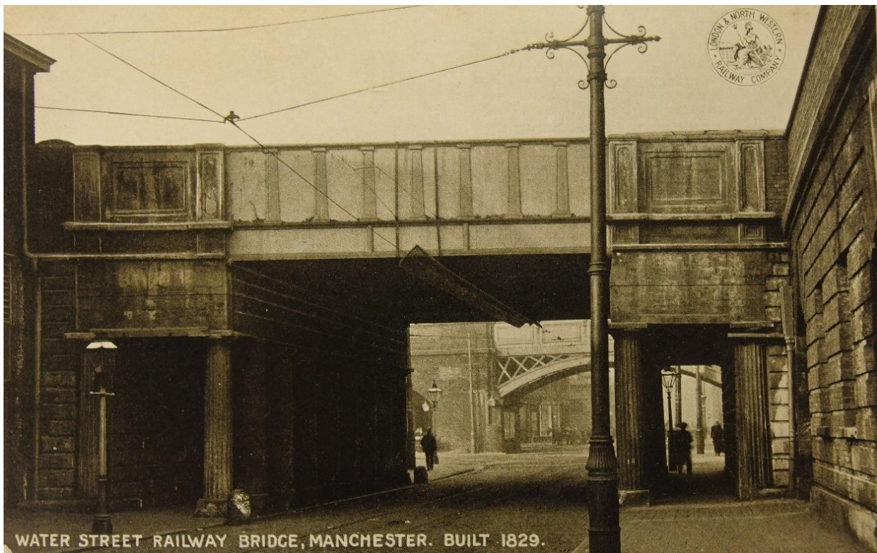
A pre-1904 postcard of George Stephenson's innovative cast iron bridge over Water Street, supported on cast iron Doric columns, which, wrote a contemporary, 'gave the interior the appearance of an elegant classical temple'.
