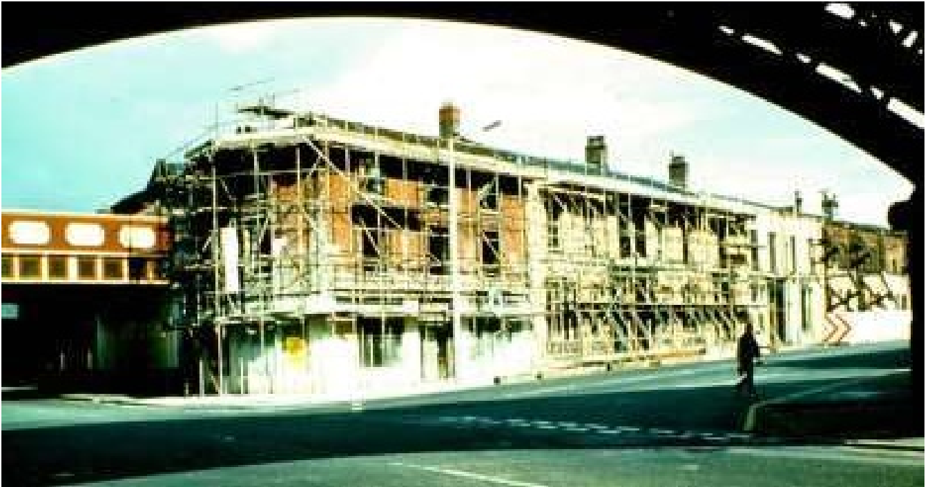
The station buildings under repair by the museum, c1980.
