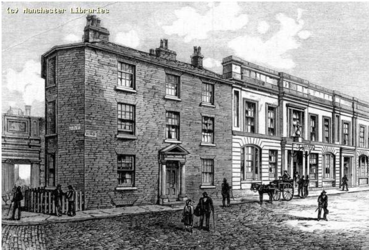
Station Agent's House c1860. The colonnade under Stephenson's original Water Street bridge is still in place.
