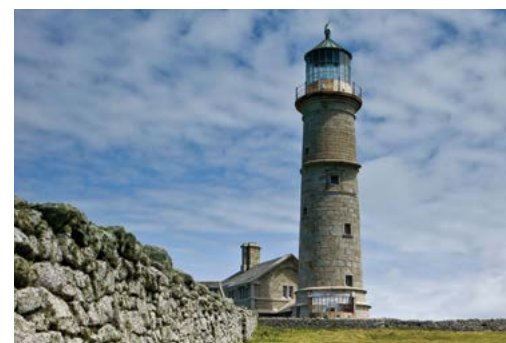
Restoration began at the Old Lighthouse on Lundy
