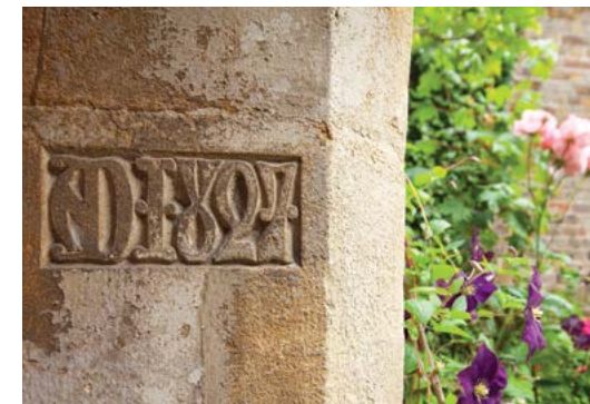
St Edward's Presbytery was on the Buildings at Risk Register
