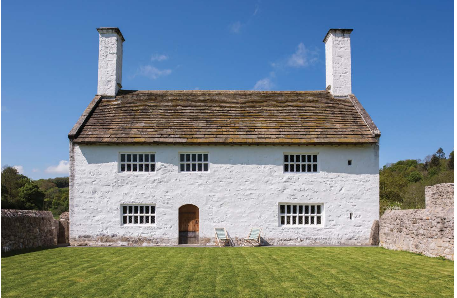
Above: Landmark's restoration of Grade II* listed Dolbelydr, Denbighshire, rescued it from roofless ruination, see opposite.
