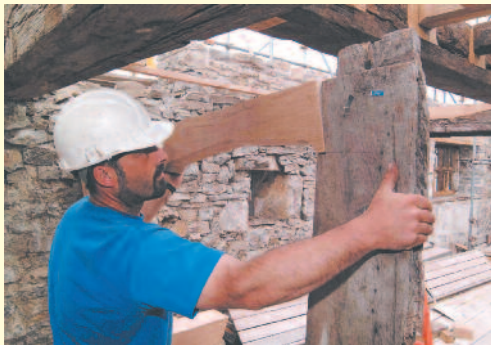
Piecing together Dolbelydr's internal timber frame.
