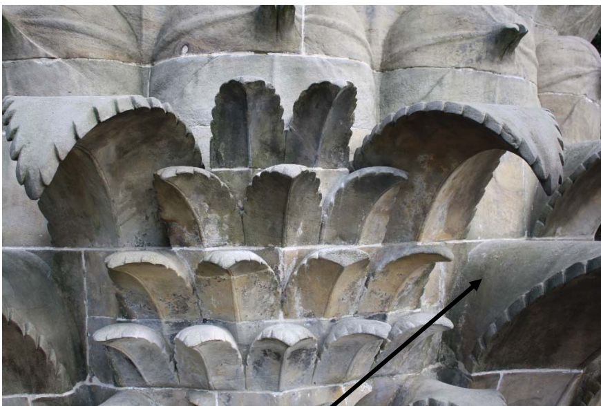
This photo shows the curve of the leaf – the clever design that allows any rainwater to run straight off the stonework. When water collects on roofs, it can cause leaks – this design stops that from happening.
