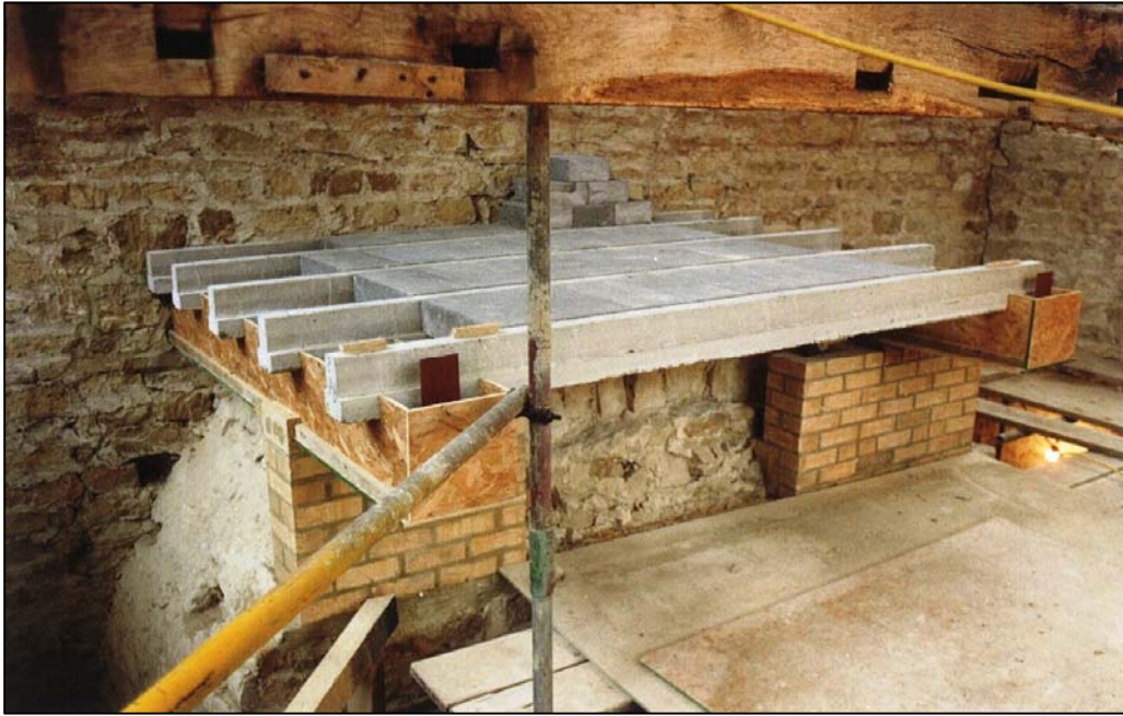
The platform for the new bathroom
