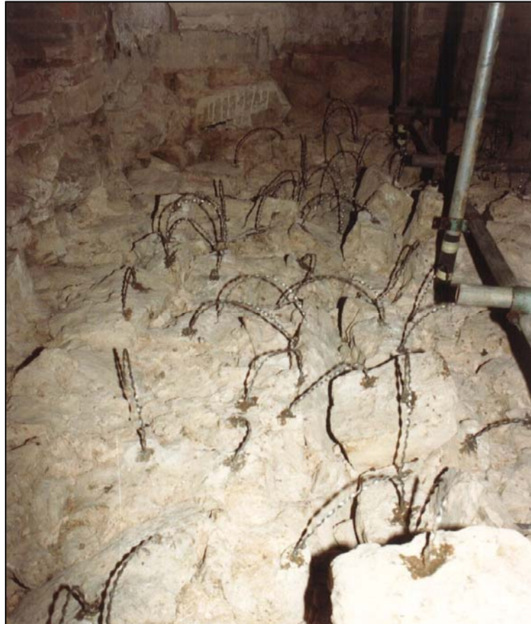
The “metallic hedgehog” of ties supporting the rock work of the bath chamber
