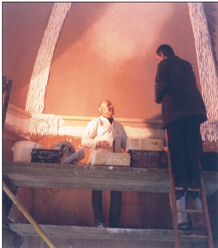
Bill Salter, the plasterer, with the architect, William Hawkes
