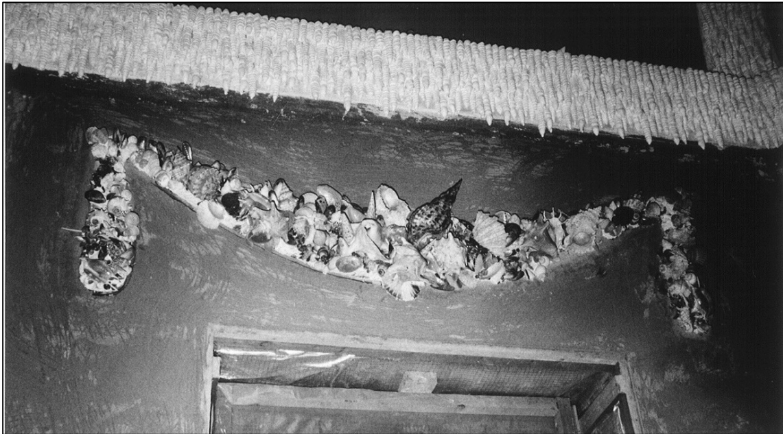
An unfinished festoon, soon after it was mounted on the wall. The smaller shells, and those that project over the plaster, were added in situ, as below and opposite.
