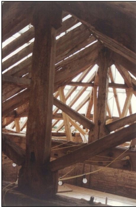
The roof structure under repair
