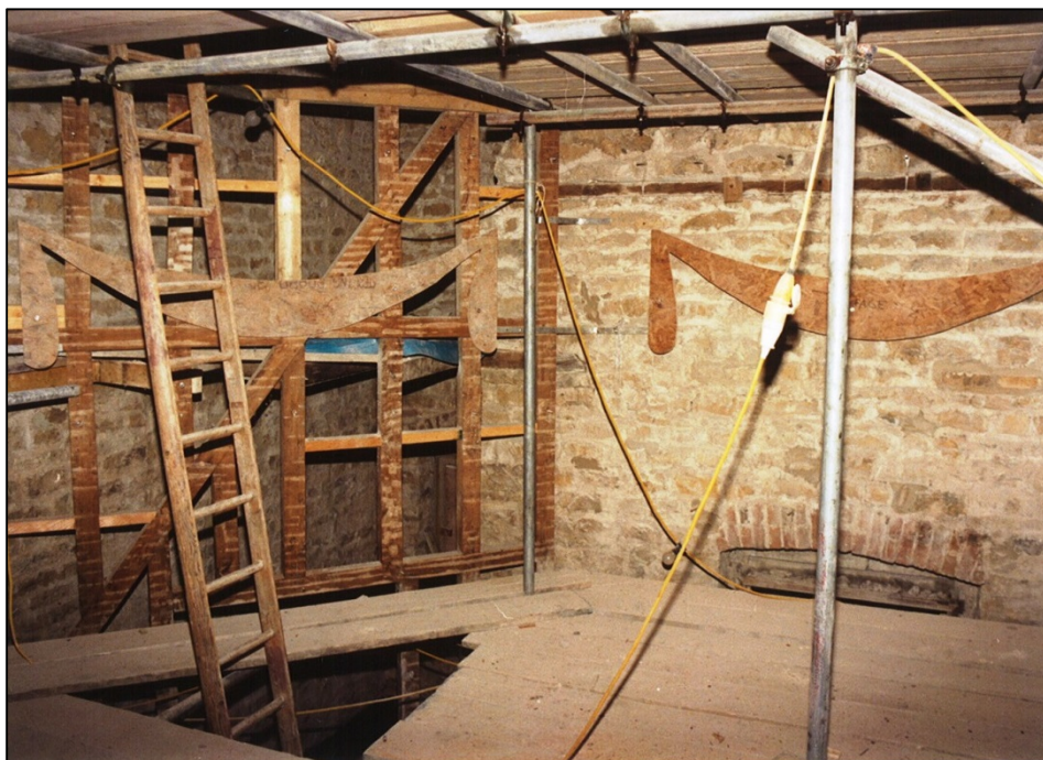
The boards marking the original positions of the festoons later served as mountings against which to fix the restored ones.
