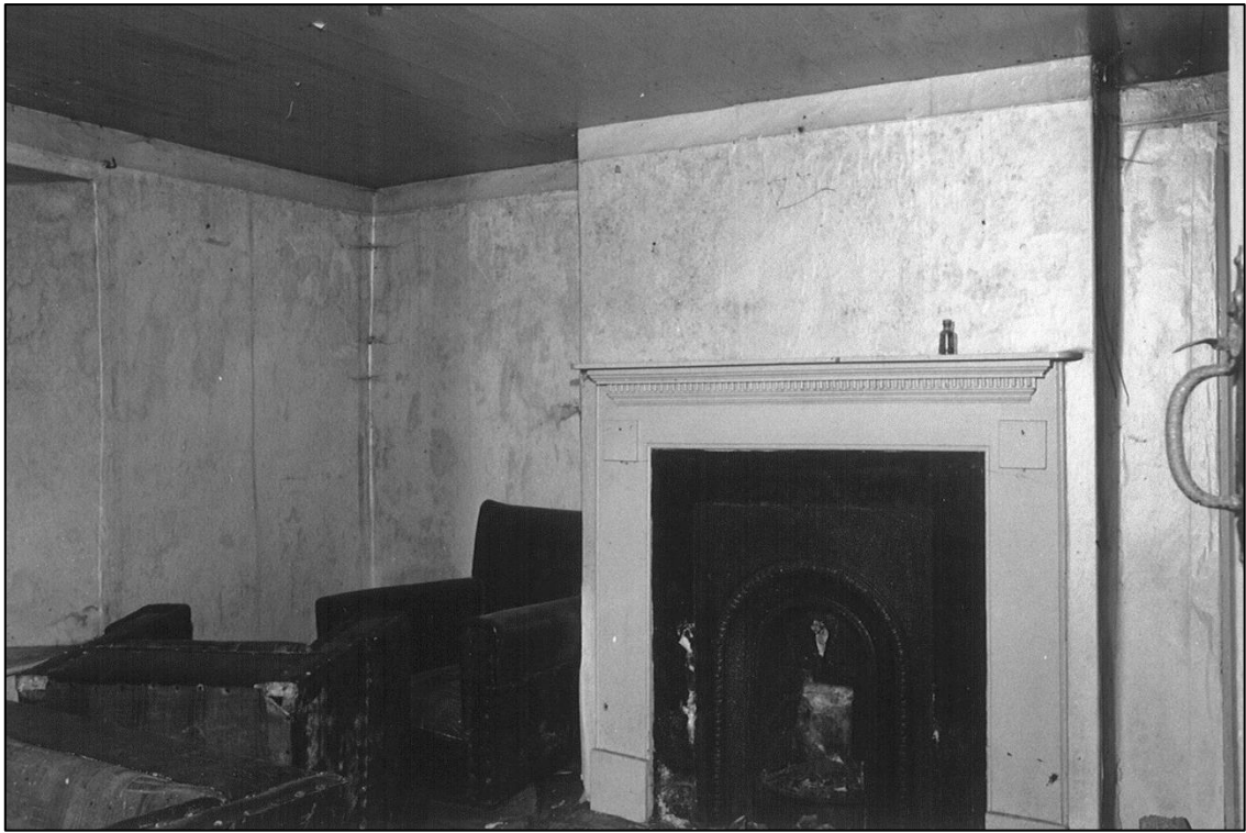
Bridge Cottage before restoration
