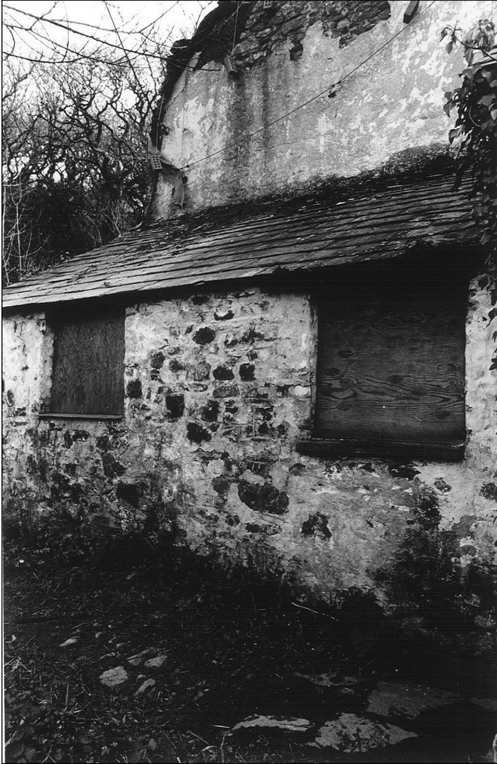
Bridge Cottage before restoration
