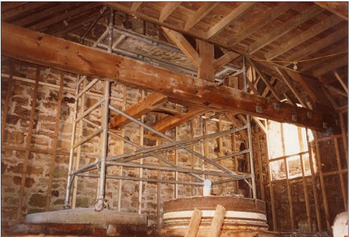
1992. The beam has been repaired.
