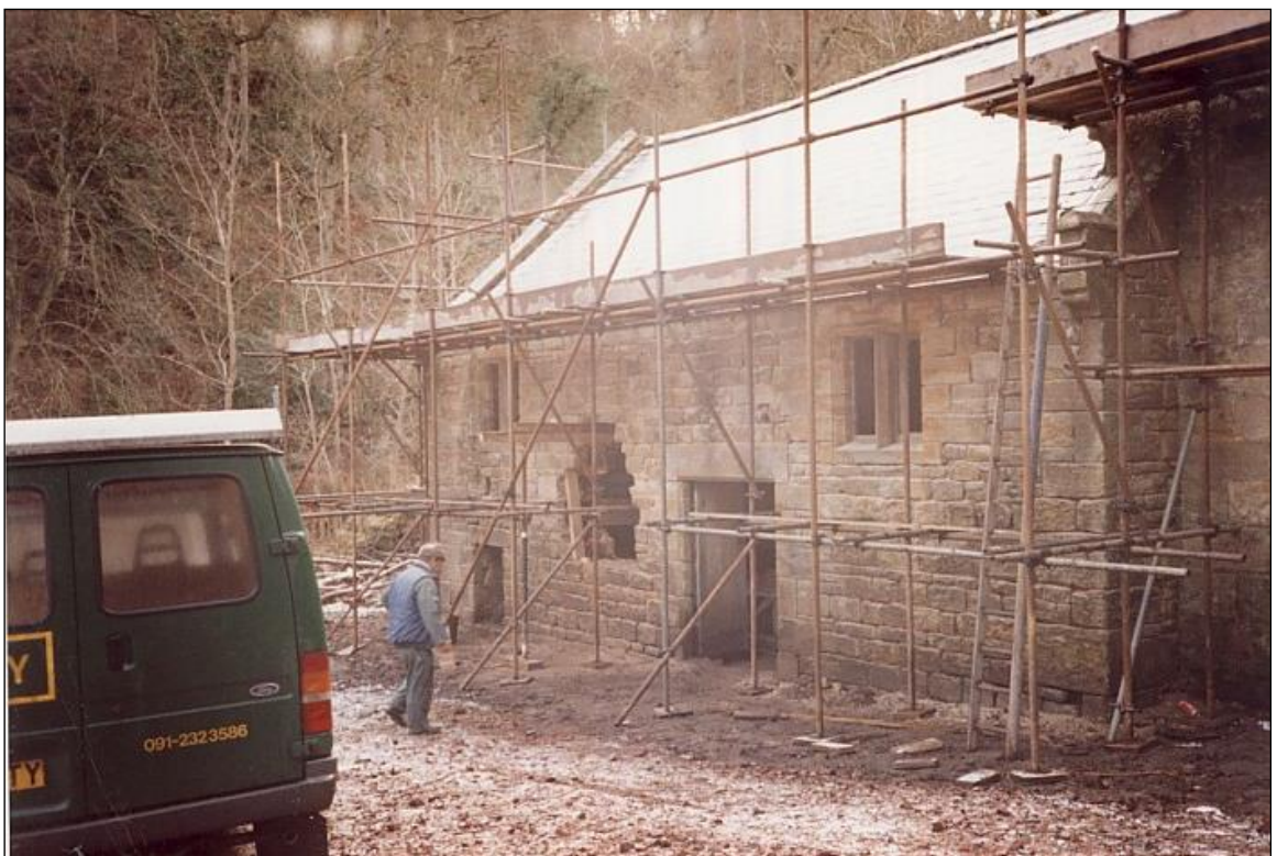
The new window being made.
