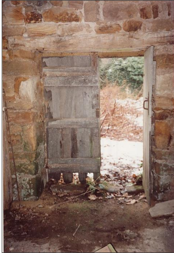
The old mill door.
