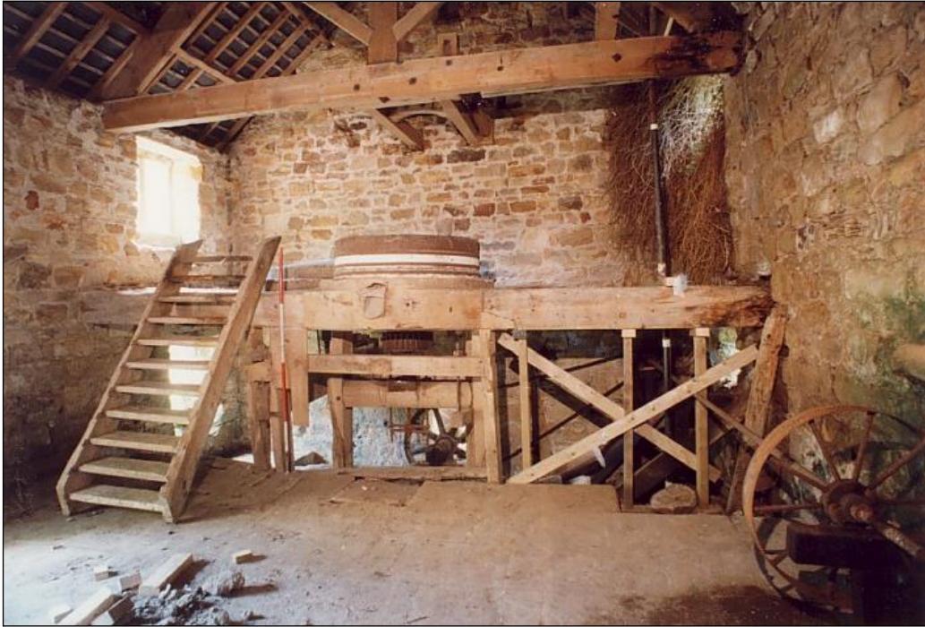
The south end before the new floor was laid.
