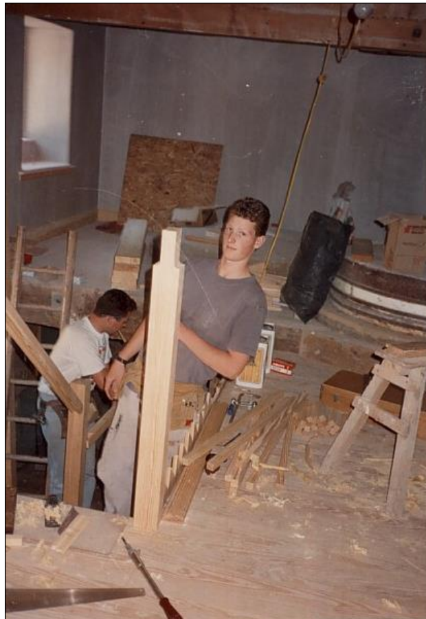
Working on the new staircase. The new floor is in place.
