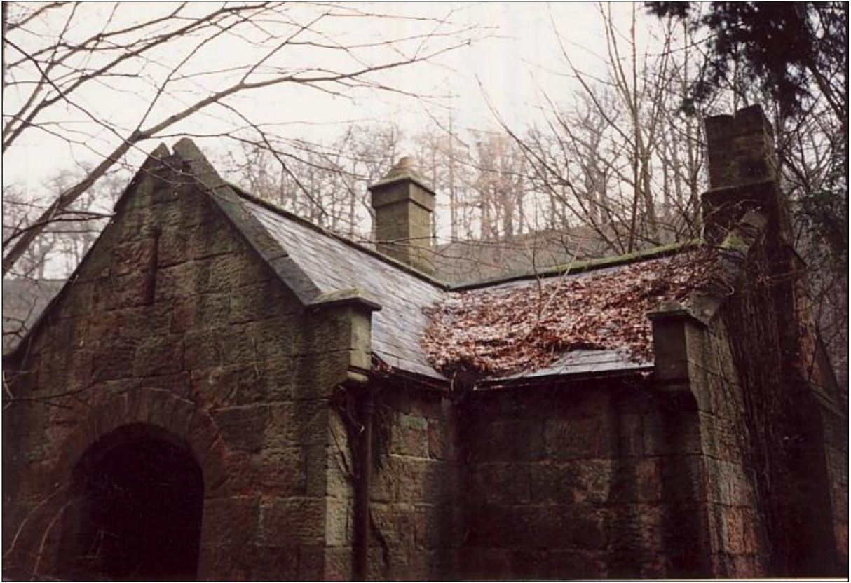
The north front in 1989. All three acorns are missing.
