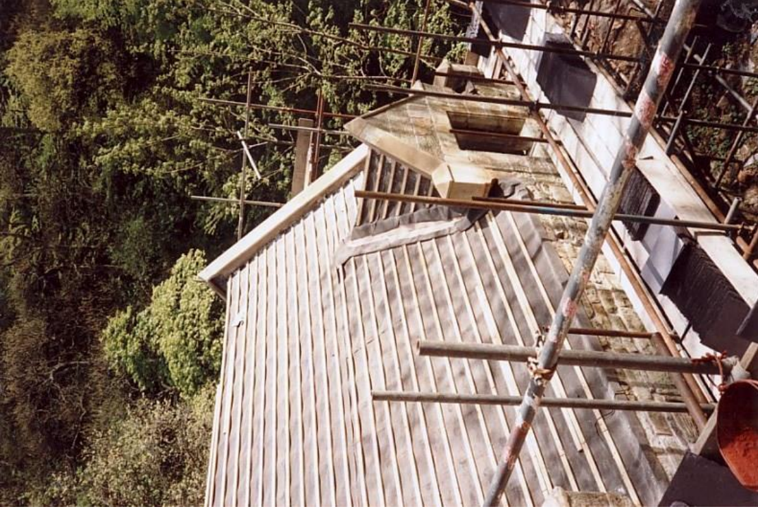
The window at the south end of the west front. Part of the cope had gone. It was found on the ground and replaced.
