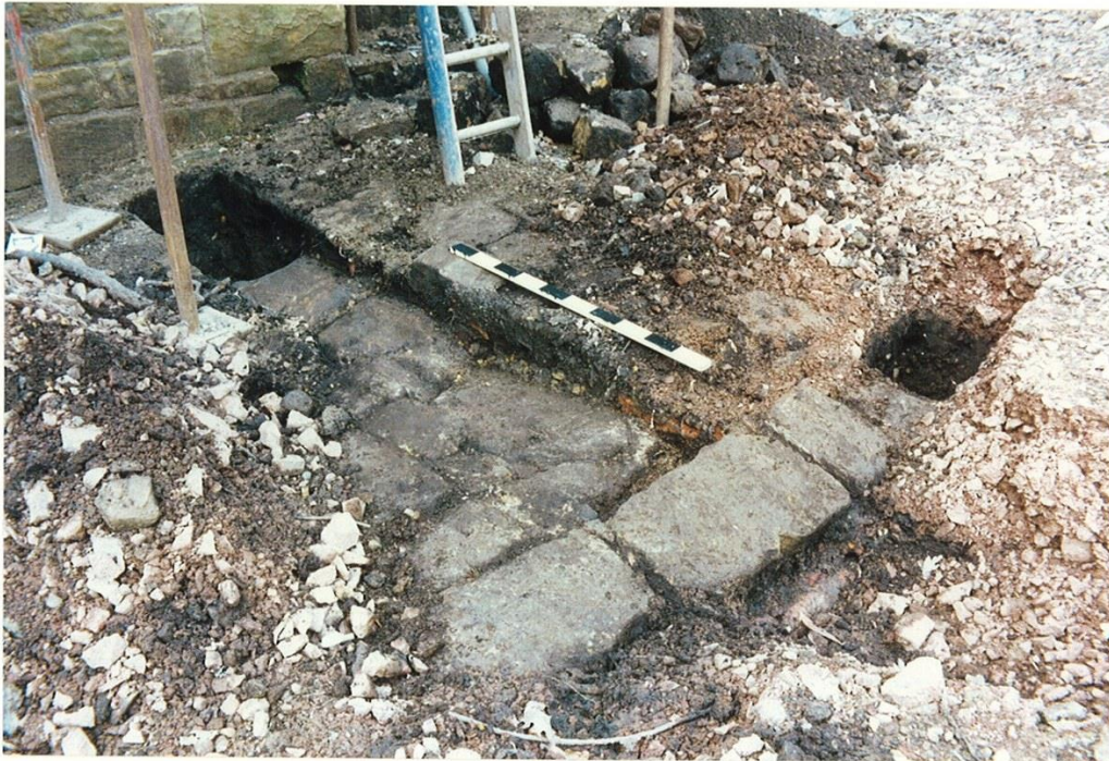
The trial trench and exposed hardstanding looking north-west
