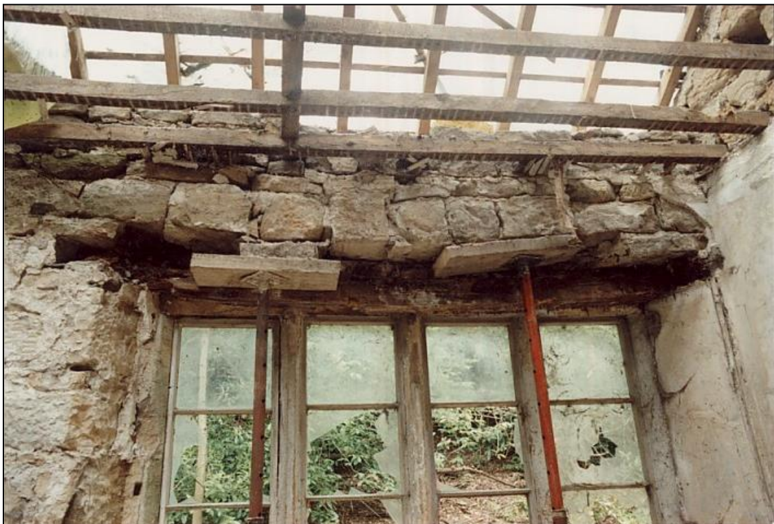
The lintel removed and about to be replaced.
