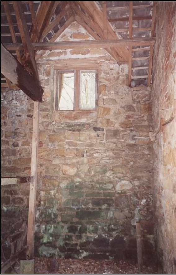
The small bedroom showing the original level of the floor. On the right the bricks show the line of the old flue, leading to the chimney in Turner's picture. The window below the dormer is still blocked up.
