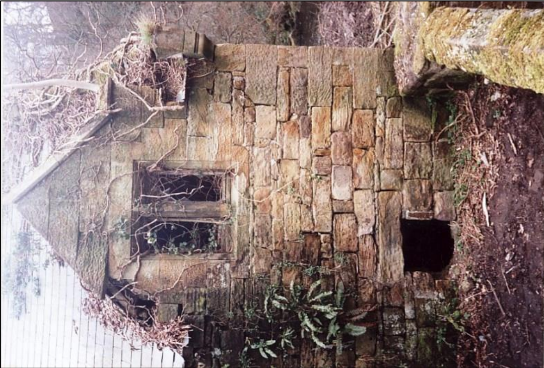
The window at the south end of the west front. Part of the cope had gone. It was found on the ground and replaced.
