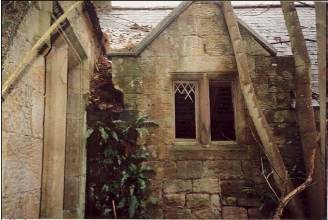
The window at the north end of the west front. The diamond panes had wooden astrigals, not lead, and they have been replaced as they were, in wood. In the top photograph traces of the old 18th- century window can be seen, blocked up when the dormer window was put in. In the bottom photograph it is being
