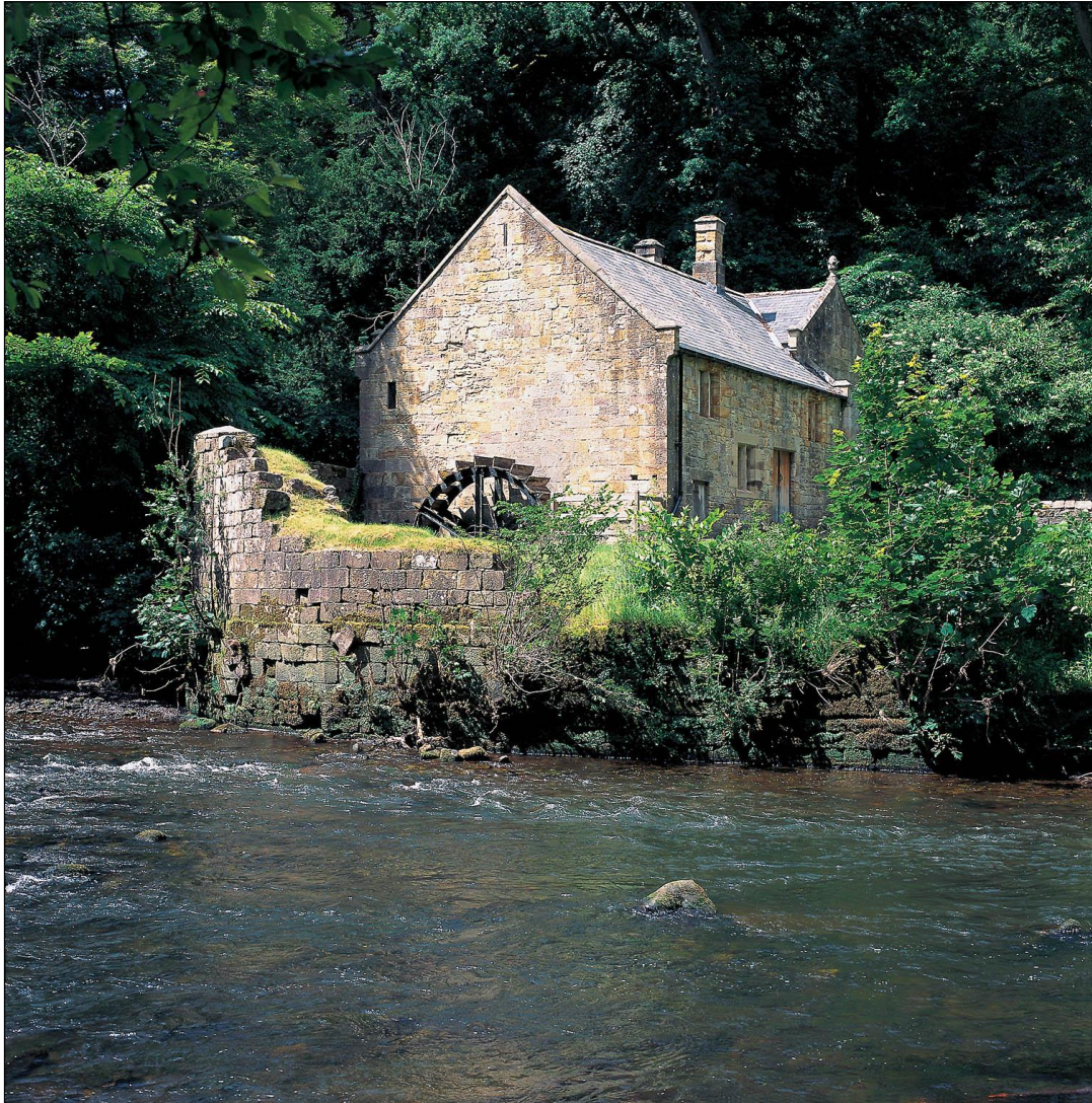
Brinkburn Mill probably stands on the site of a medieval mill, within the ancient precinct walls of Brinkburn Priory.
