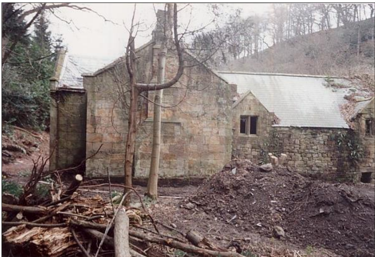
West front, ground being lowered.
