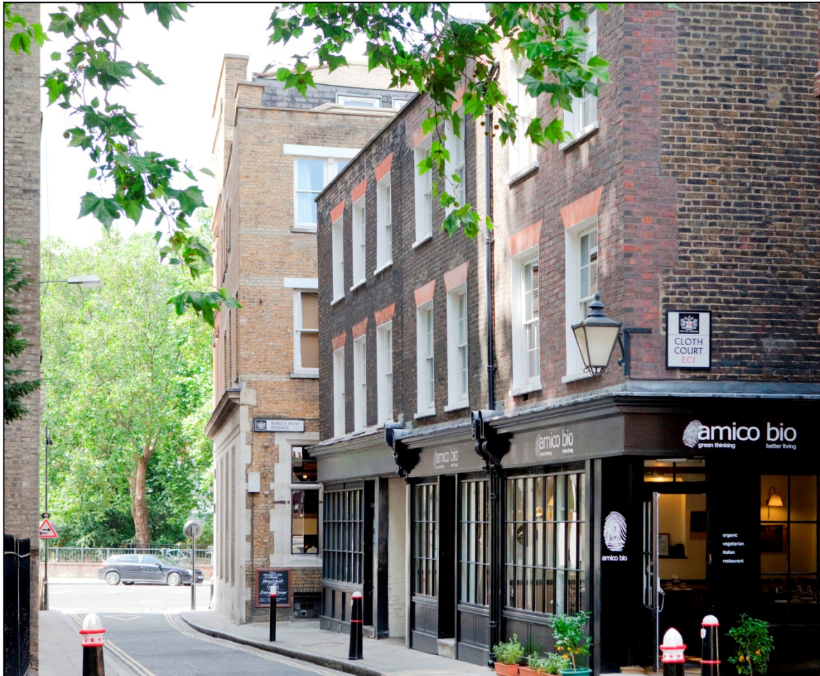
Re-faced in brick during the 18th century, Nos. 39-45 Cloth Fair are hold late 16 th -century houses at their core, built on a once crowded medieval street plan and rare survivors in the City of the Great Fire of London.
