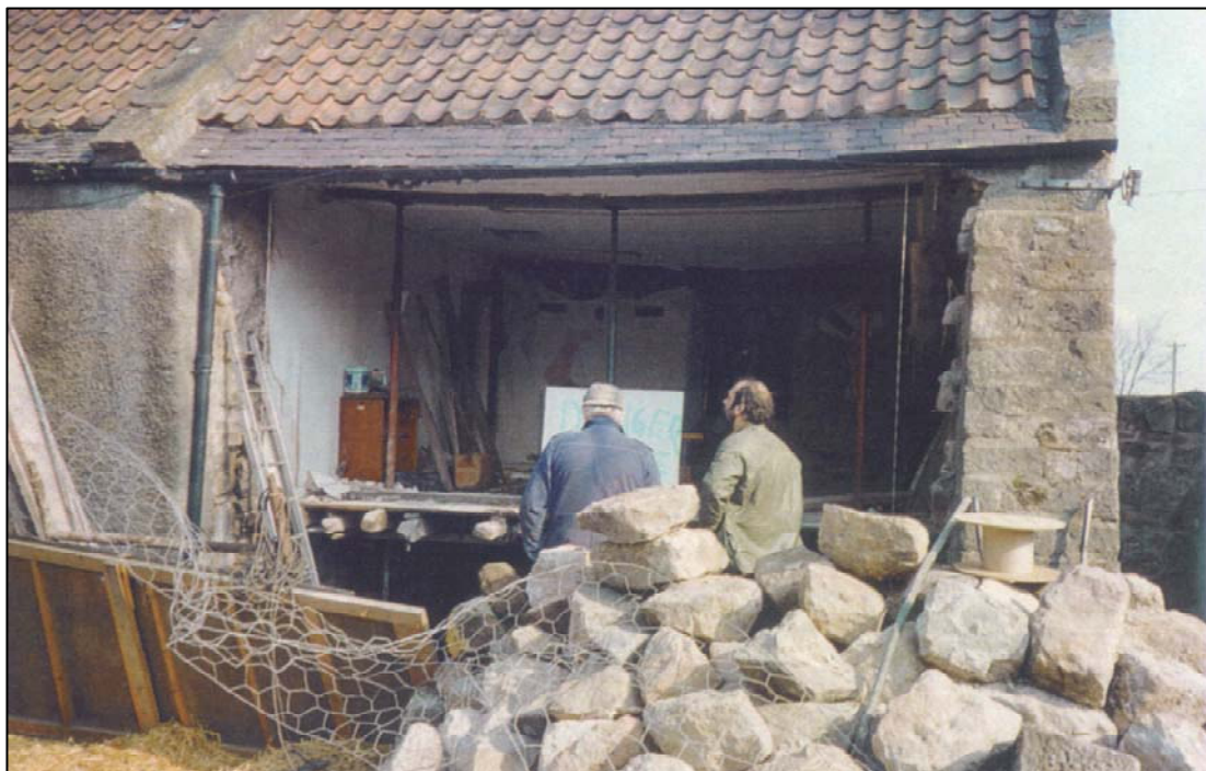
South wall of kitchen before rebuilding.
