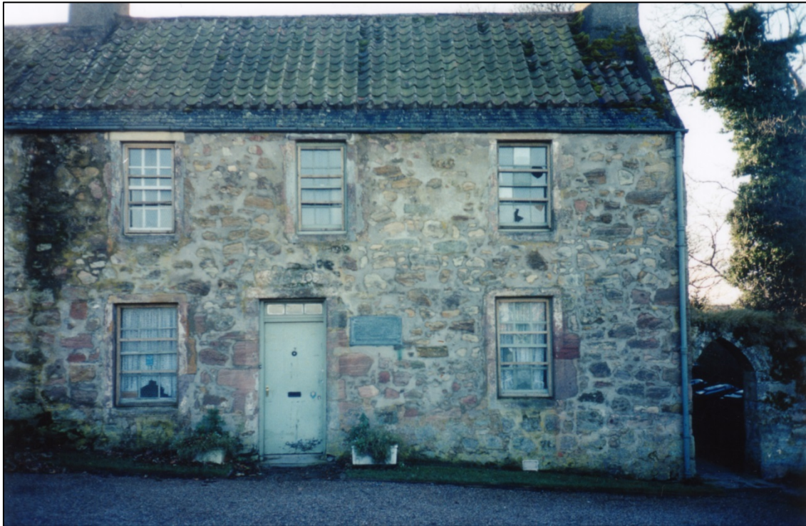
Collegehill House before work began
