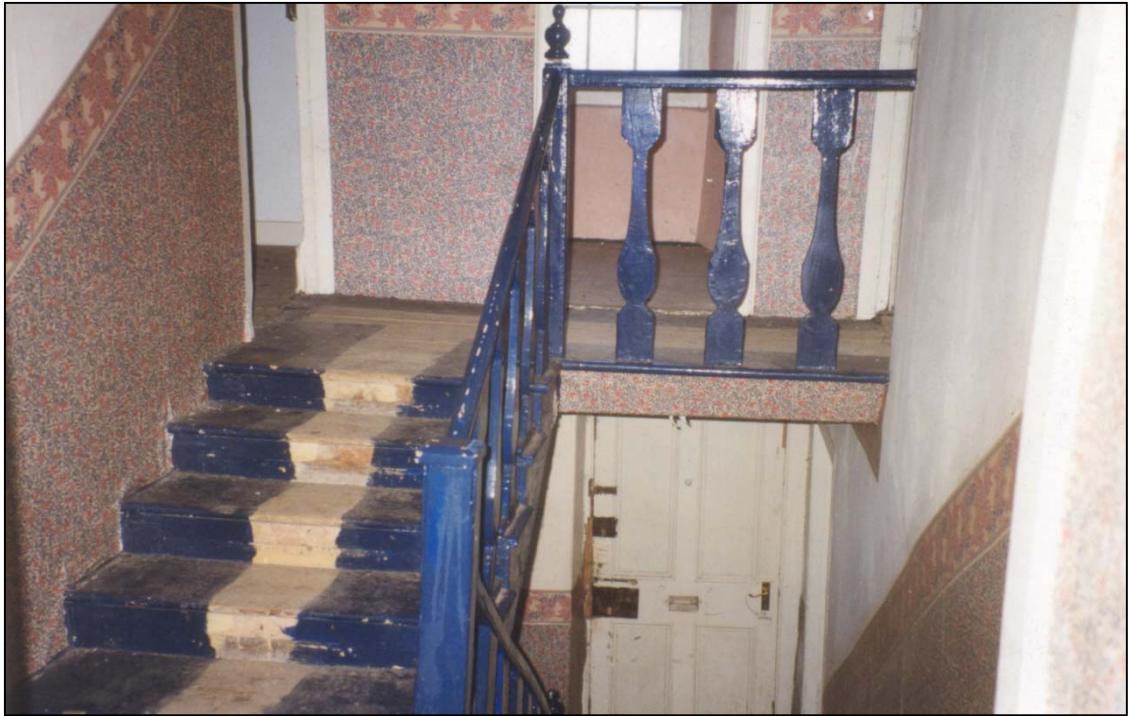
The first floor landing before work began.
