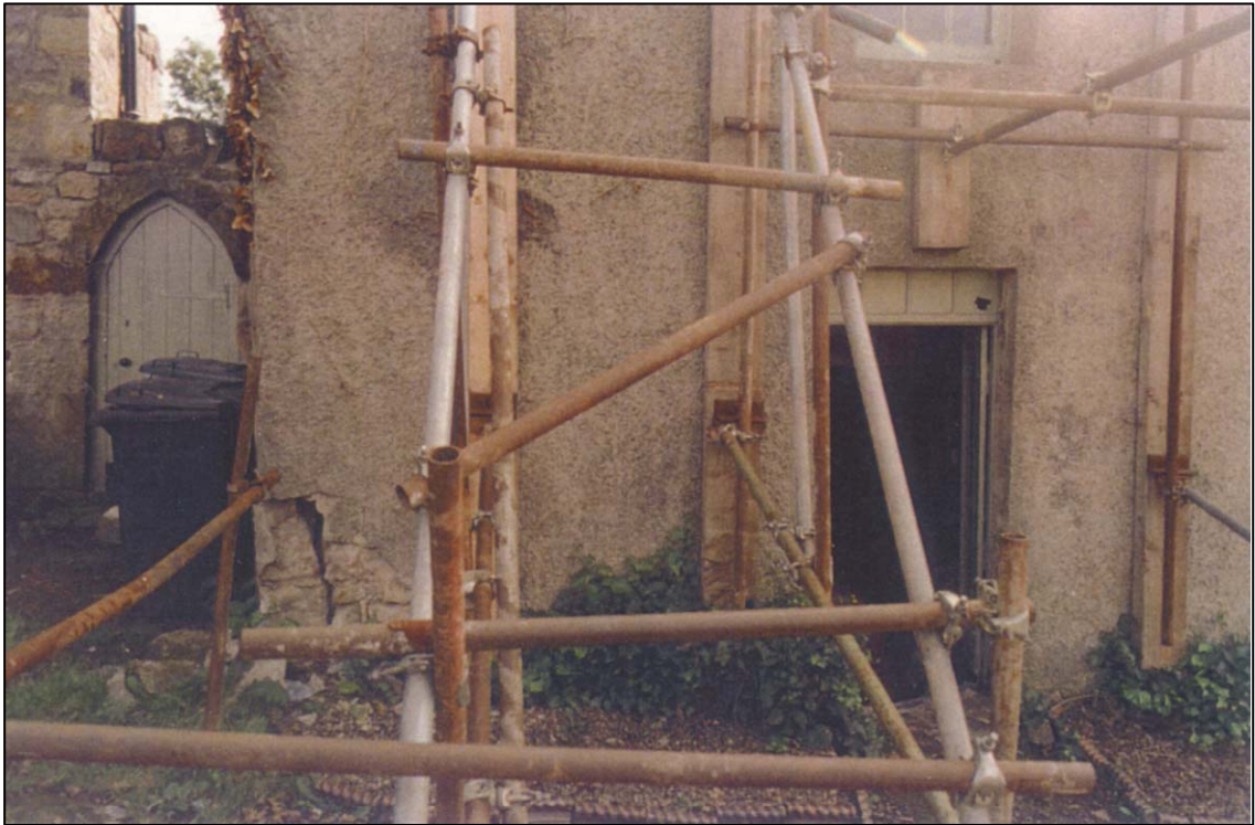
North east corner
