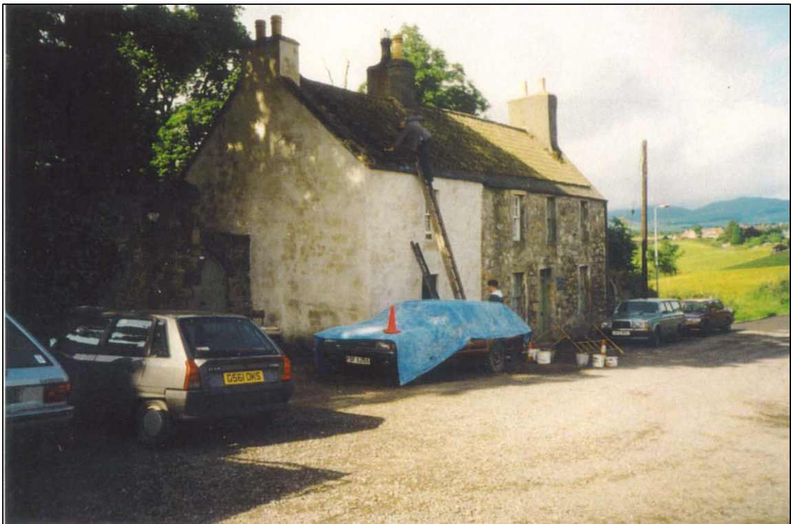
Working nearing completion, the east end now harled.
