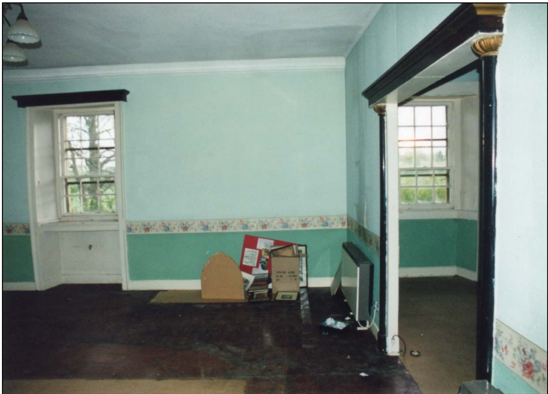
North west entrance to the sitting room on the first floor. The pillars from the Prince's Theatre, Edinburgh flank the doorway.
