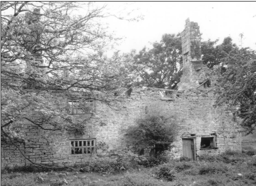
West elevation with inserted door and altered SW window.
