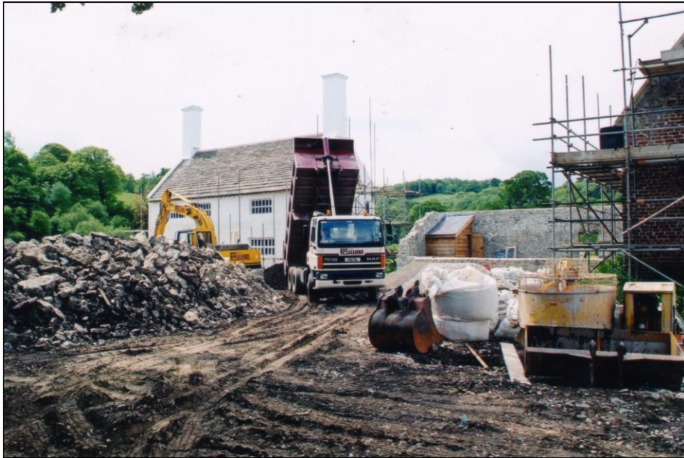
Final landscaping to correct ground levels.
