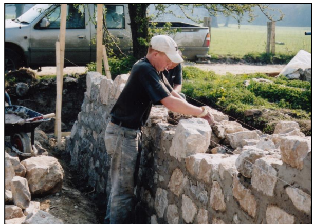
Packing the rubble core of the forecourt walls
