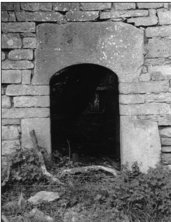
Below: The 'cyclopean' doorway, outside and in. Note the socket for a draw bar.
