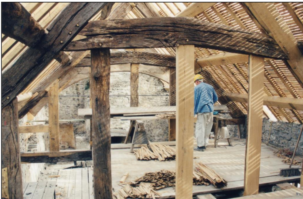
With the rafters in place, the fixing of battens could get underway (above, looking south across today's landing and below in the solar roof space).
