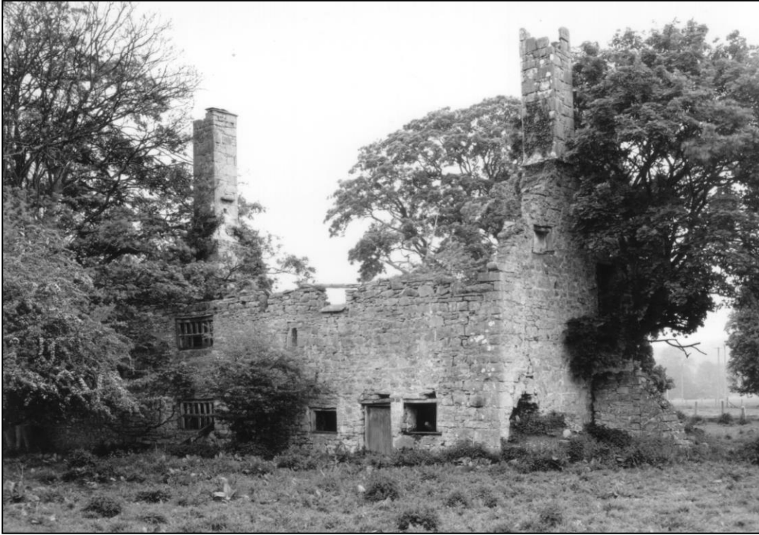
West ('rear') elevation with remains of bread oven in the SW corner and of external staircase on the west south wall.
