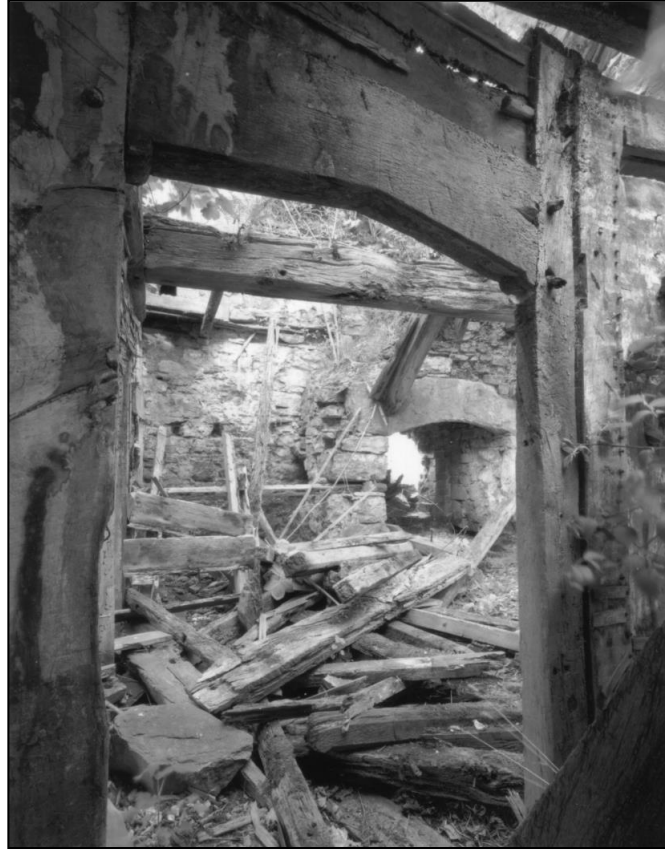
Top: View SW from passage through service room with remains of bread oven in the far corner. Its massive stone lintel was almost certainly re-used from an entrance gateway, where it now again resides.
