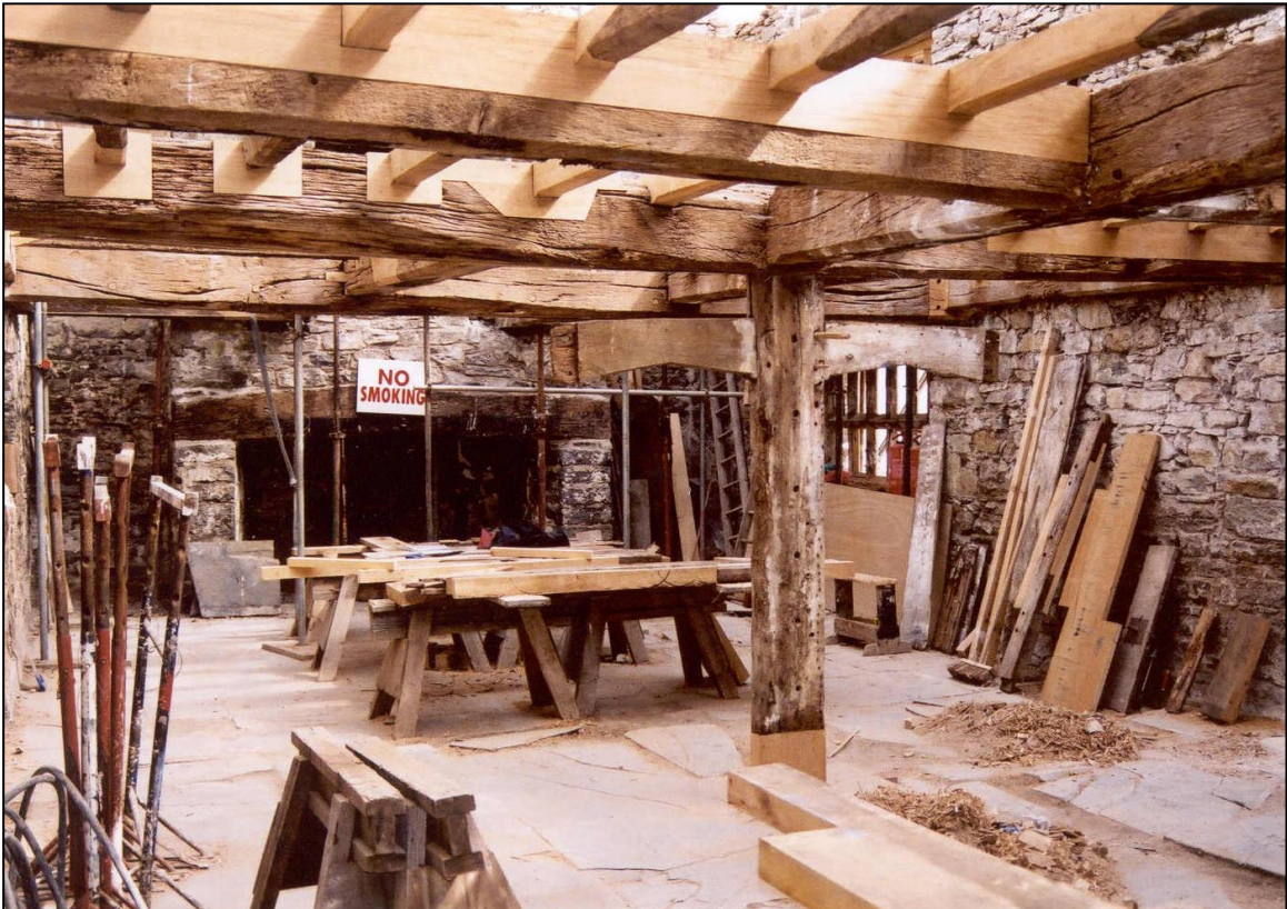
The same floor structure viewed from the hall below.
