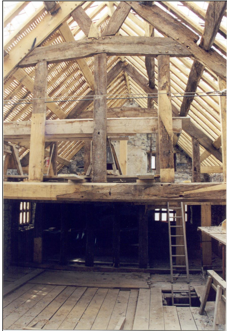
With the rafters in place, the fixing of battens could get underway (above, looking south across today's landing and below in the solar roof space).
