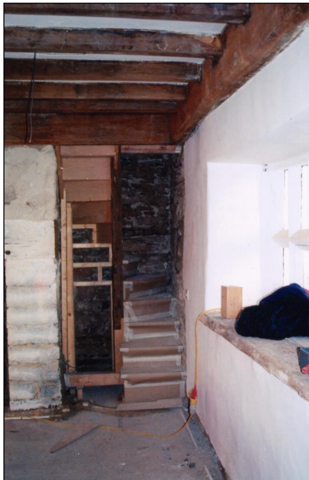
Test fire in the hall hearth – always a relief when it draws! A sample floor slate is laid out and the fretted screen above the cupboard is now installed. The spiral stairs are under construction.
