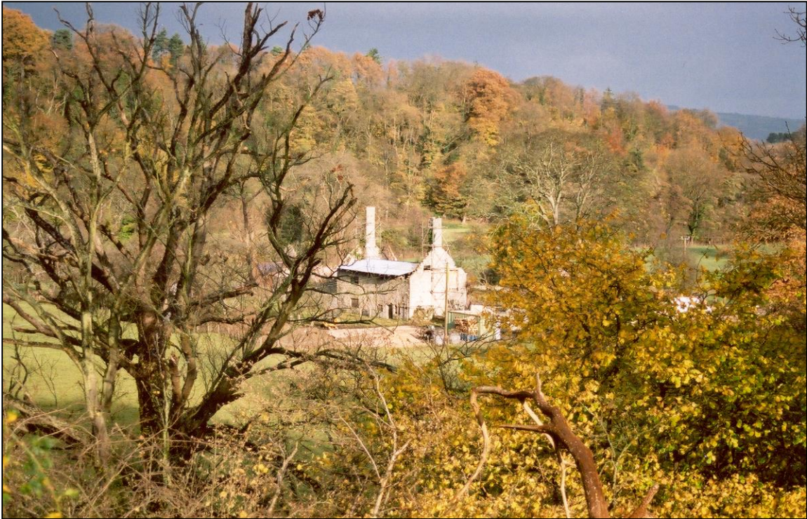
At the very beginning of work on site, autumn 2001.
