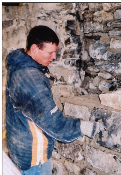
Repairs to the walls, using lime mortar.
