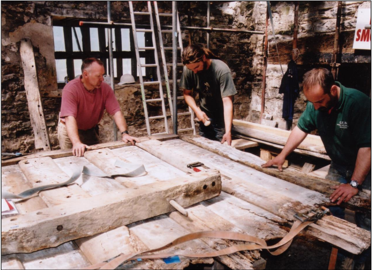
Piecing the plank and muntin screen back together.
