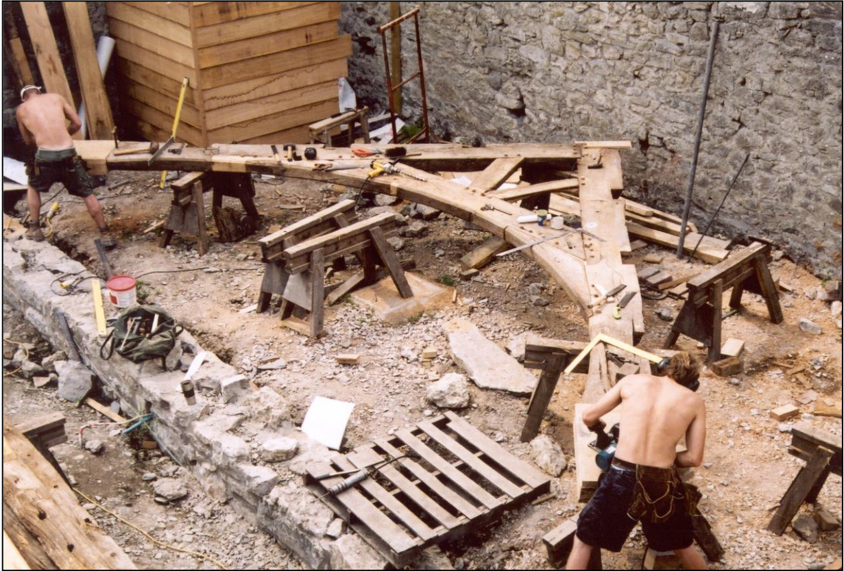
The truss was then returned to the site for final adjustments....
