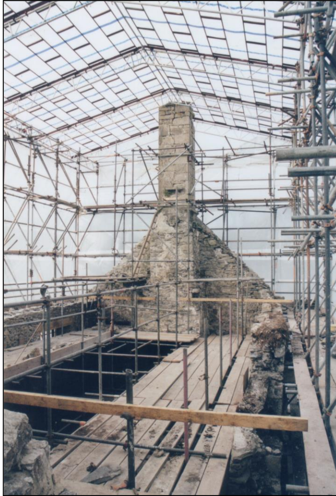
The roofspace beneath the canopy, all timbers removed.
