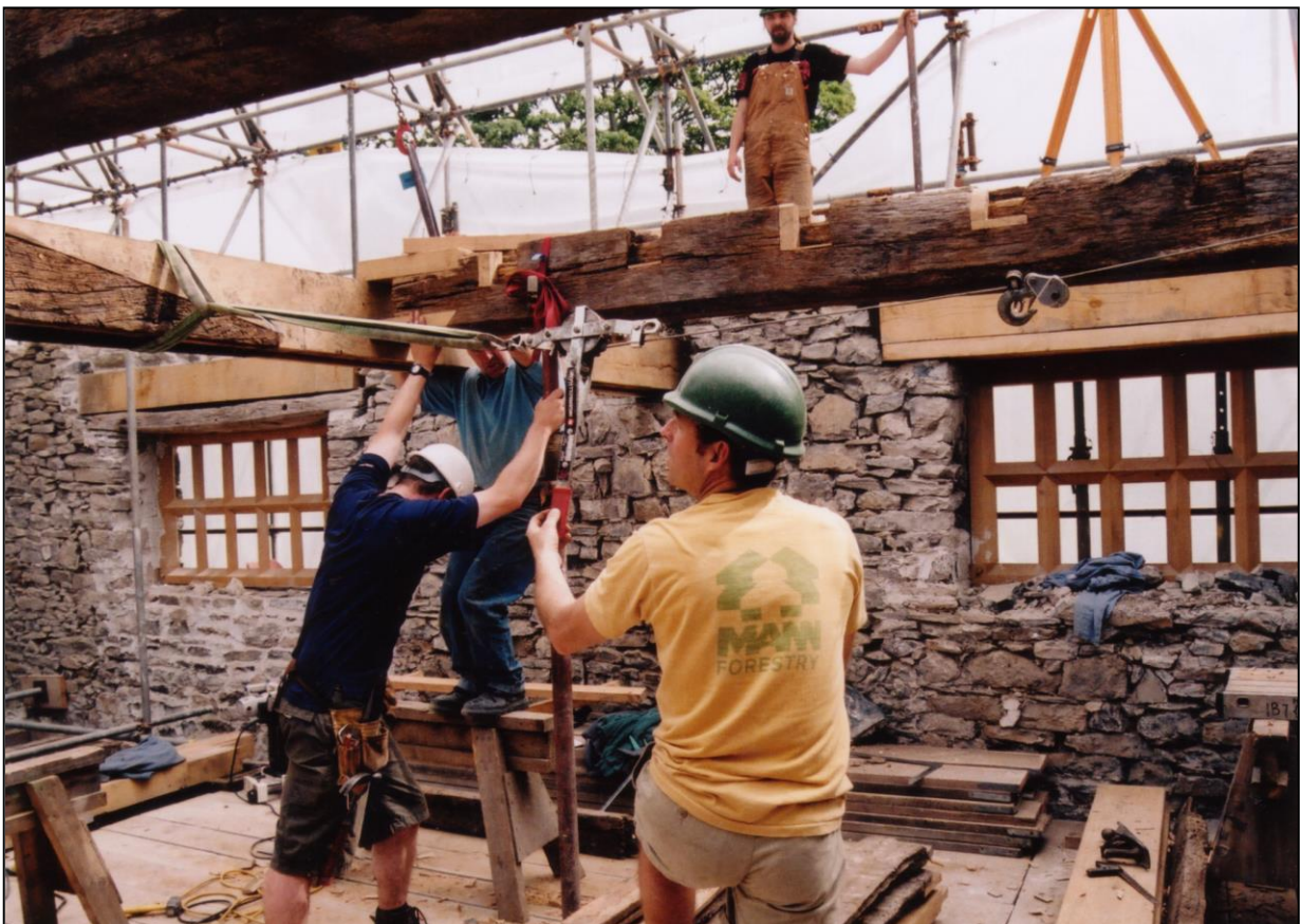
The repaired first floor joists being carefully repositioned above the hall.
