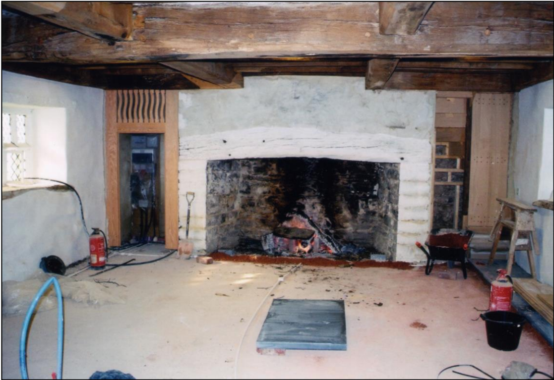
Test fire in the hall hearth – always a relief when it draws! A sample floor slate is laid out and the fretted screen above the cupboard is now installed. The spiral stairs are under construction.
