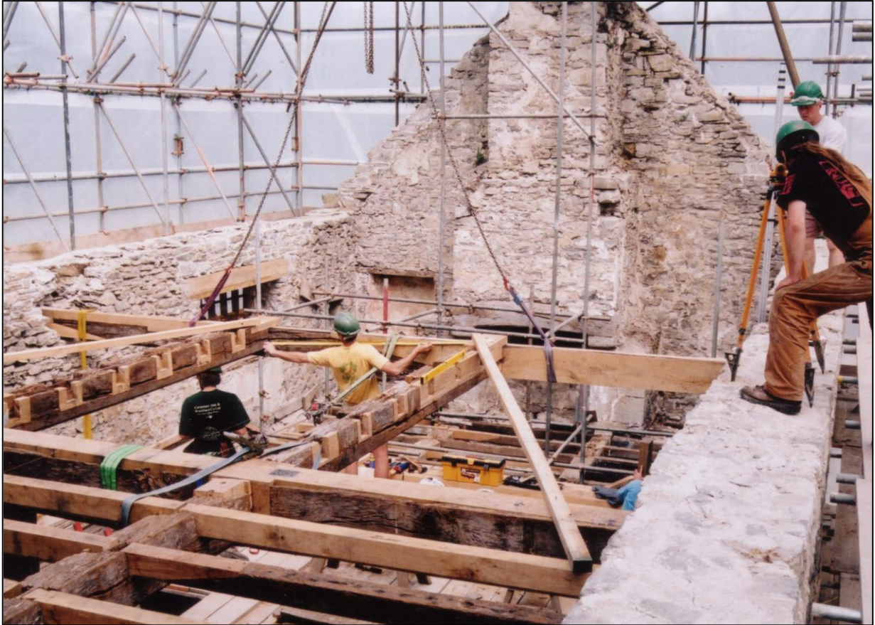
The repaired first floor joists being carefully repositioned above the hall.
