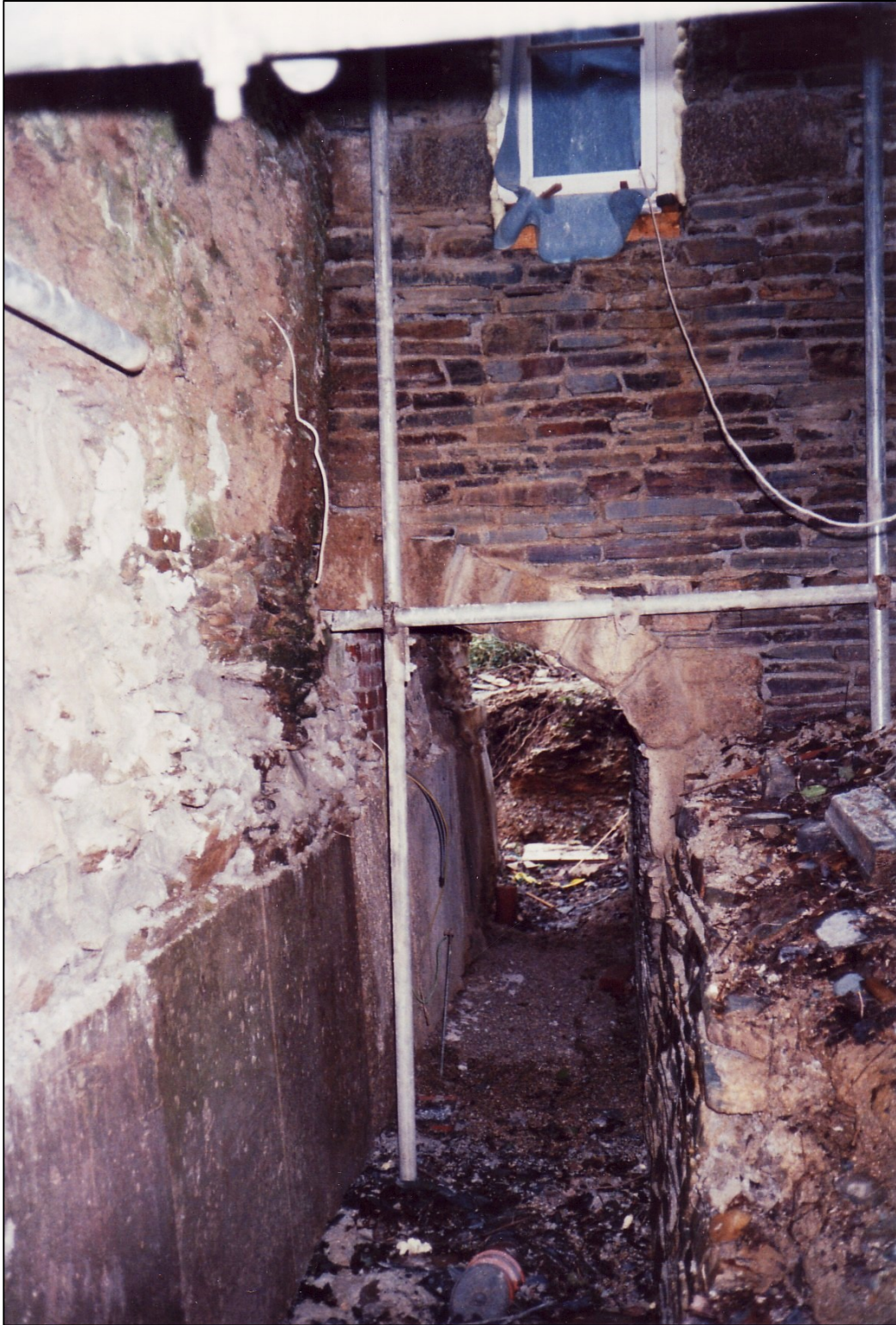
Reinforcing the back wall
