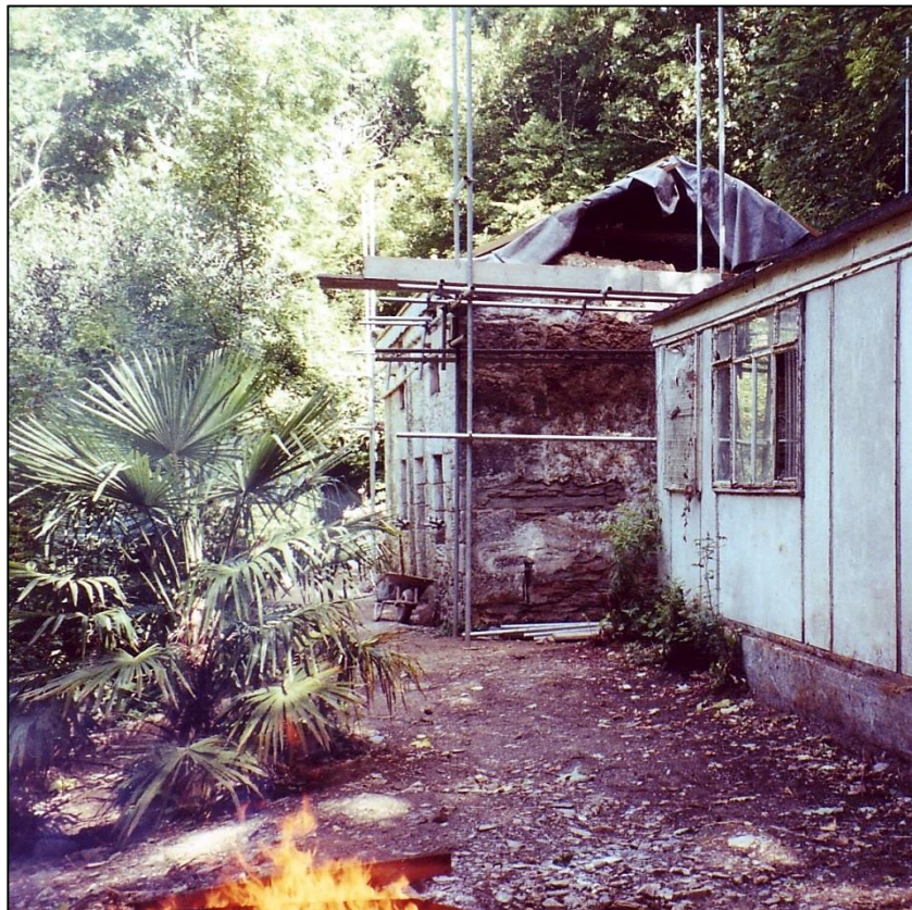
Rebuilding the gable walls
