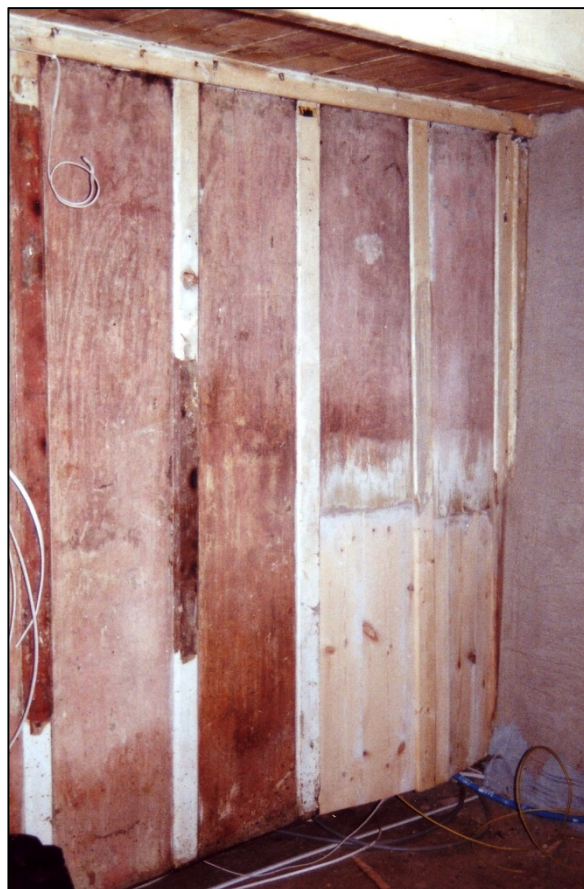
Repairs to the partition on the ground floor
