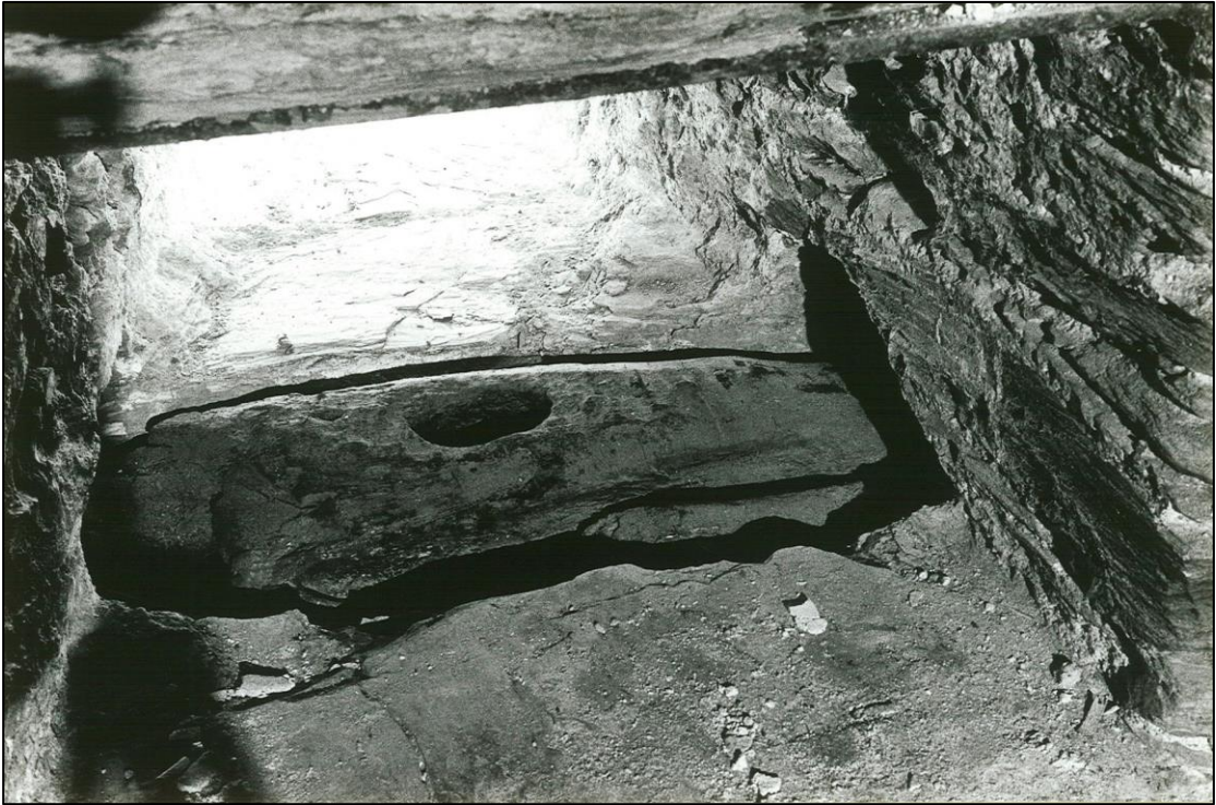
One of the timber plates discovered in the cills of the gun embrasures.
