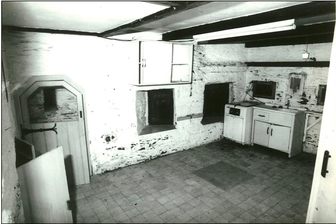
The ground floor – east side
