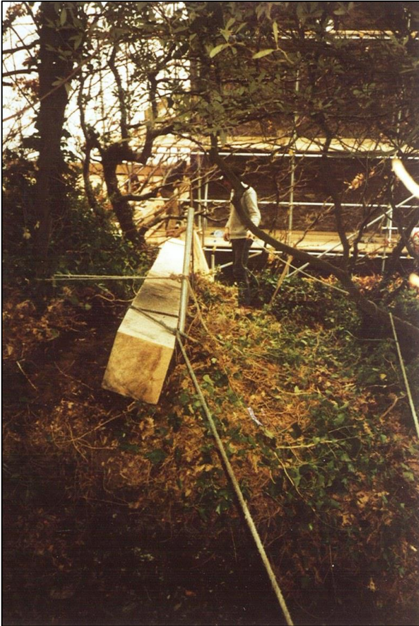
Working the bridging teams for the new first floor.
