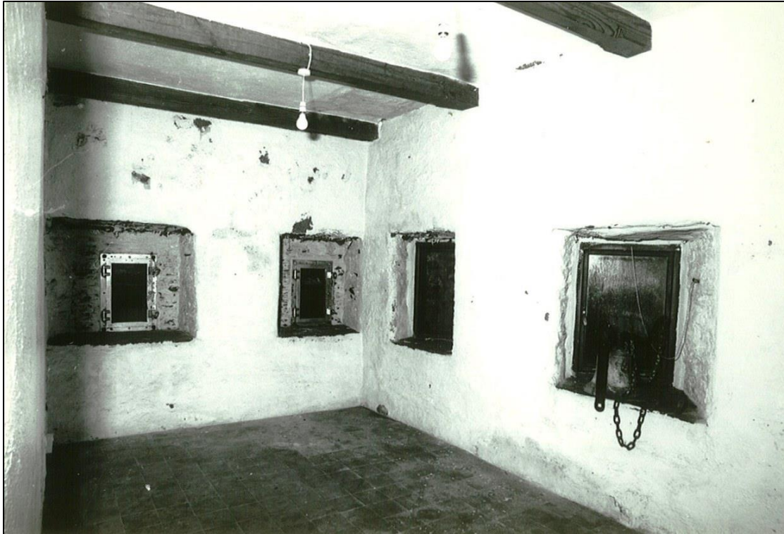
The ground floor – west side
