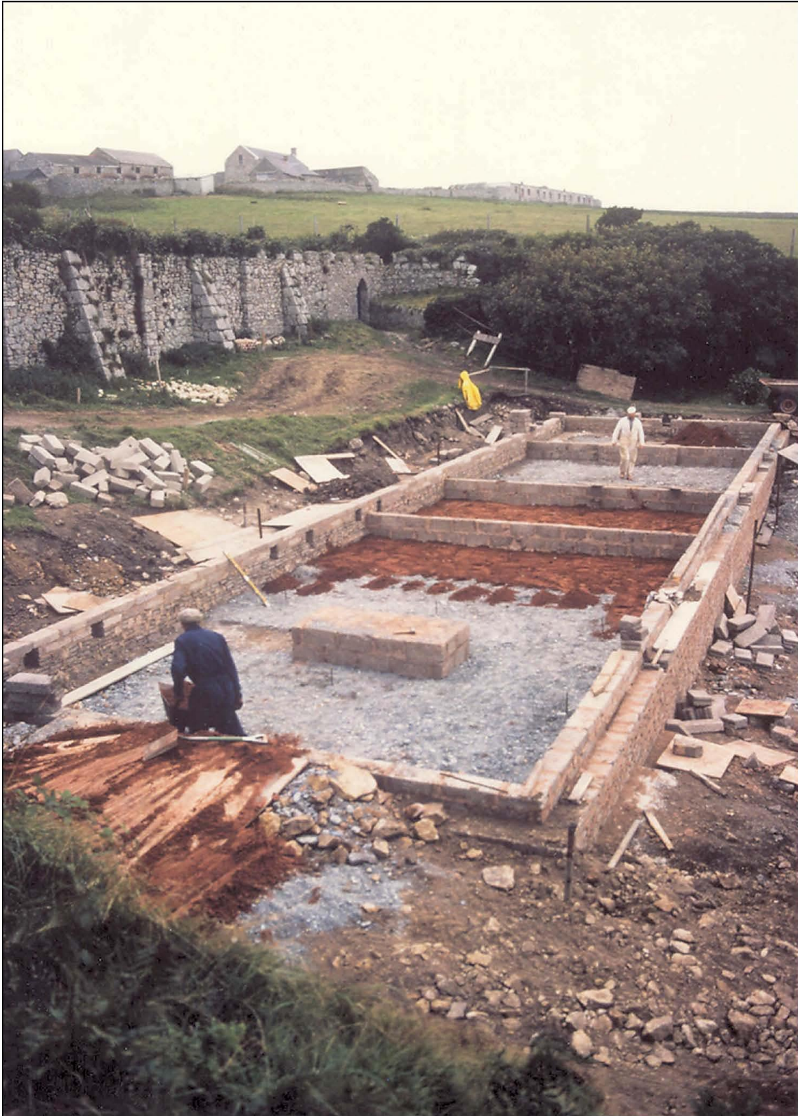
The construction of Government House
