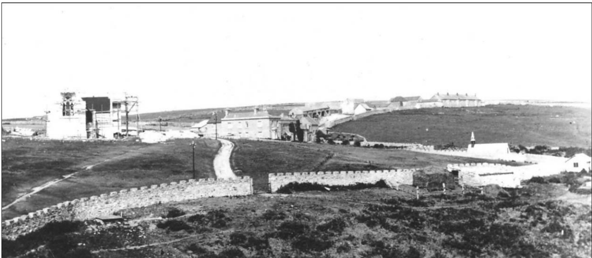
Another view of the Church under construction with the village beyond and to the right. Barton Cottages on the skyline have gabled roofs. The corrugated iron church with its spire, which preceded St Helen's, is below Barton Cottages
