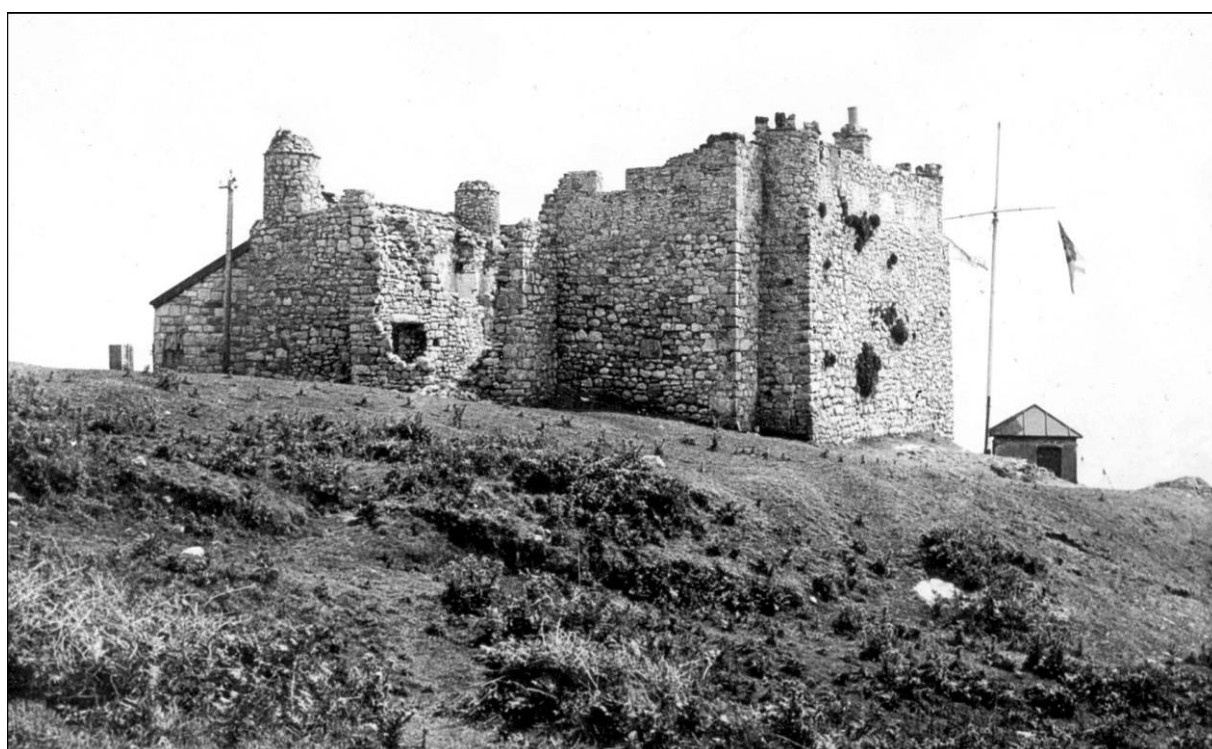
Photo taken in June 1928 which was part of the SPAB report by Charles Winmill
