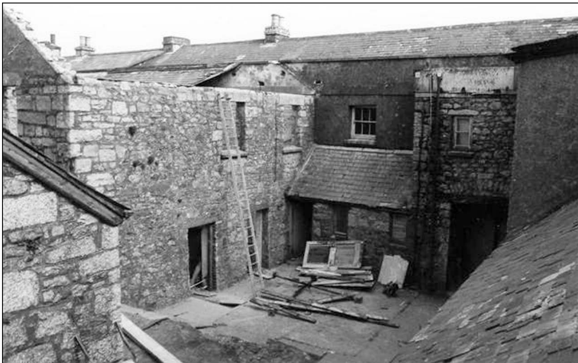
Starting demolition of the hotel outbuildings to create the courtyard. The gable end of the Radio Room is on the left and the sloping roof on the lower right was part of what is now Square Cottage
