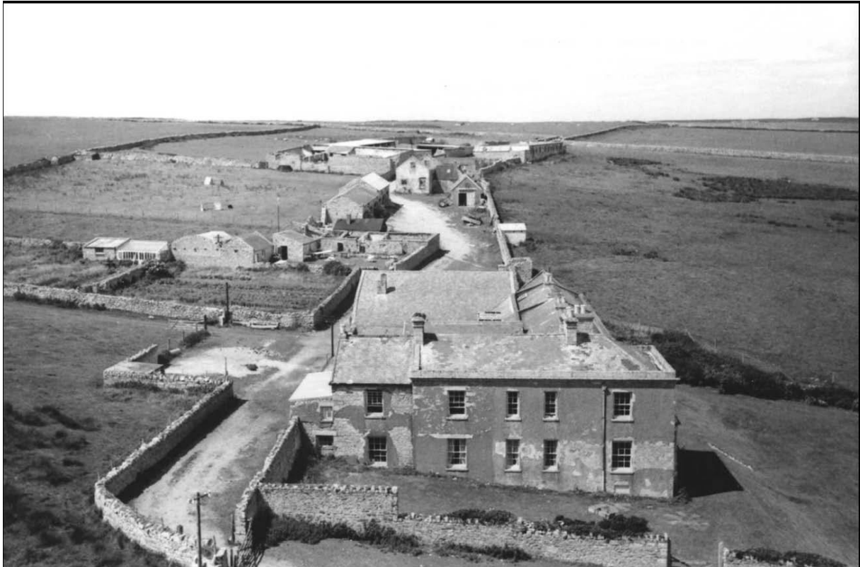
The Big House, now mostly demolished
