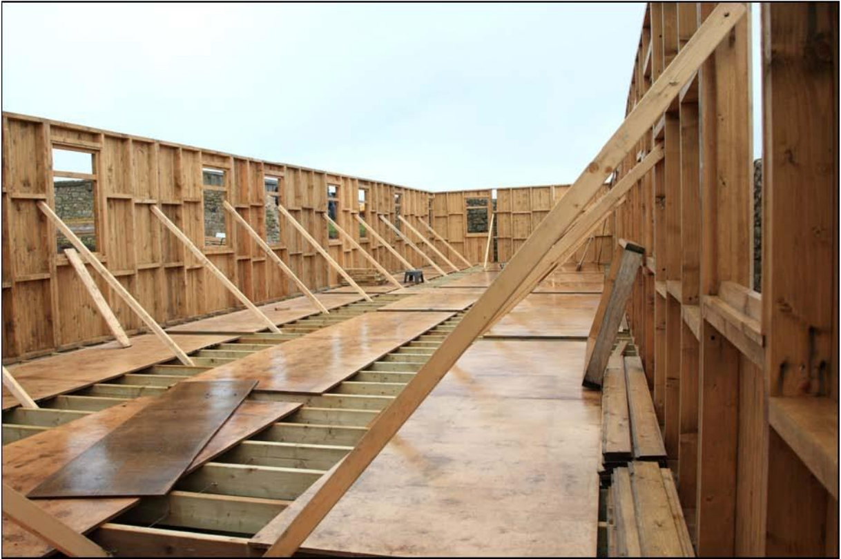
The Lodge under construction
