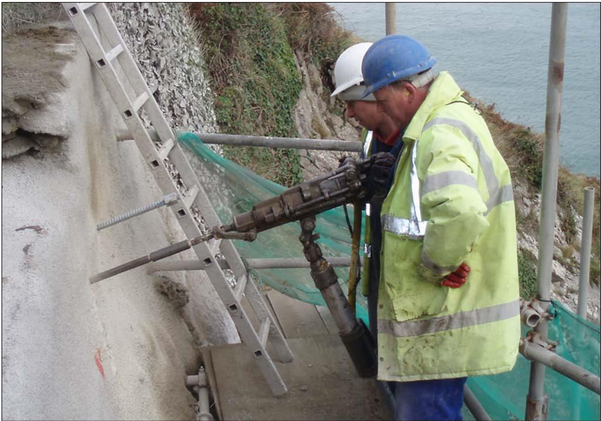
Stabilization work on the Beach Road
