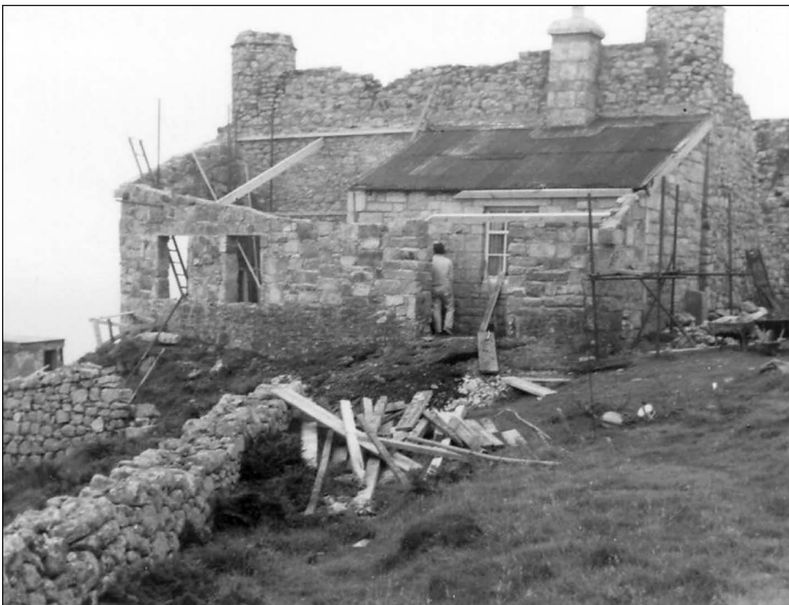
The Cable Hut being extended in the late 1950s
