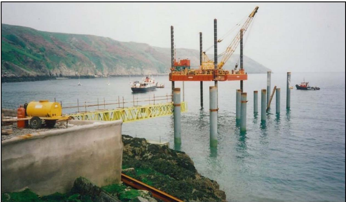
The jetty under construction in May 1999
