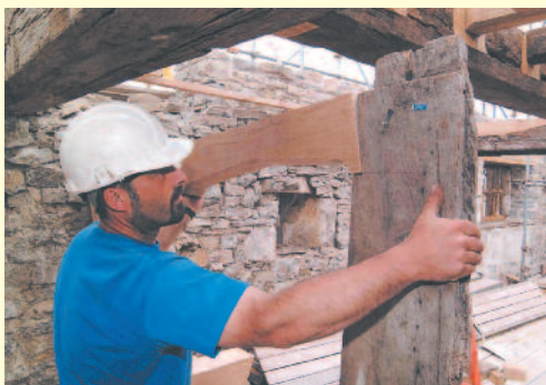
Piecing together Dolbelydr's internal timber frame.
