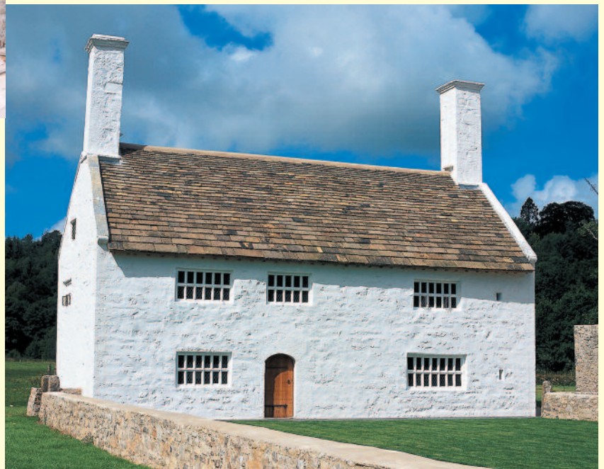
Following major restoration work, Dolbelydr is welcoming successive visitors and now has a sustainable future.
