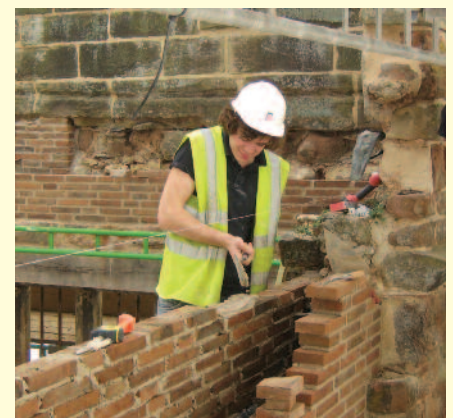
An apprentice laying brickwork at Astley Castle.
