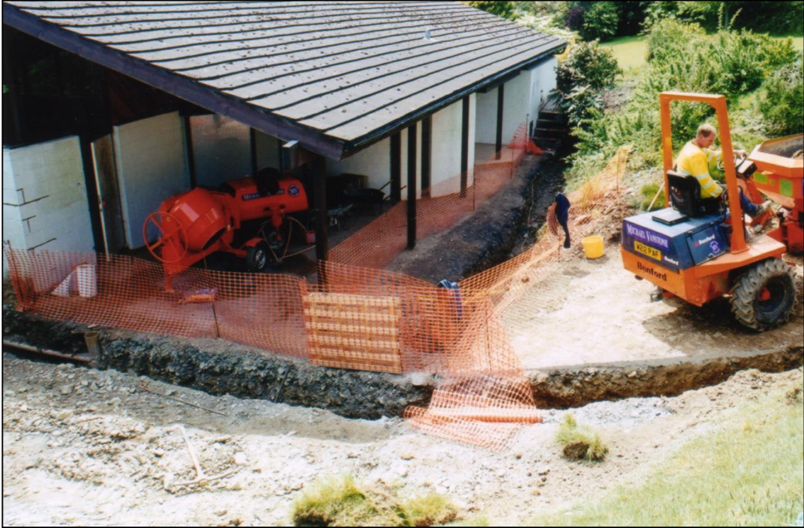
Installing improved drainage. The grid now to be seen in the middle of the lawn is a last resort overflow in case even the new soakaways prove inadequate.
