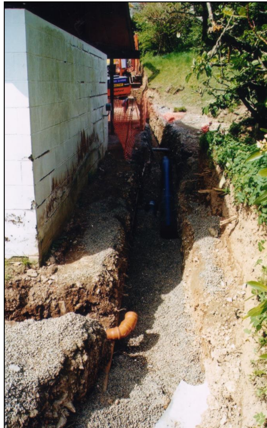
Installing improved drainage. The grid now to be seen in the middle of the lawn is a last resort overflow in case even the new soakaways prove inadequate.
