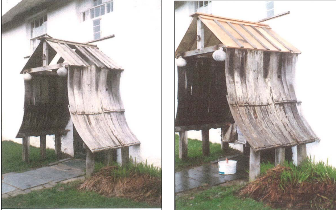
Canopy at no 1 Hawker's before and after 2004
