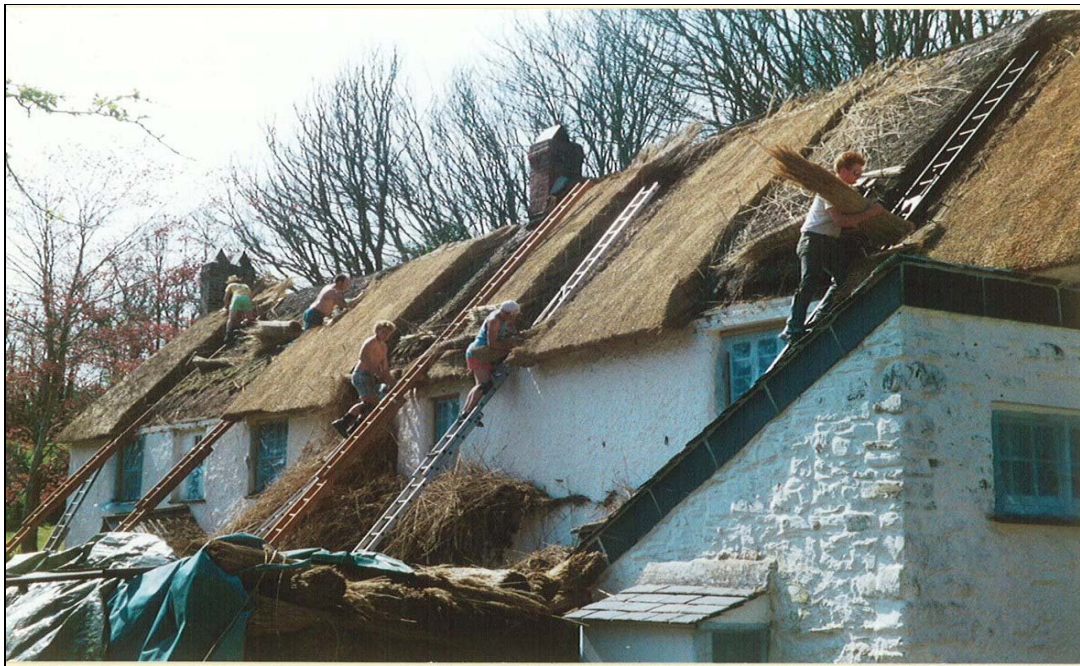
Re-thatching at Hawker's cottage
