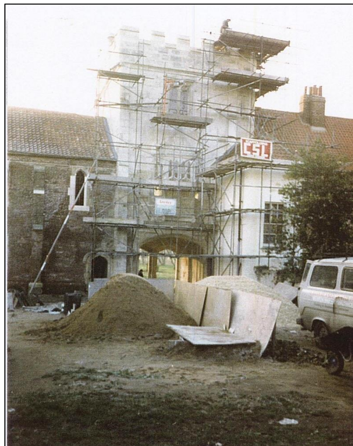
The parapet completed: work in progress on the spiral staircase turret
