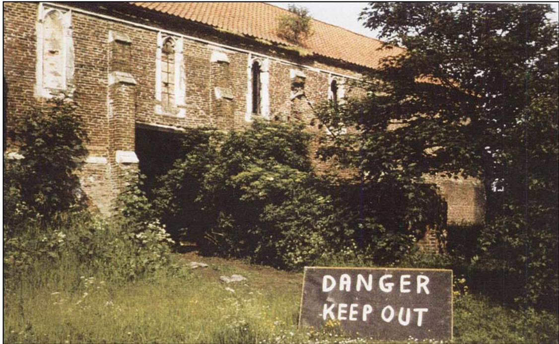
The south side in 1985, showing the barn door, the bricked-up windows and the buttress hacked away for a farm shed
