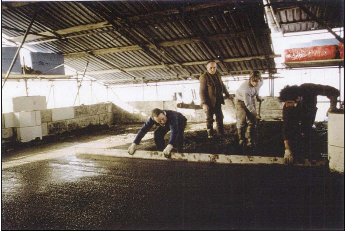
Concreting the Gatehouse roof
