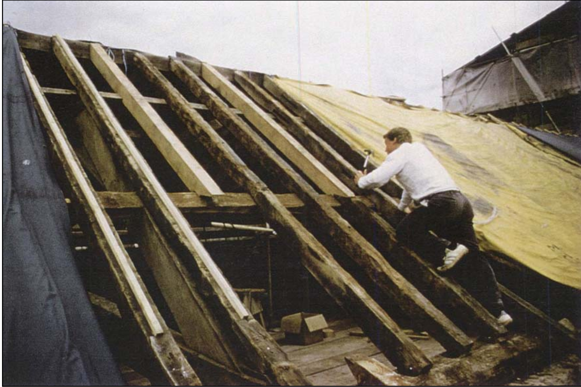
Repairing the roof and rafters of the east range
