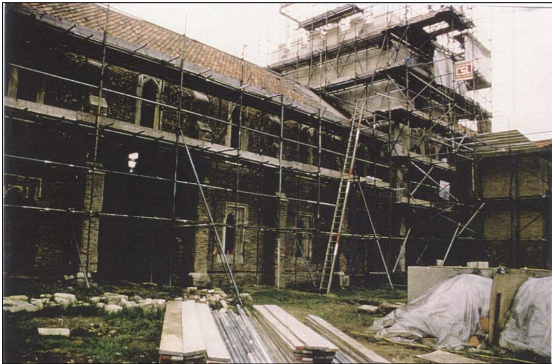
Work in progress on the north side
