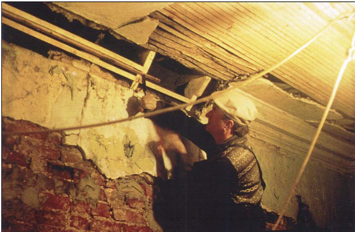
Running the plaster cornice in the Georgian staircase
