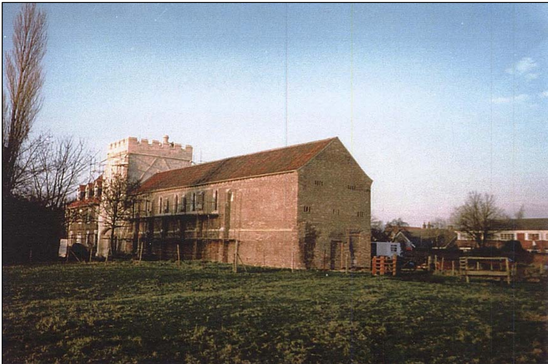
The south and east sides of the east range after restoration but before reducing the ground level
