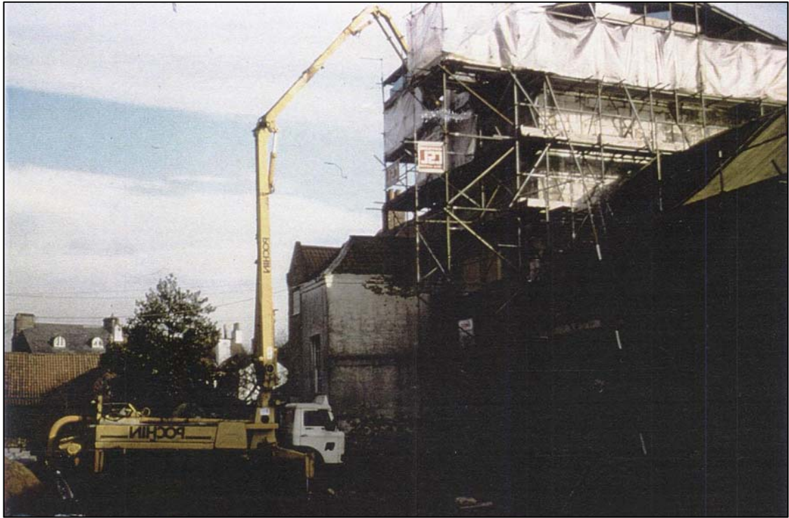
Hoisting up the parapet stones
