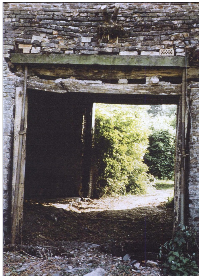
The barn door from the north side in 1985
