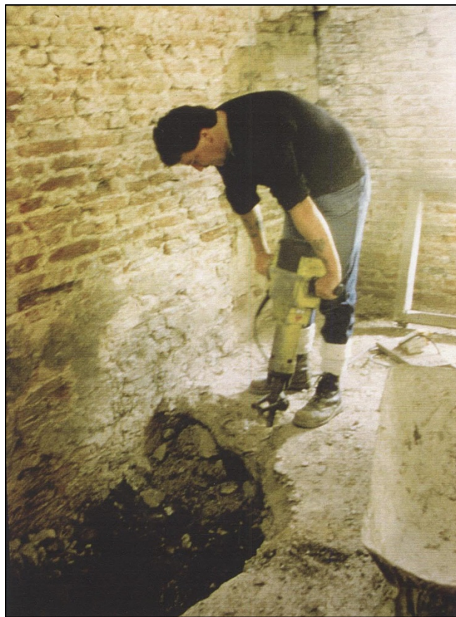
Investigating the floor in the east range
