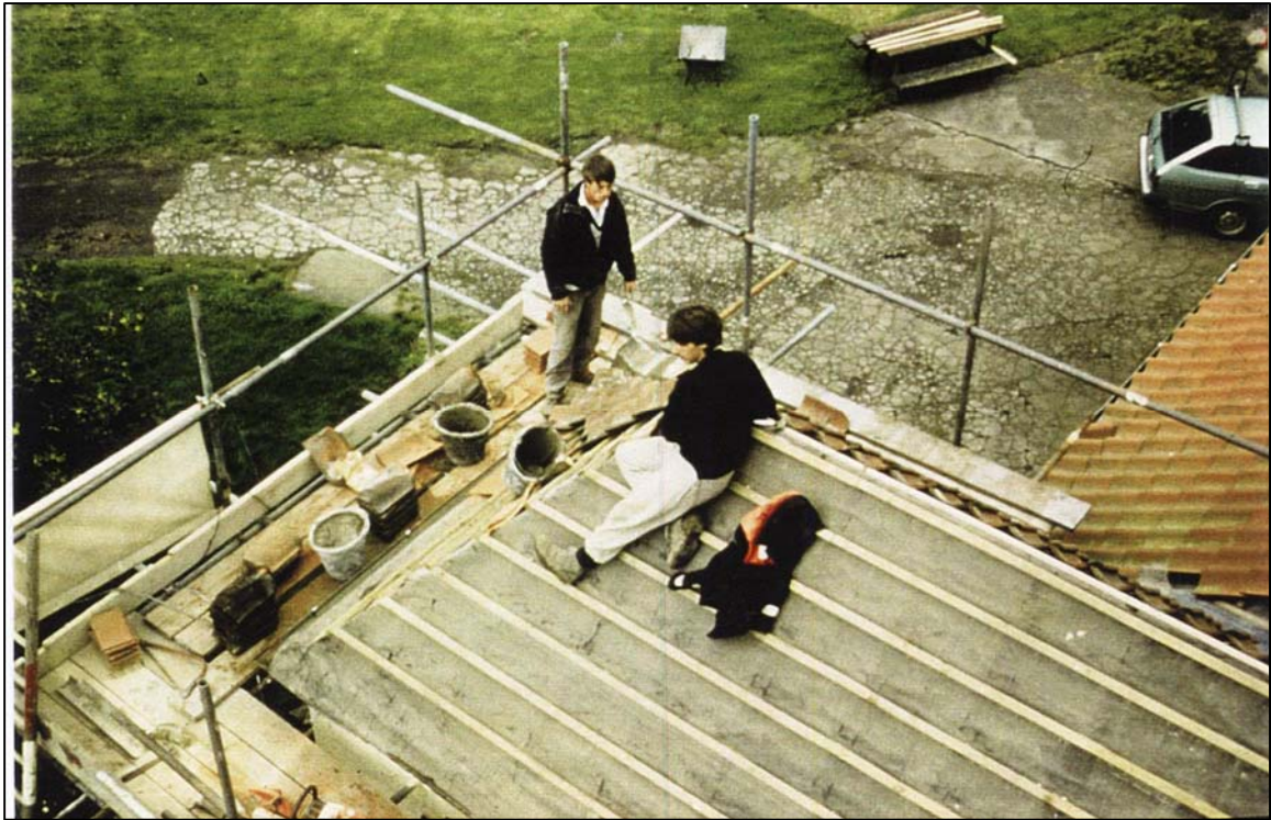
Reroofing the Georgian staircase
