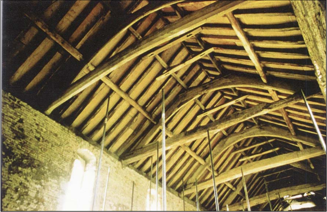
The roof restored
