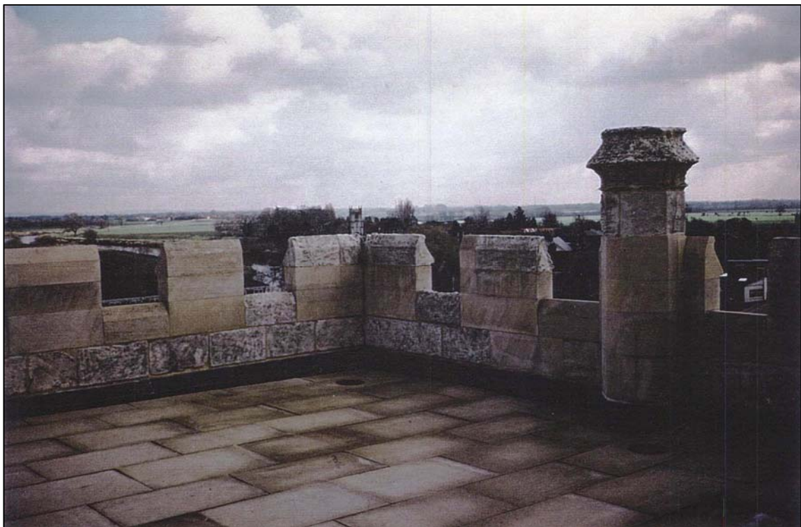
The restored roof, parapet and chimney
