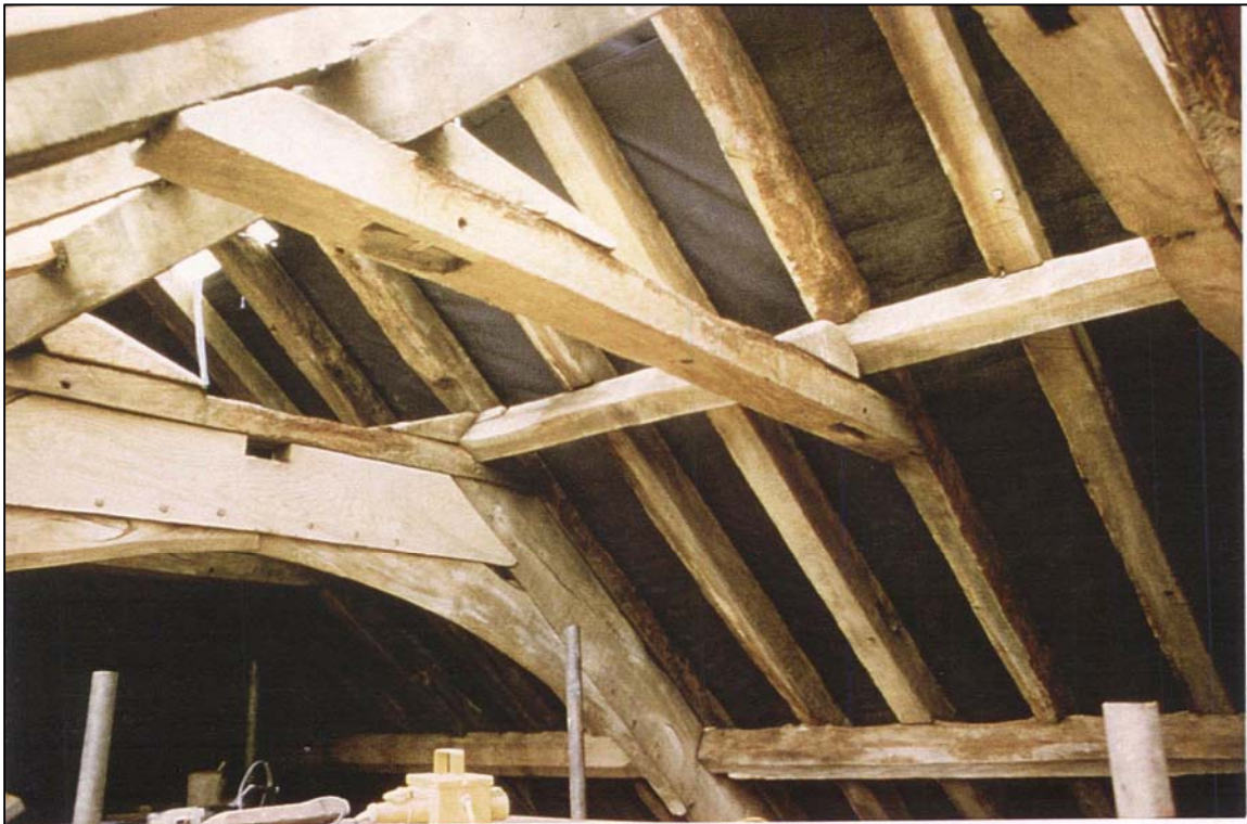
The restored roof: rafters, collars and braces
