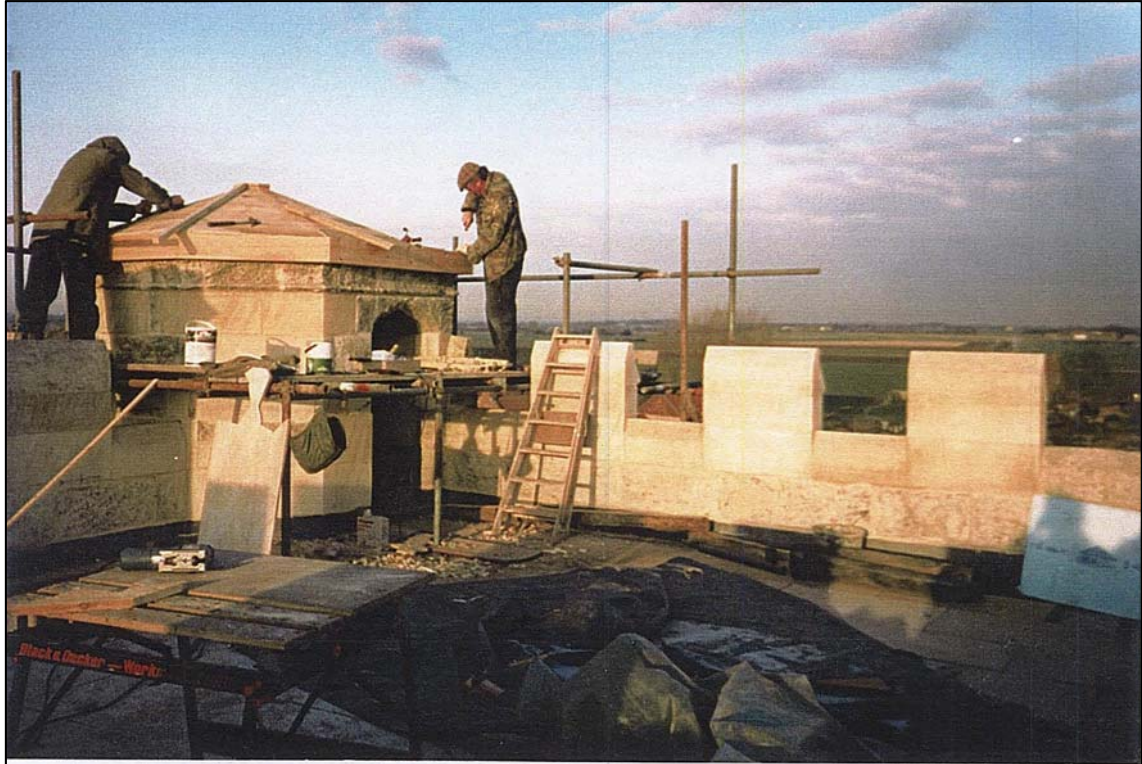
Construction of the spiral staircase turret
