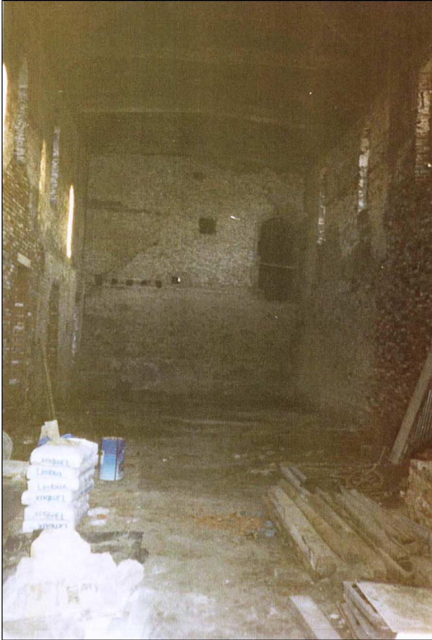
Looking east at the later cross wall with rebuilt first-floor doorway
