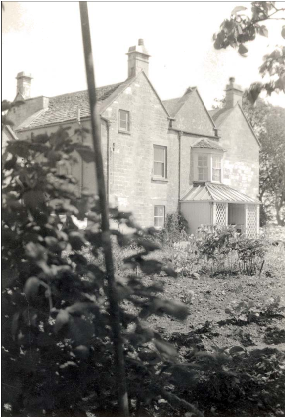
The west side of Field House in about 1970.
