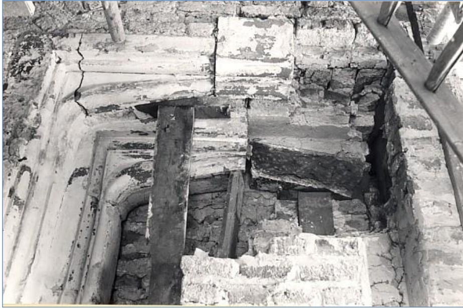
The first floor doorway when newly discovered behind plaster.
