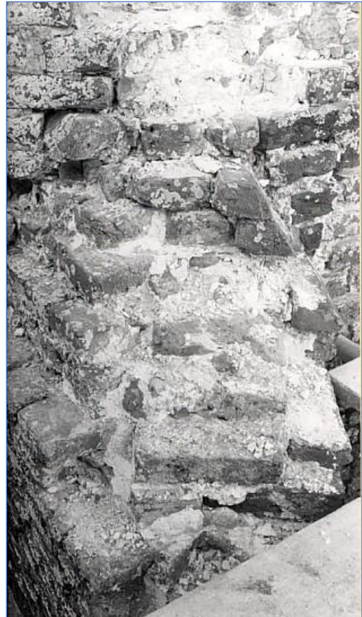
Remains of a crenellated parapet, beside the stair turret.
