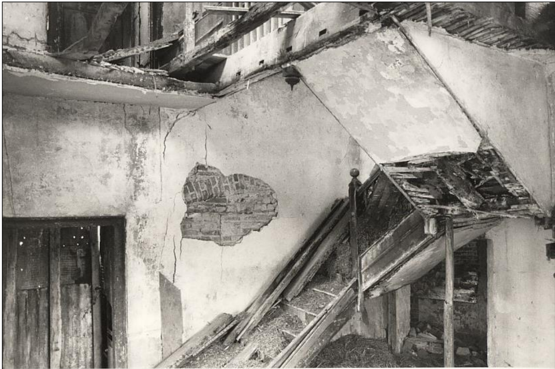
The Ground Floor. The decayed Georgian stair, blocking the door to the stair turret. The head of the Tudor window can be seen behind the plaster. The door on the left led into the dining room of the Georgian Gothick house.
