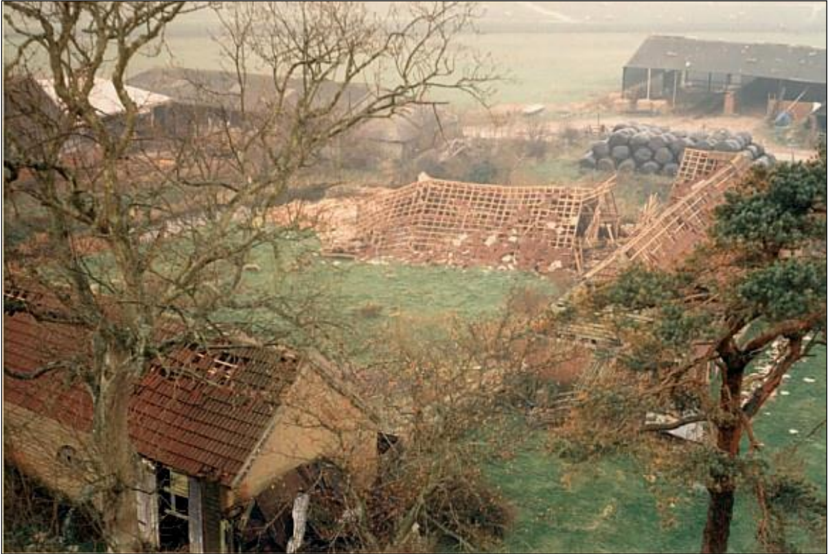
Buildings inside the southern corner of the moat after the gales in October 1987.
