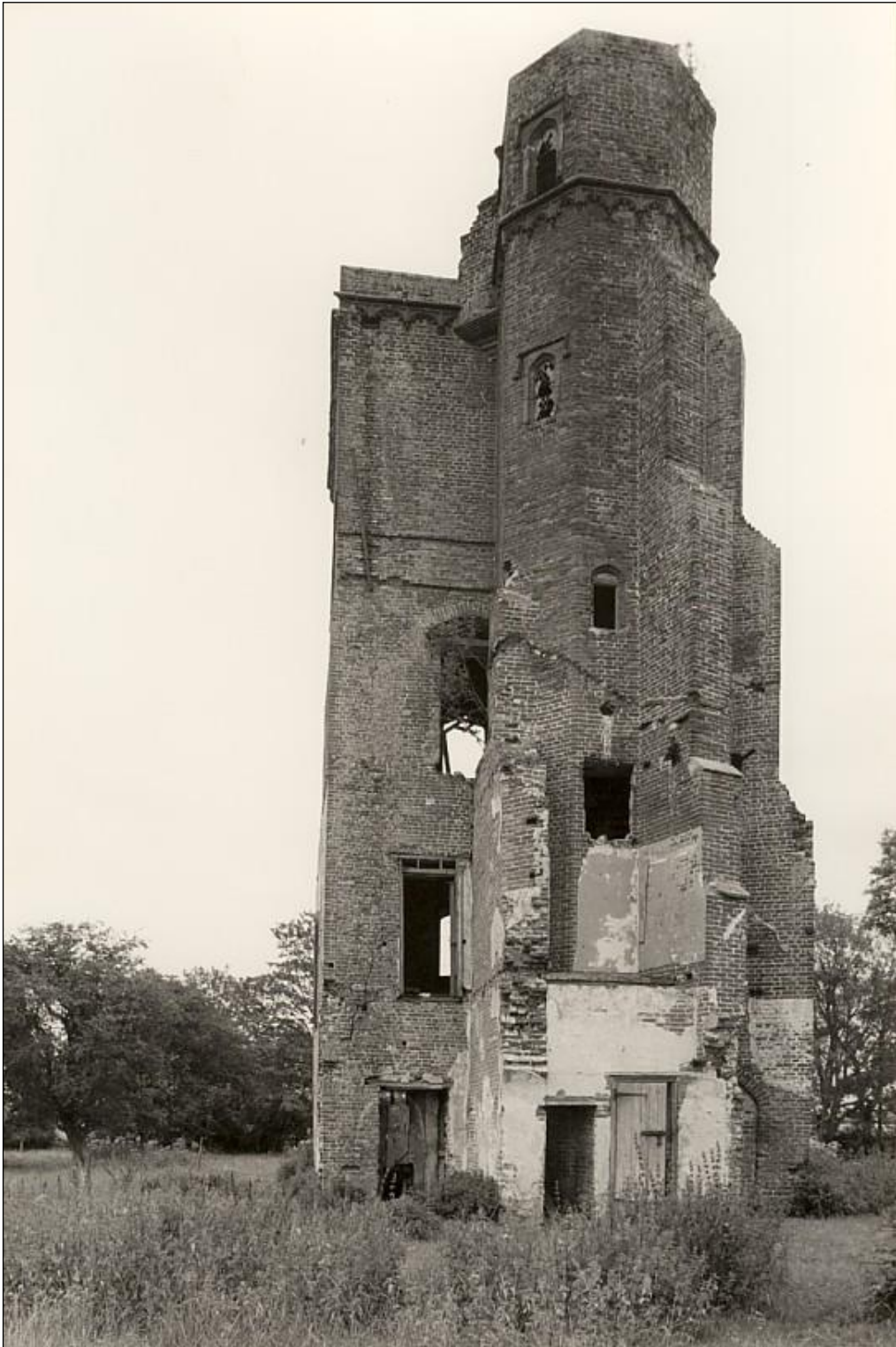
The North West Face. The remains of the 18th-century additions can be seen against the stair turret.
