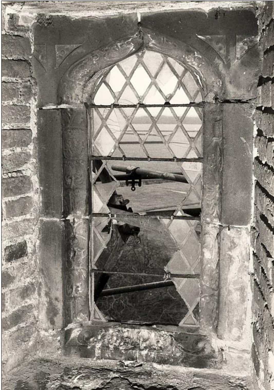
A Stair Turret Window
