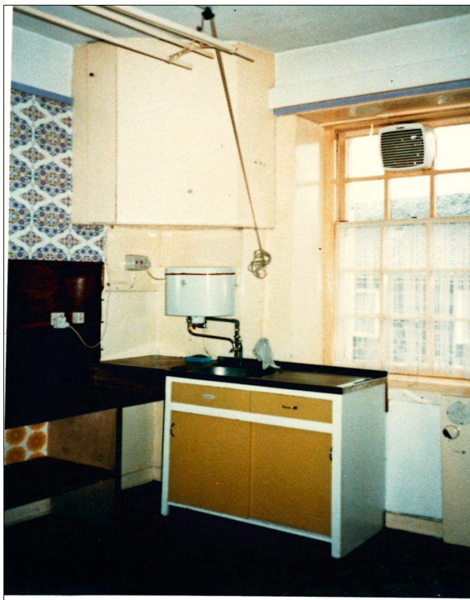
In the kitchen, some original wallpaper and distemper was uncovered in the kitchen.
