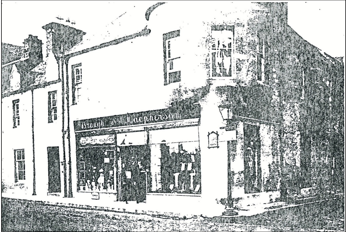
(1.3(a)) Early photograph of building (above). (1.3(b)) General view from across the river Earn (below).
