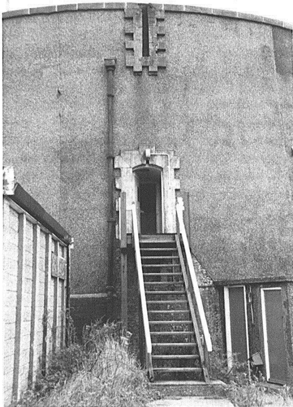
3. Tower P, Felixstowe, Suffolk, entrance. (Charles Blackwood)
