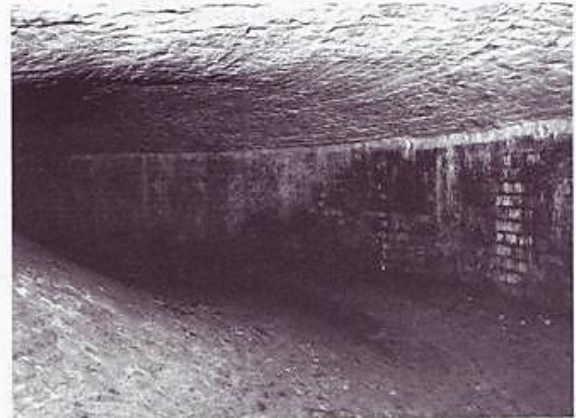
Empty water tank in base of Martello Tower 73. Base of rising central pillar at left (Andrew Goodwin)
