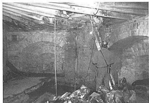
4. Tower U, Felixstowe Ferry, interior. (Charles Blackwood)
