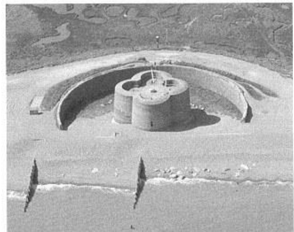
12. An aerial photograph of the unique quatrefoil Tower CC, Aldeburgh, Suffolk. (Damian Grady © English Heritage NMR: 23496/15 23 Apr 2004)
