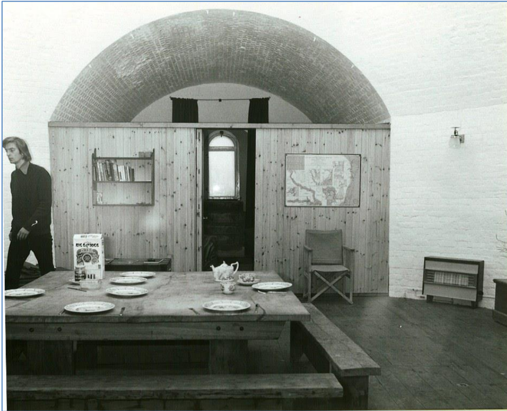
1975. The original restoration had used "knotty pine".
