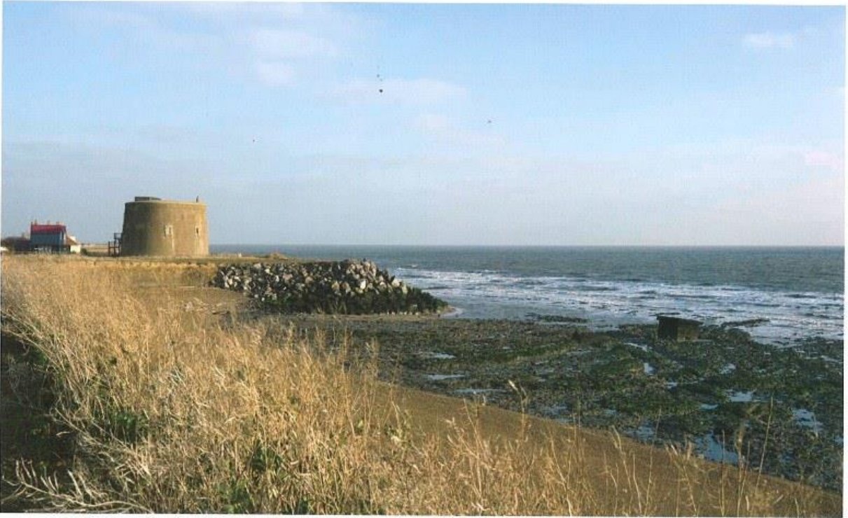
Martello Tower W, Bawdsey, Suffolk, showing the level of coastal erosion in this area. (Steve Cole © English Heritage NMR: DP046351)
