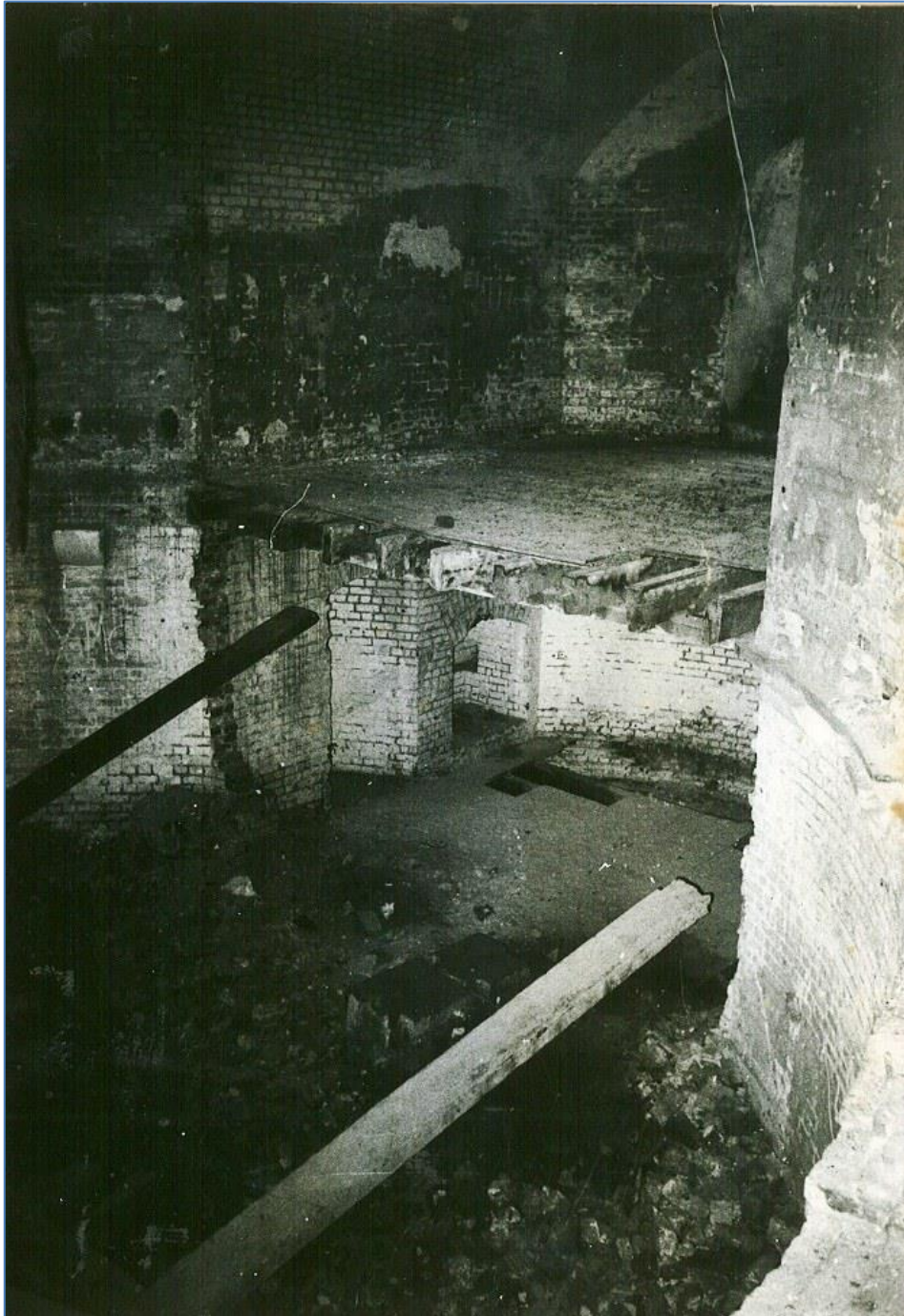
Looking down into the basement
