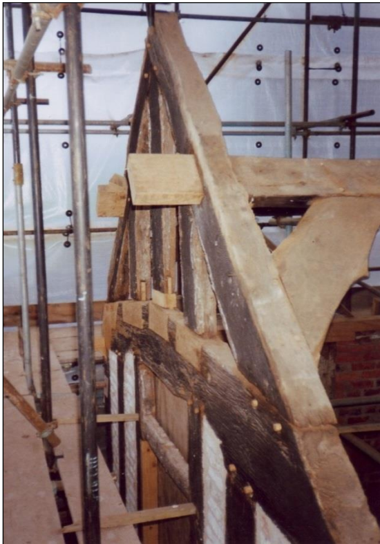
Detail of eaves, notched to fit the slate and prevent rain driving in, making it unnecessary to fit a fascia board.
