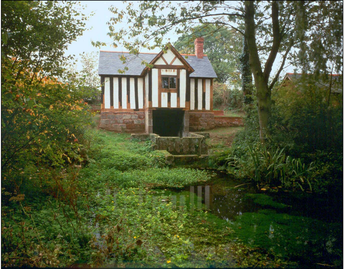
St Winifred's Well, restoration newly complete, in 1991.
