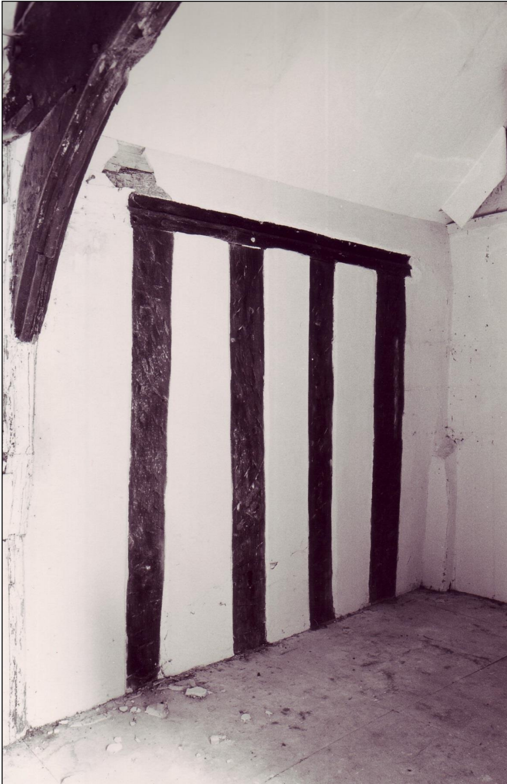
Some sections of the timber-framing were visible inside the building.
