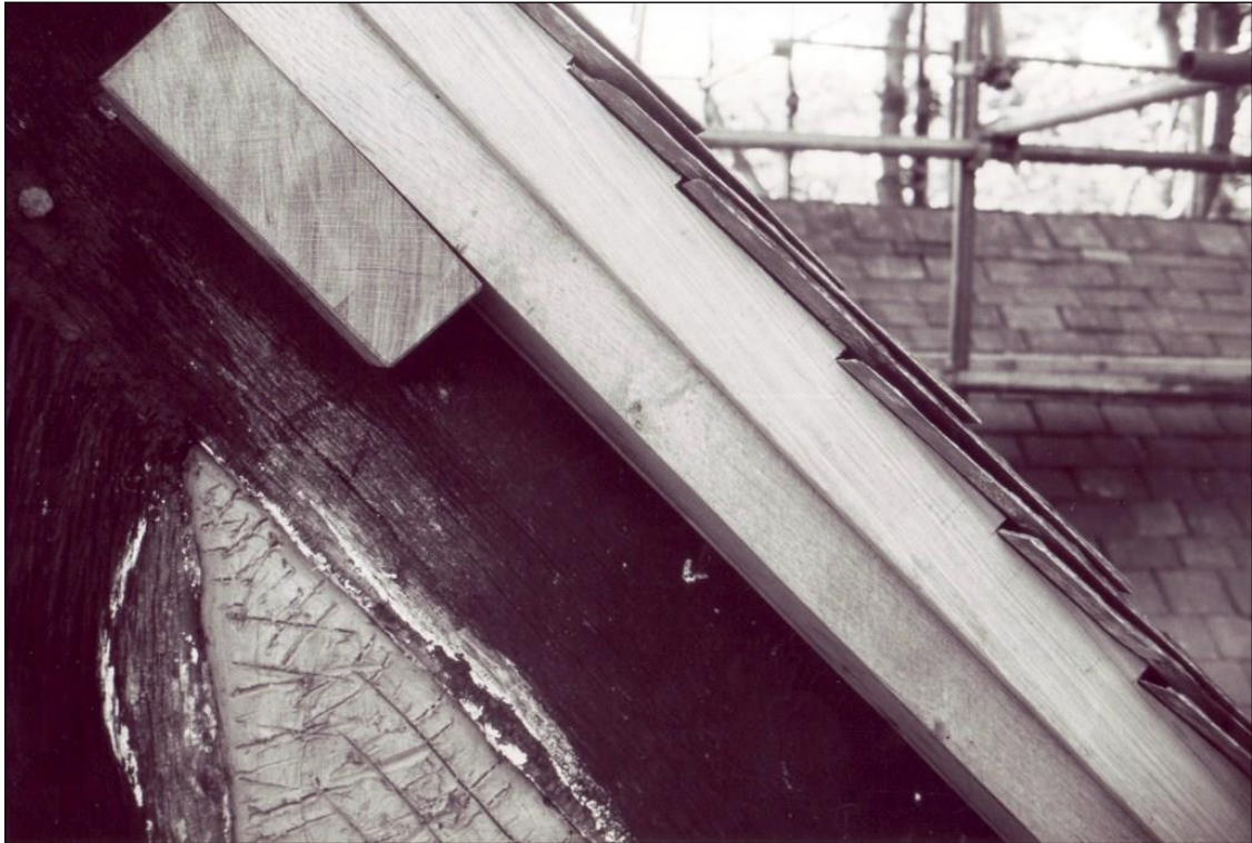
Detail of eaves, notched to fit the slate and prevent rain driving in, making it unnecessary to fit a fascia board.
