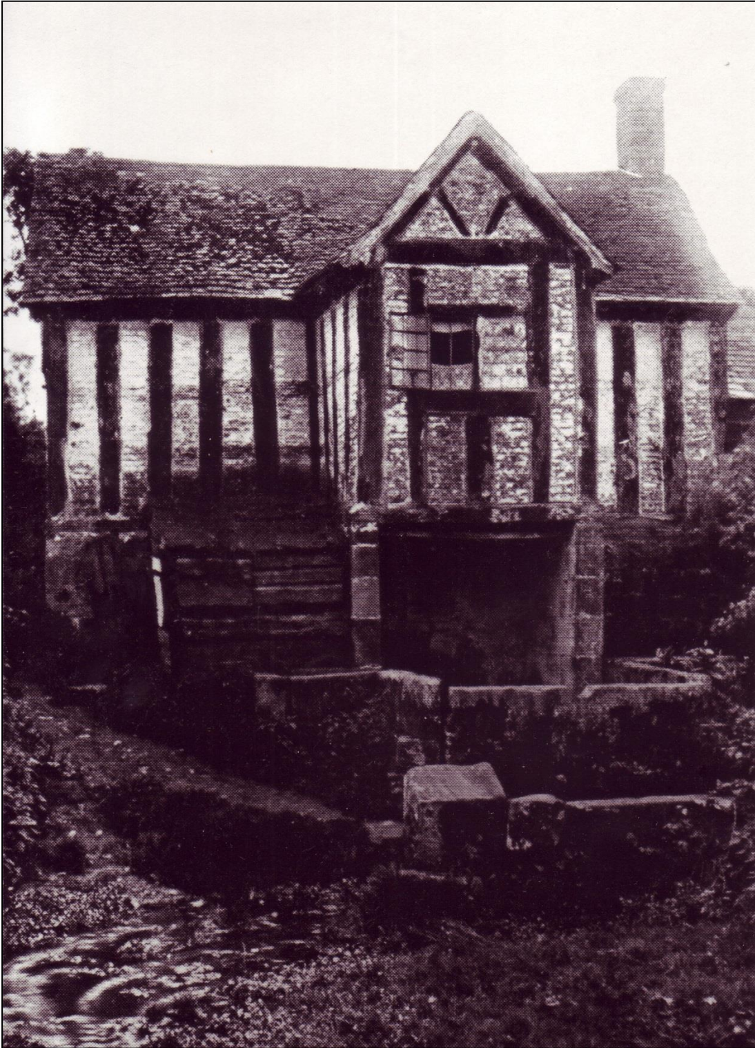
A photograph taken before 1930, when the old roof of small stone slates was renewed. This provided a clue for the original roof pitch, over which a replacement had been rather crudely placed by the time Landmark took on the building. Landmark's repairs reinstated this original pitch.
