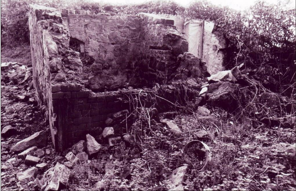
The pigsty before restoration – today the bathroom.
