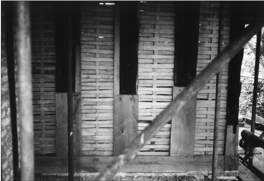
Split lathes awaiting plaster in the projecting wing.
