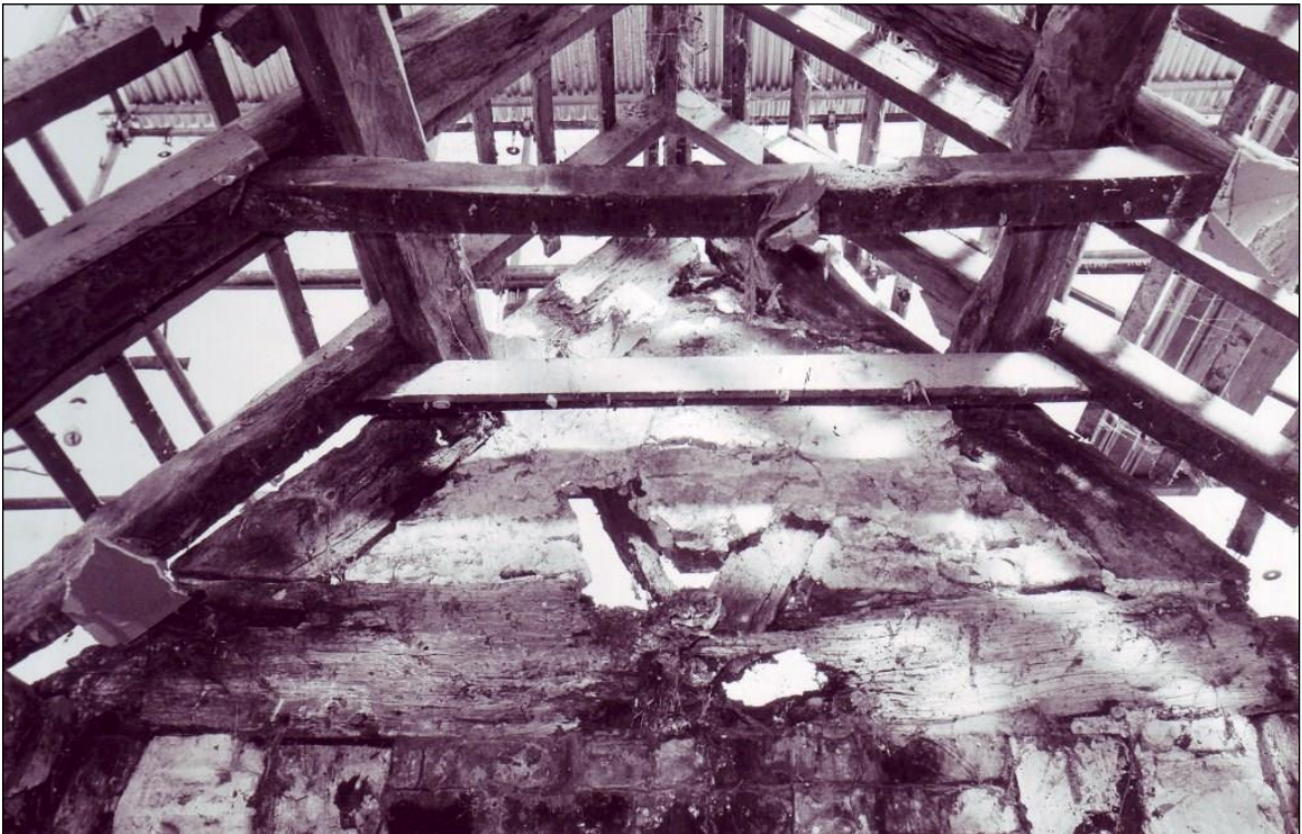
When the roof was renewed c.1930, battens were laid over old joists to provide a more level surface.
