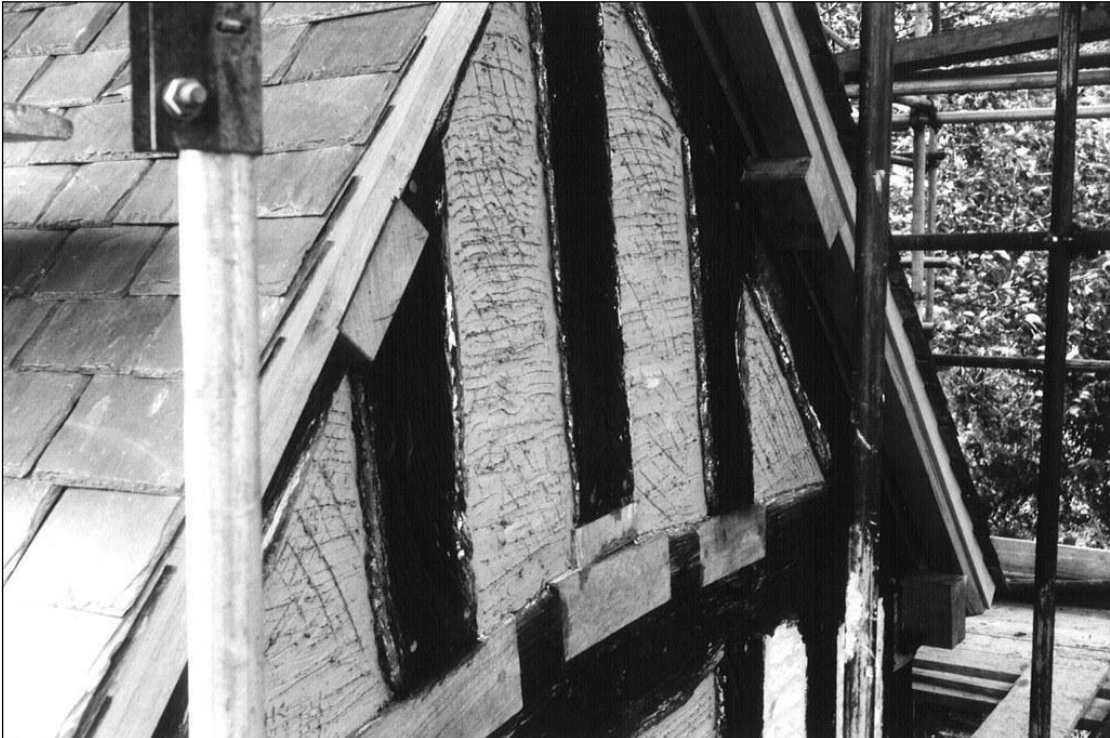
Scratch coat of hair plaster, or daub, on the west gable.
