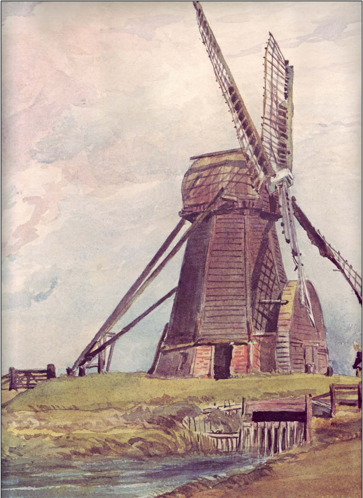
A typical fen windmill, of the kind erected at Mere Mill on the Waterbeach Level, and whose salvaged bricks would be used in the building of the 1841 toll house, later known as Stoker's Cottage.
