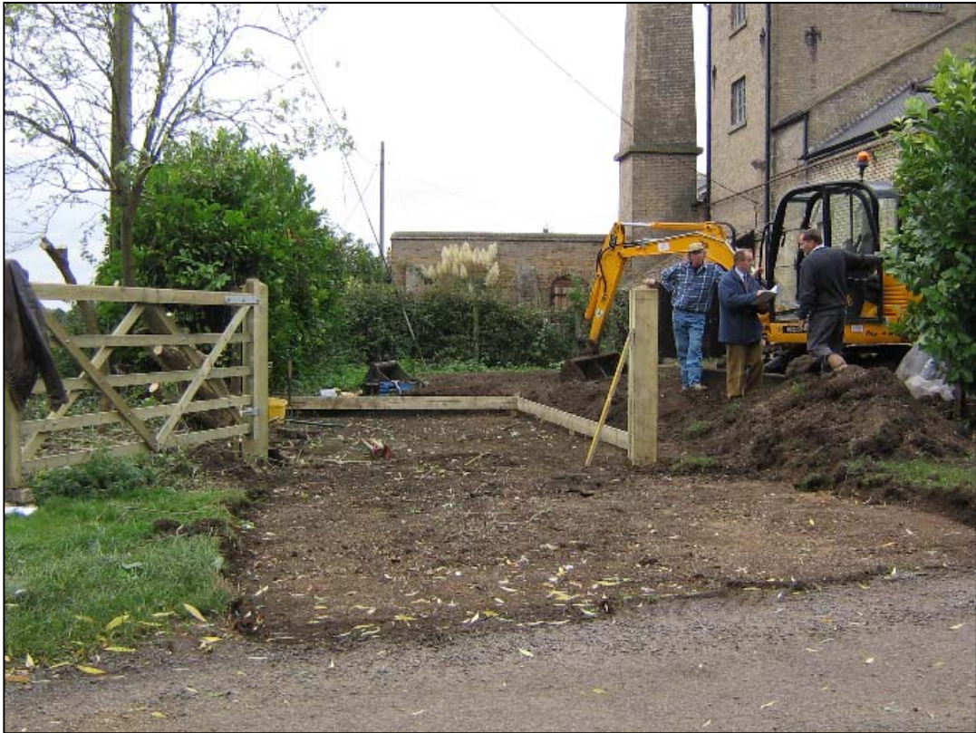
Creating the parking space, after the demolition of corrugated iron garages.
