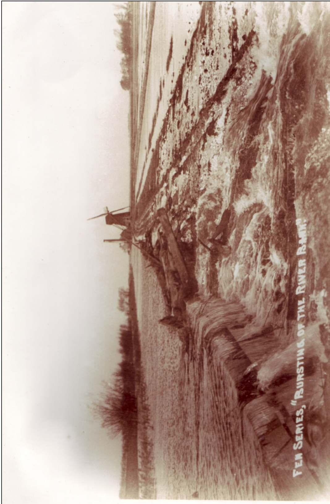
The river bursts its banks: Lakenheath, c. 1900. What happens if the pumping stations fail to cope. Wind pump and 40 hp beam engine and scoop wheel erected in 1844.
