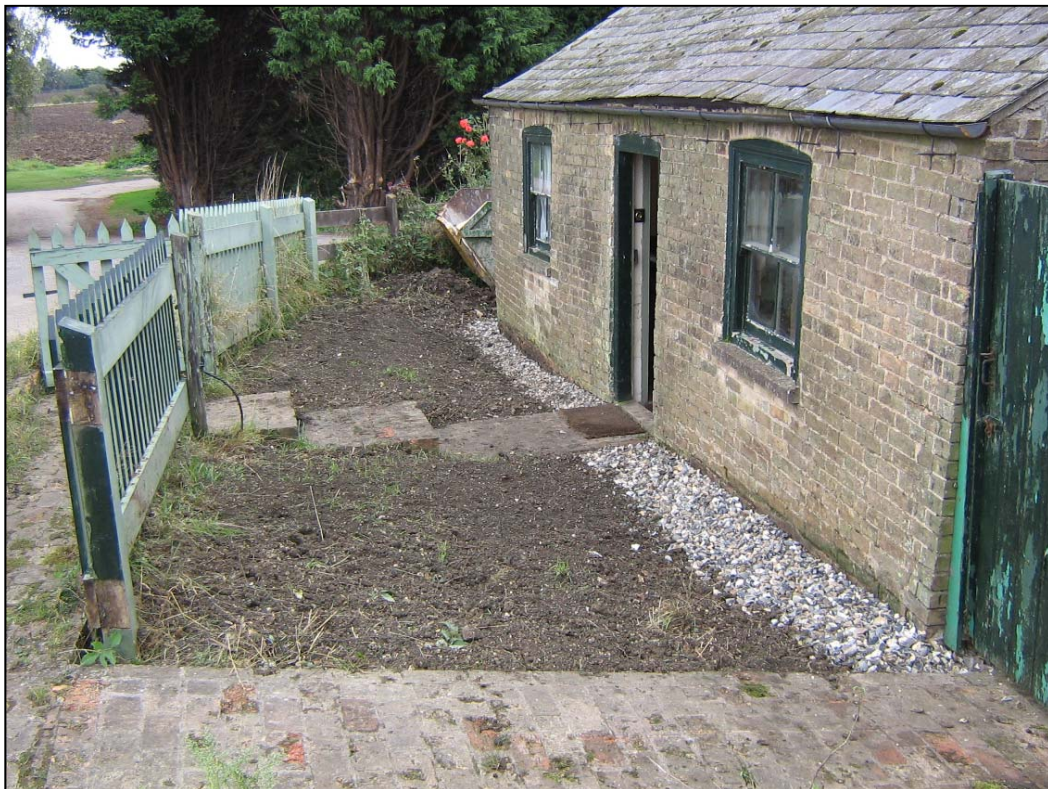
Newly laid French drains, before the front lawn was laid.
