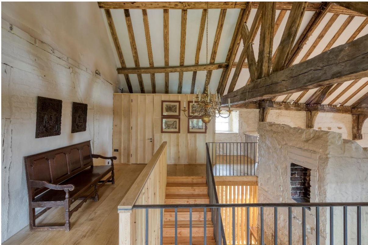
Image 14: The staircase hall at the upper level, looking over the staircase towards the lift
