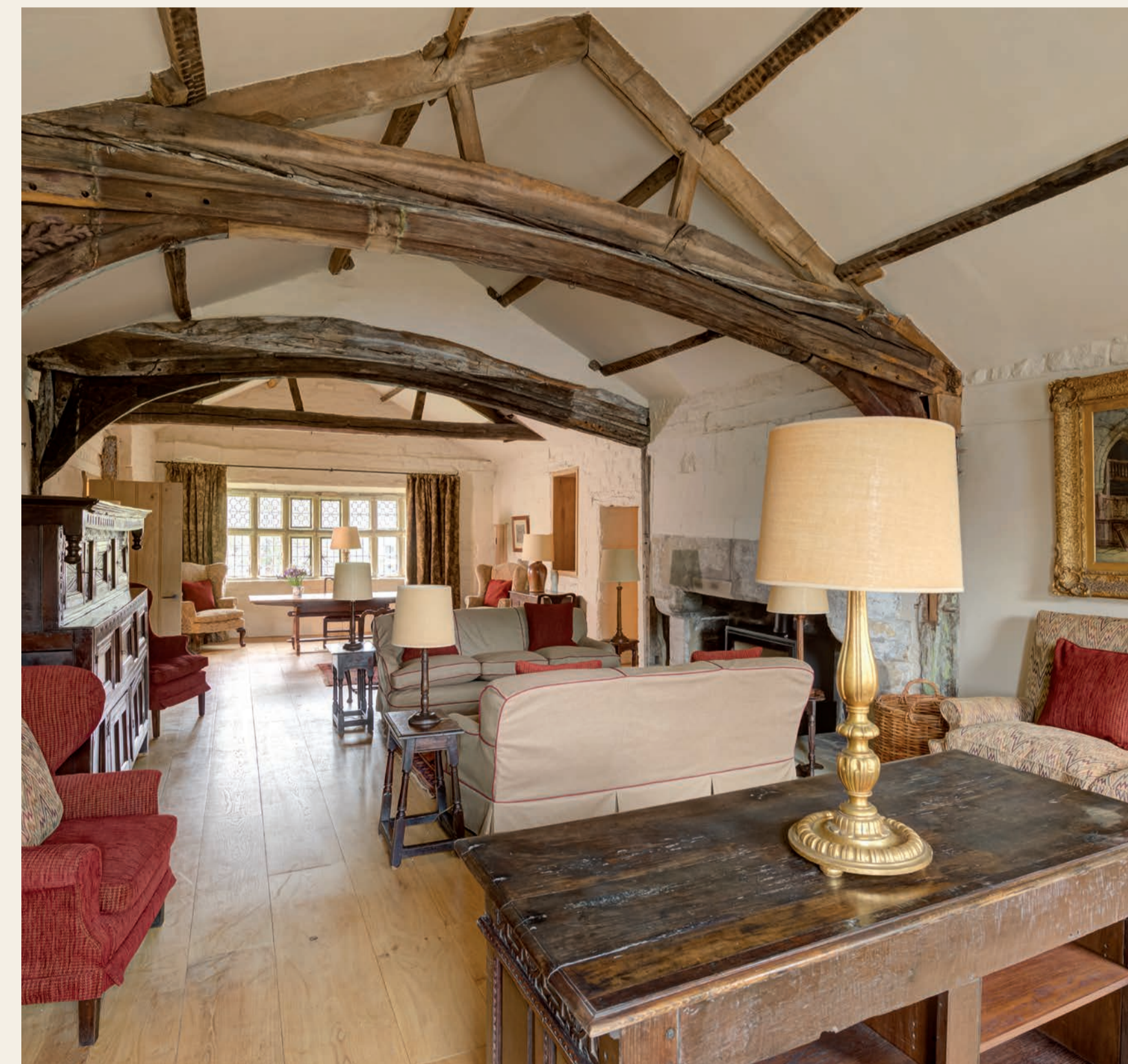
The upper floor of the Solar Block, after repair and conversion.
