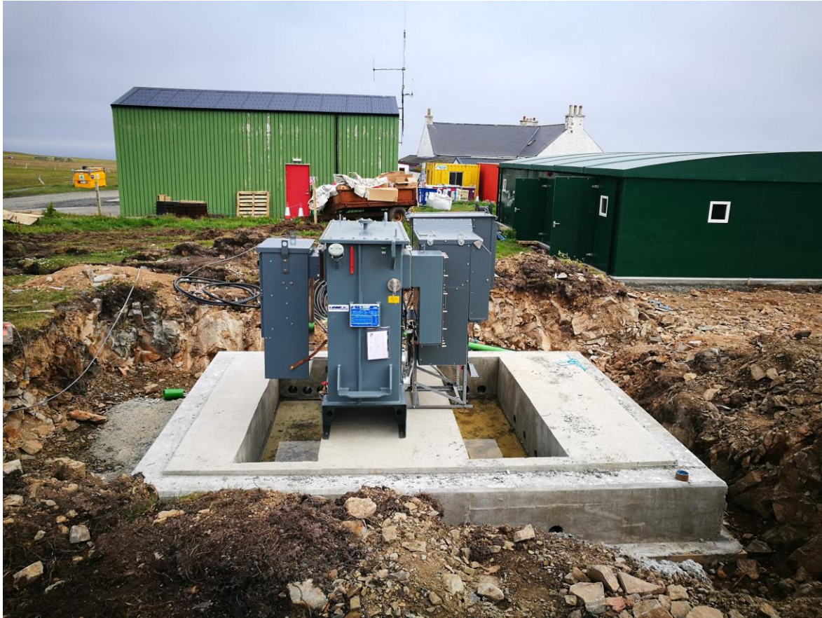
Transformer and batteries being installed
