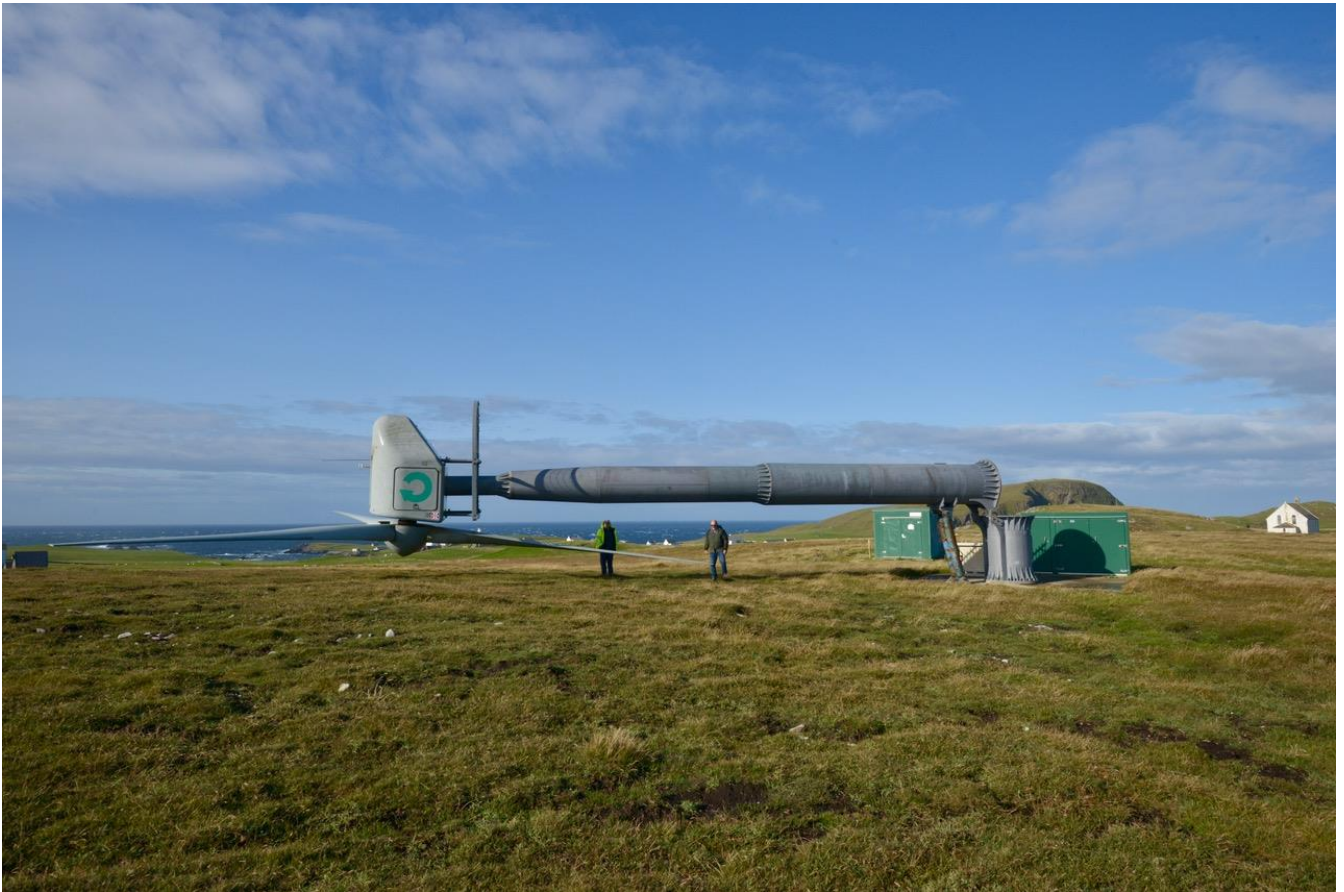
No 2 Turbine on the ground on the hydraulic ram
