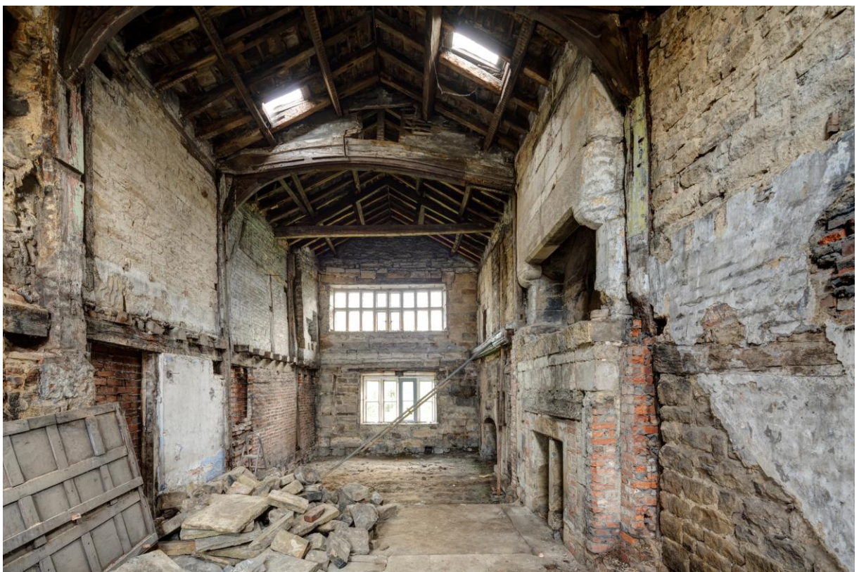
The Great Hall (top) and gutted first-floor hall/Solar Block in 2020.
