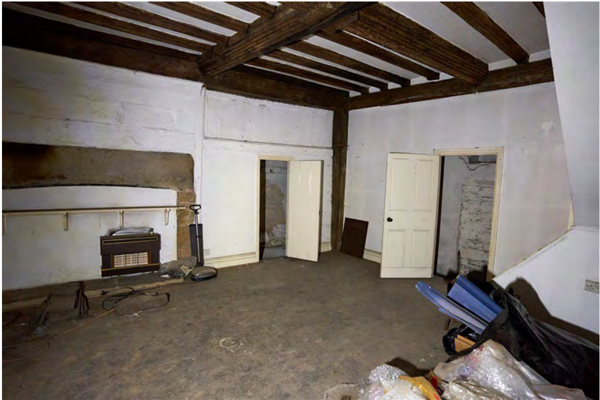
Top: the ground floor of the Parlour Block in 2020. The slope of an inserted cottage staircase is in the foreground. The blocked doorway to the Solar Block was a cupboard.
