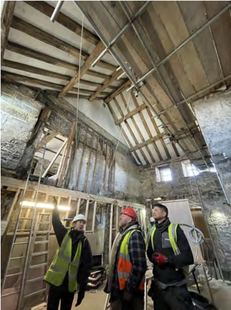
During the clearance of the cross passage, the original doorway into the first-floor hall was discovered in 1320s framing. Here, architect Karen Lim briefs Kevin Woods, plasterer (in the red hat) Michael Bloom, joiner
