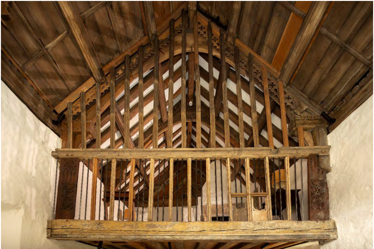
The chapel gallery seen from below, 2024.
