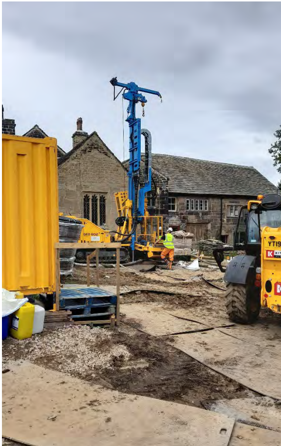
Drilling the bore holes for ground source heating. Six bore holes were drilled to a depth of 143 metres. The process proved easier than anticipated, to everyone's relief.
