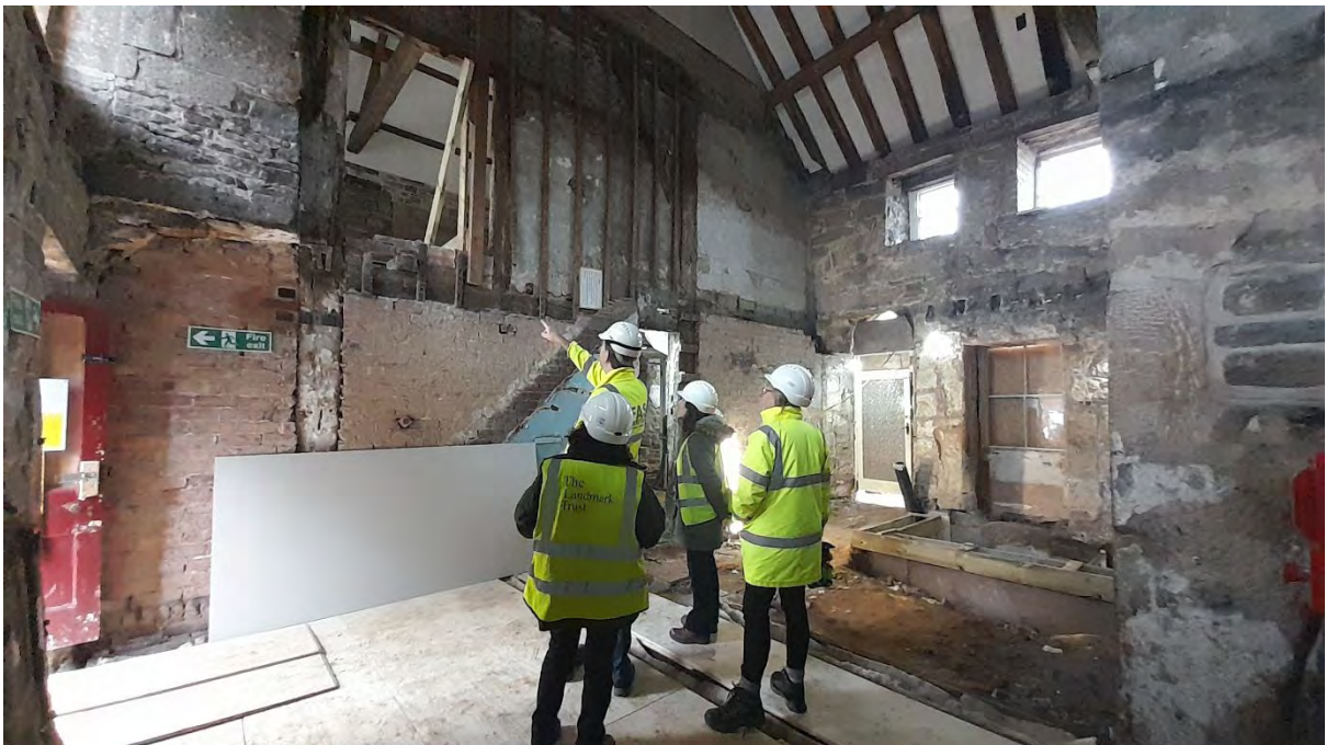
Analysing the evidence in the Entrance Hall, its cottage infill now removed. This was once the cross passage for the 1480s Great Hall. Before this hall was built, a narrow gallery would have run along the far wall, with an external staircase providing access to the 1320s first floor hall via the present doorway. The early cesspit that disproved the current Great Hall as the site of the original hall block was discovered against this wall, near the greenish door in this image. Above it, the timber frame has evidence that could suggest a long drop garderobe.
