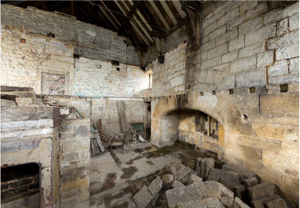
The Great Hall in 2020. The remains of cottage chimney breasts have yet to be cleared. While they remained in situ, it was impossible to find a viable alternative use for the Great Hall. Heaps of carefully salvaged stone and other materials lie on the original flagstone floor.
