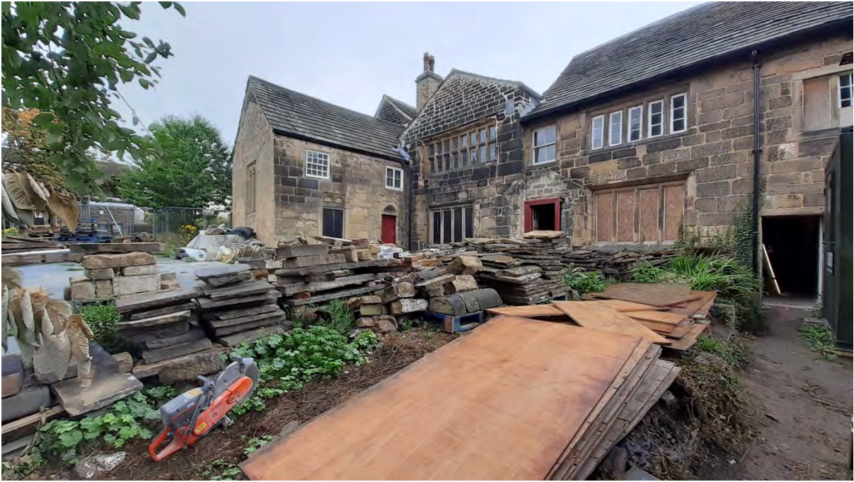
By summer 2022, the scaffolding was down and site set-up complete. The flagstones from the Great Hall had been recorded and were now carefully stacked while underfloor heating was installed.
