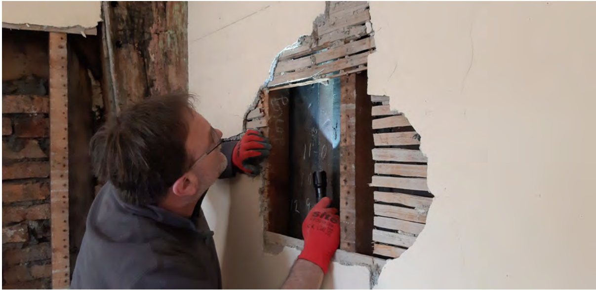
With traces of paint clearly apparent on the revealed corner jowl post, investigations were taken further.
