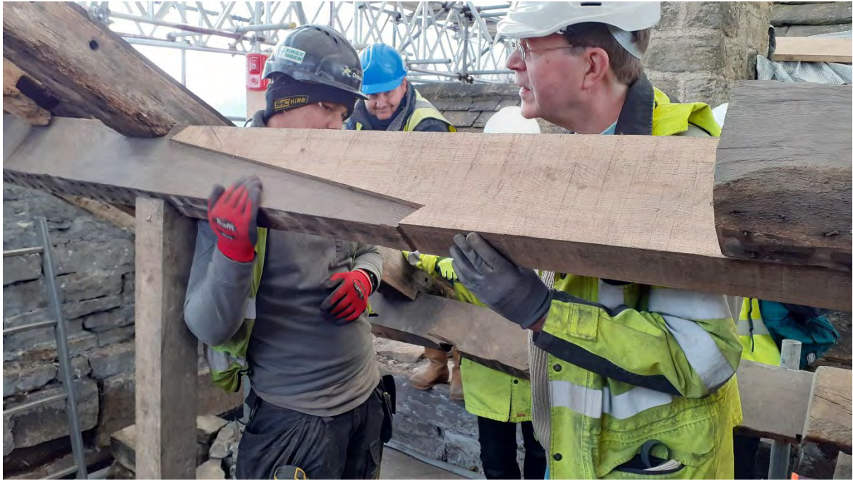
Archaeologist Jonathan Clark inspects a scarf joint repair to a decayed purlin.
