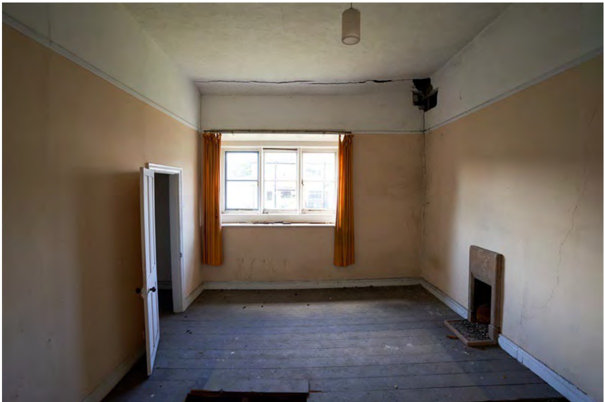
The Painted Chamber as cottage bedroom in 2019. Apart from the corner jowl post and hint of a coved ceiling in the top picture, there was little suggest that there was anything of significance. Only the small mid-20 th fireplace and slight shadowing in the plaster hinted at a bigger hearth.
