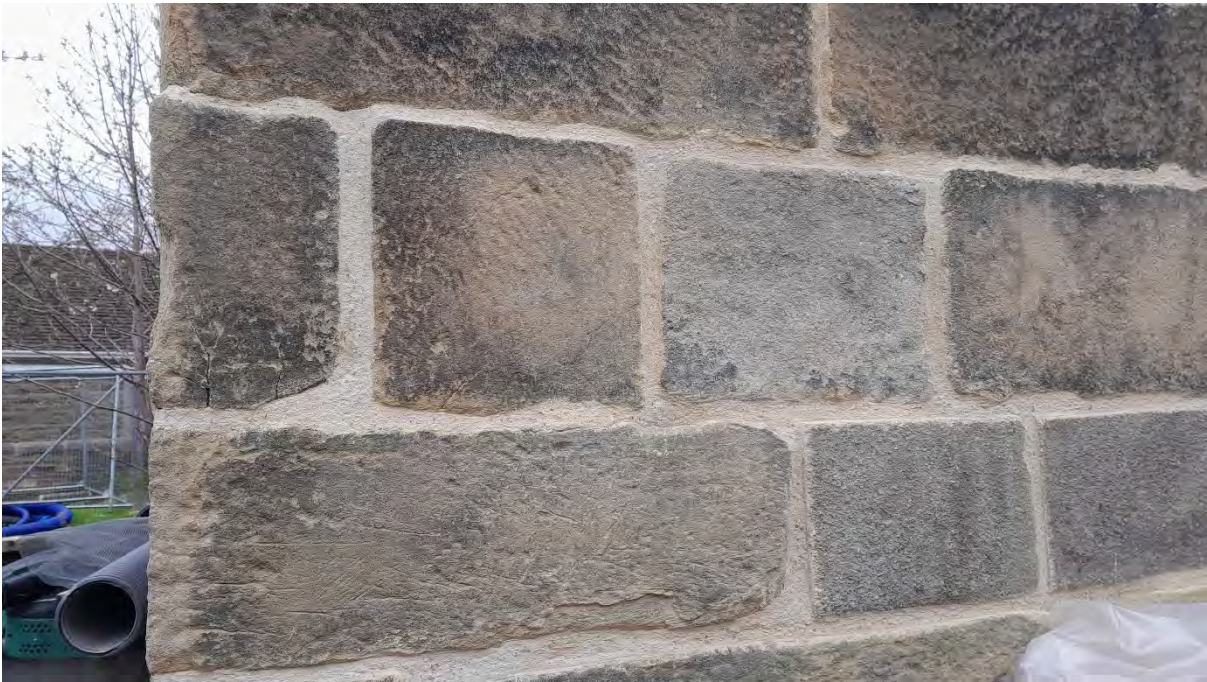
From top left: slaking lime on site; tile repairs in one of the many wall cavities, here in the partition wall of the Great Hall; a sample of external pointing, the mortar mix and style refined with great care by Dobsons'
