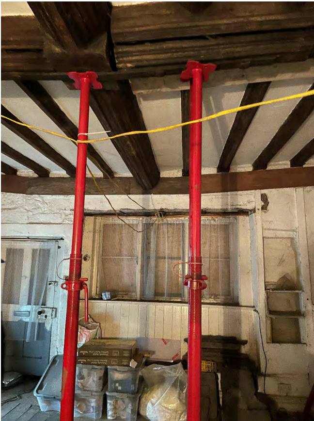
Left: the cottage sitting room (now a bedroom) propped as a precautionary measure. Right: the cottage stairs before removal. By now, the wall paintings had been discovered in the room above and can be glimpsed beneath protective Perspex on the left. Below: the room midway through works. The former breach in the ceiling for the staircase has been made good. The far wall has yet to be finished. The new staircase for the adjacent cottage is under construction.
