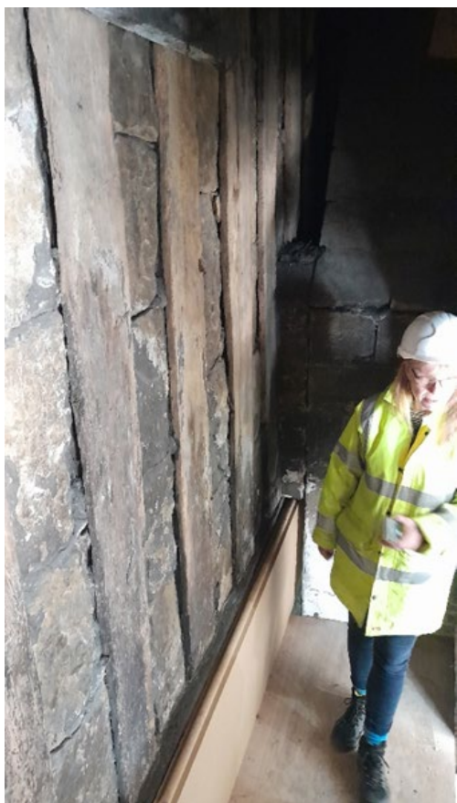
Remnants of a canvas patch used to disguise a mortice hole in the wall plate, tacked in place by the Calverley artist.
