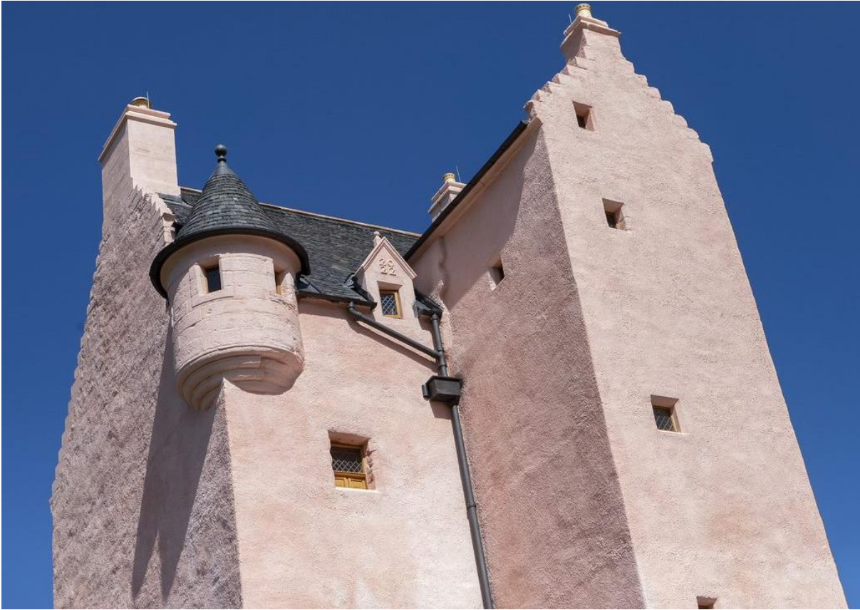
The stair turret, one of the two bartizans and the dormer with its datestone, all reconstructed along with the inhabitable top storey in 2020-22. They were originally added to the main tower c1600.
