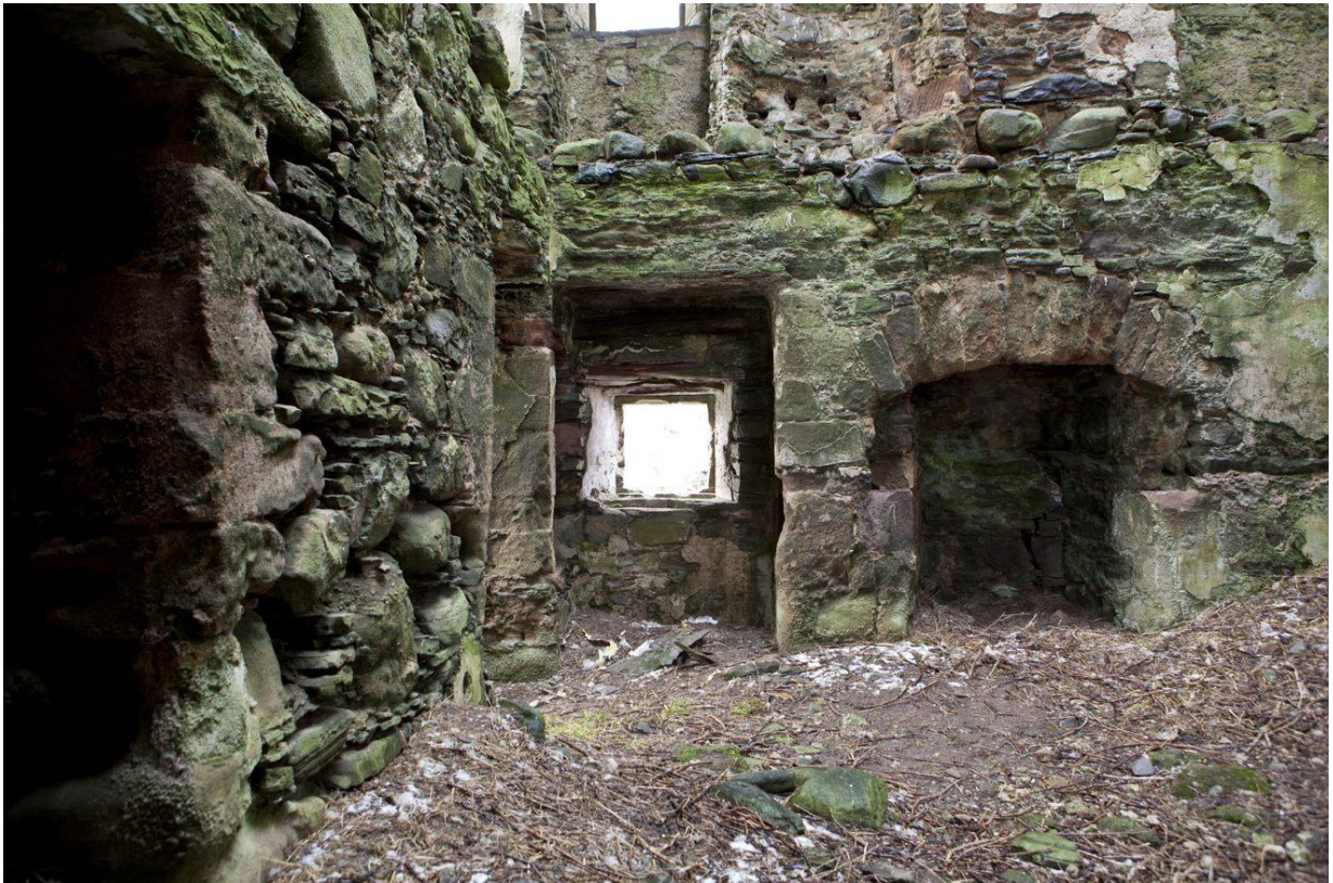
Top: the cellar with its gun ports and finely constructed vault, off which the tower is built.
