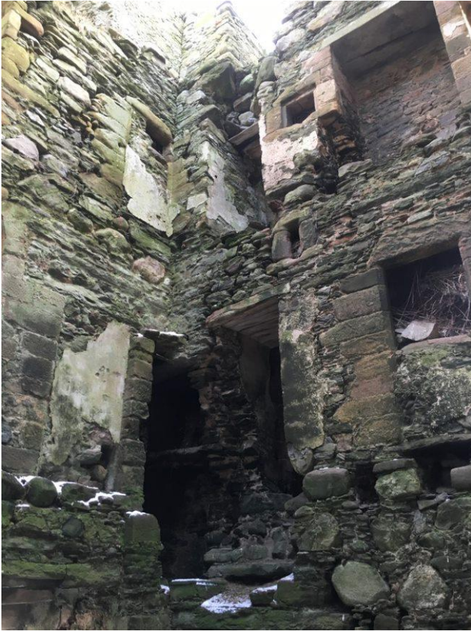
View from today's kitchen of the main entrance.
