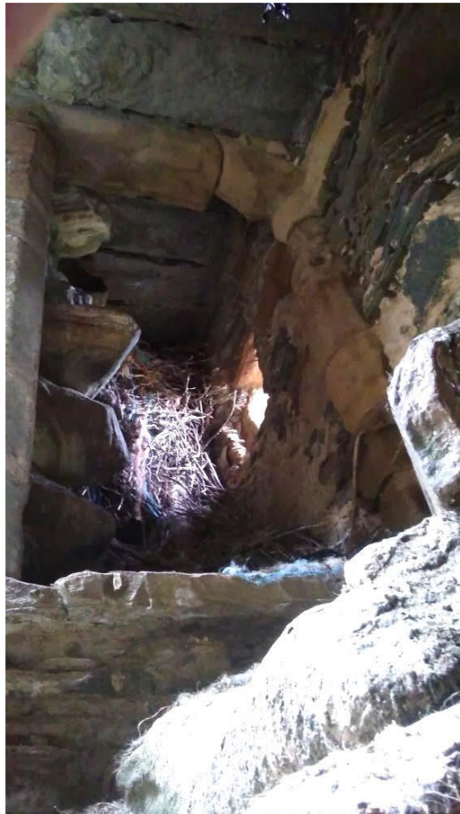
Interior of the former turnpike stair that wound up inside the walls of the upper storeys. A few stone stair treads remained at the upper level (left). The entrance vestibule to the second floor (right).
