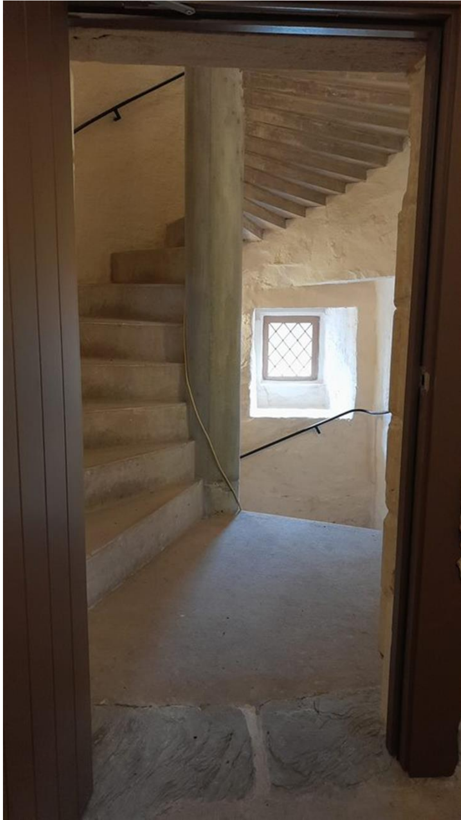
A section of the completed concrete stair.
