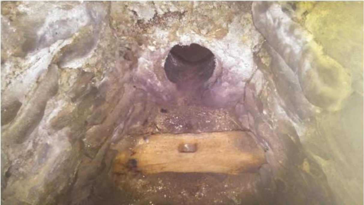
Gun port on east side of cellar with very rare surviving timber beam and pivot support for a firearm.
