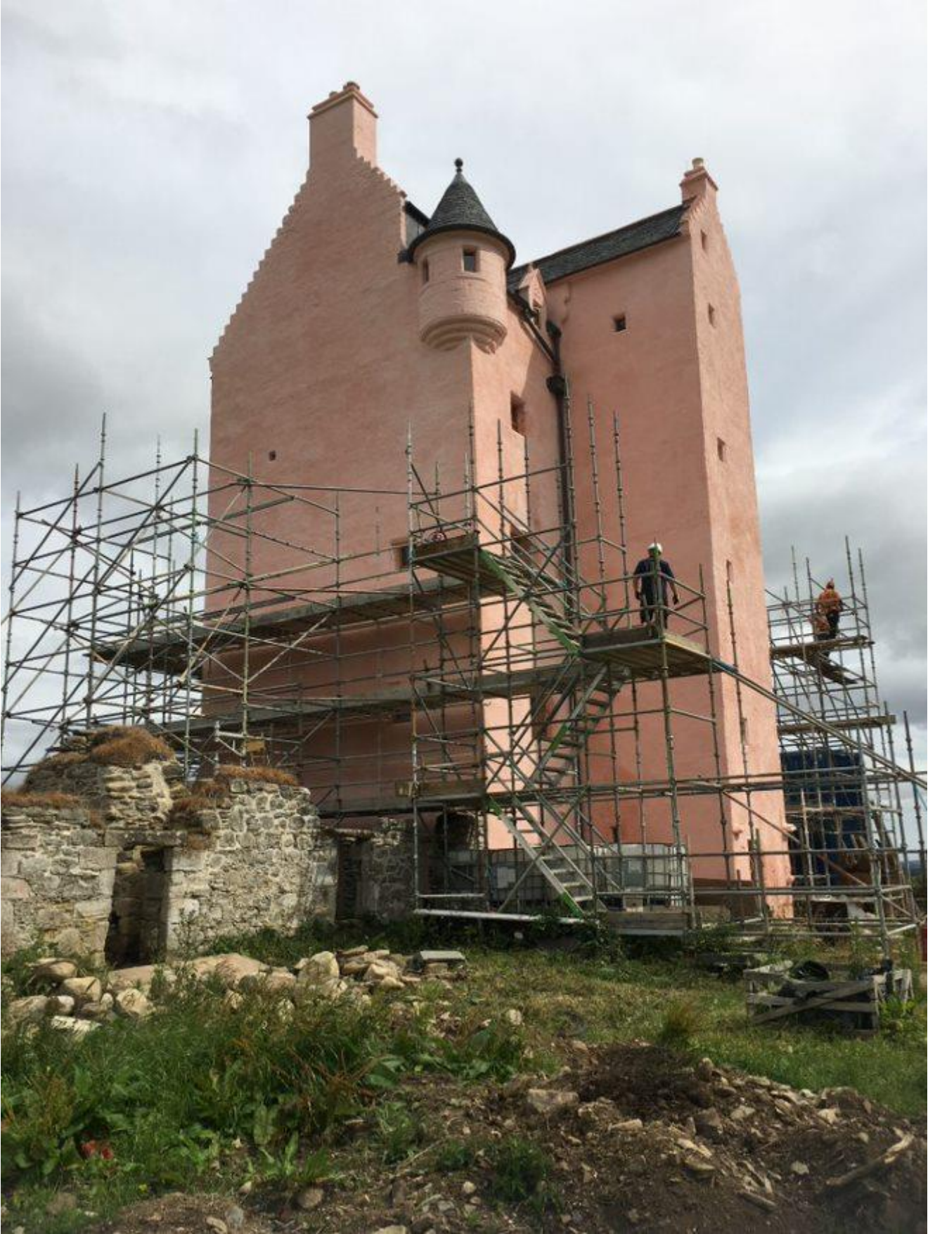
By August 2022, the tower was finally emerging from its chrysalis of scaffolding.
