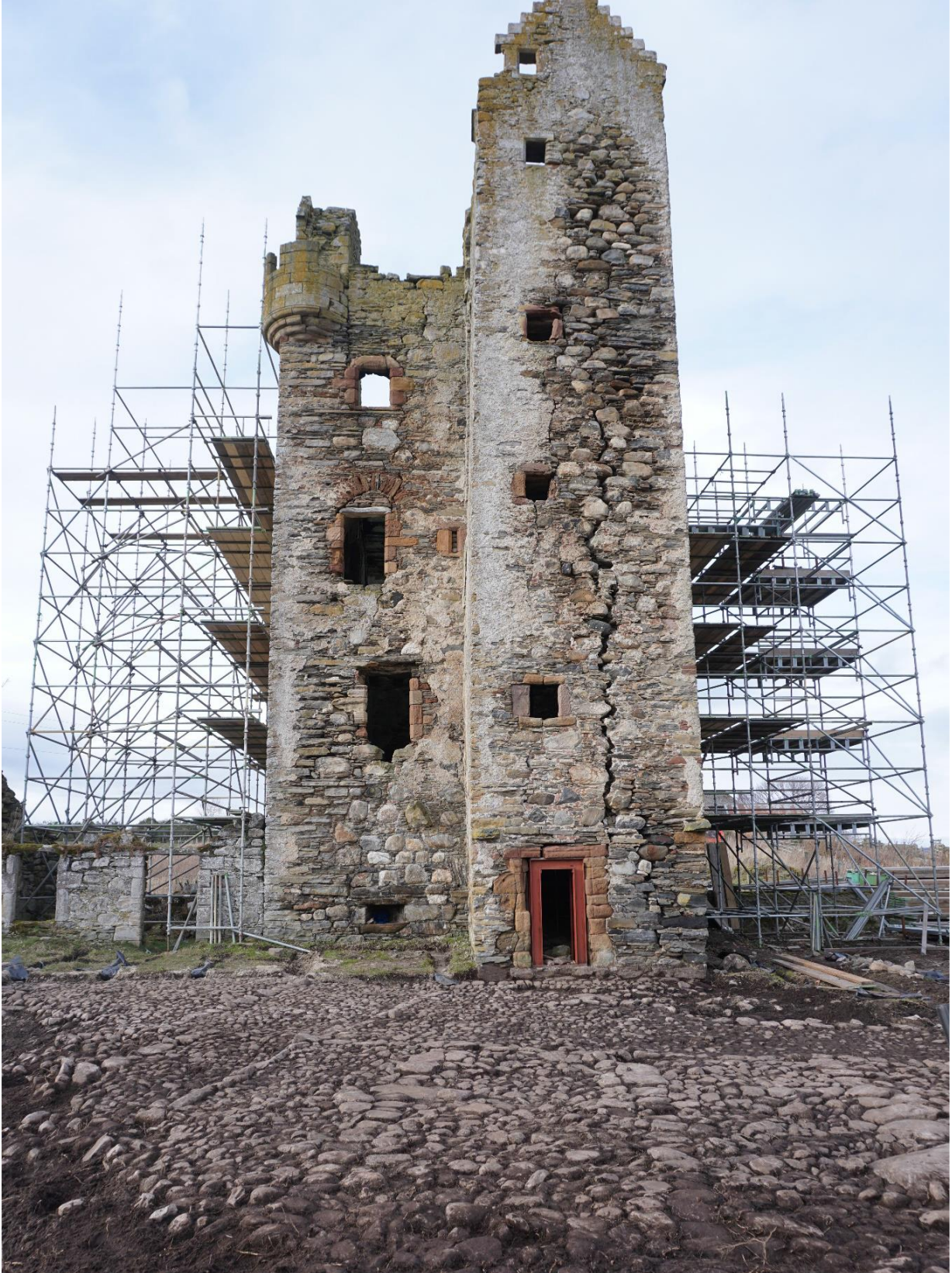
View of the tower from the south after excavation of the cobbled surfaces, March 2020.
