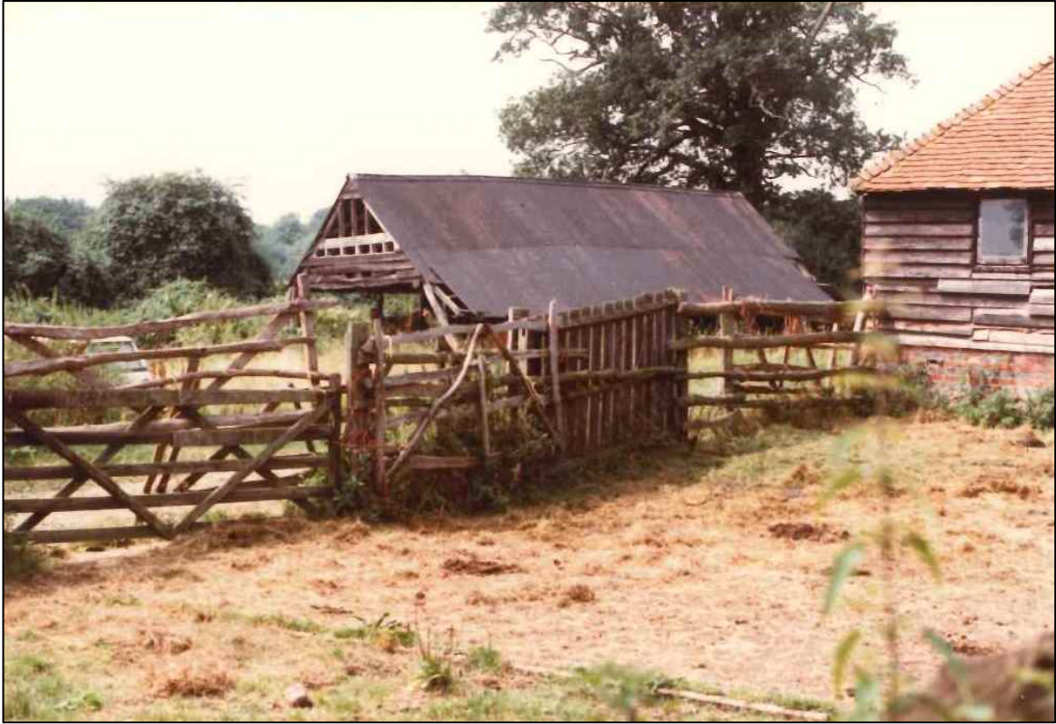
The demolished cartshed.
