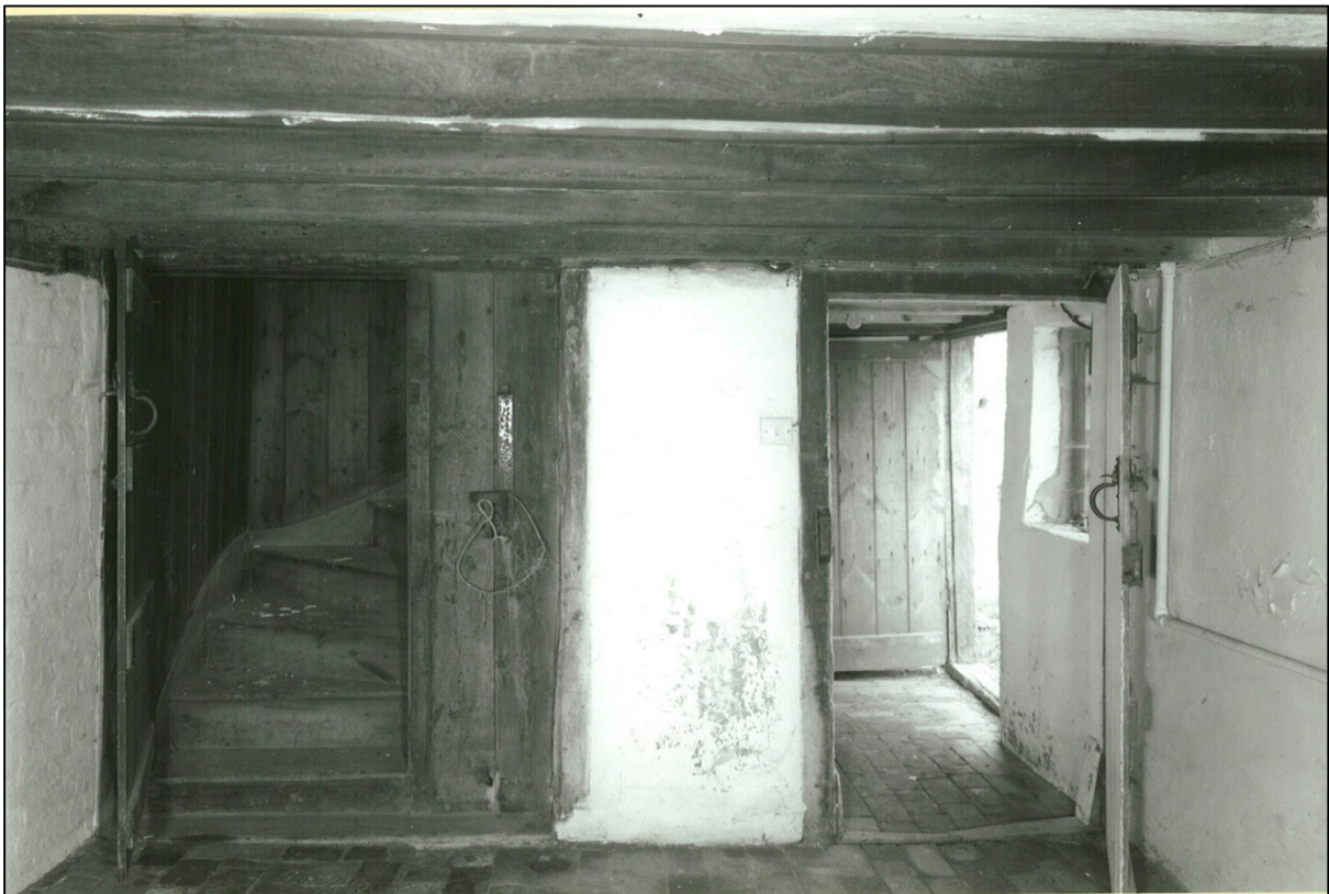
The back hall with the second staircase now removed.
