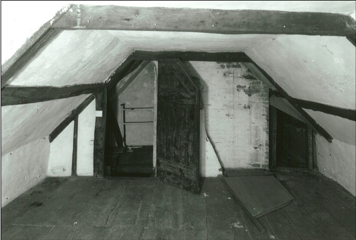
The attic room.
