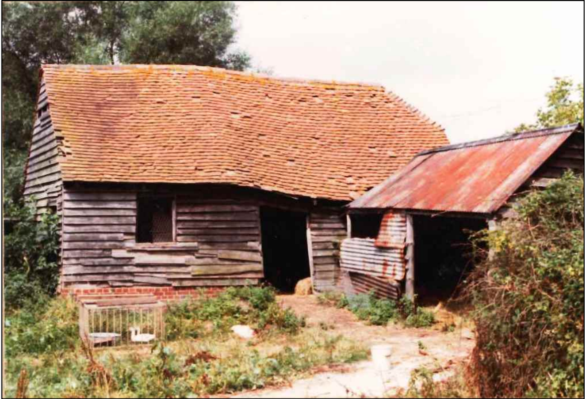
The cow byre with attached shed.
