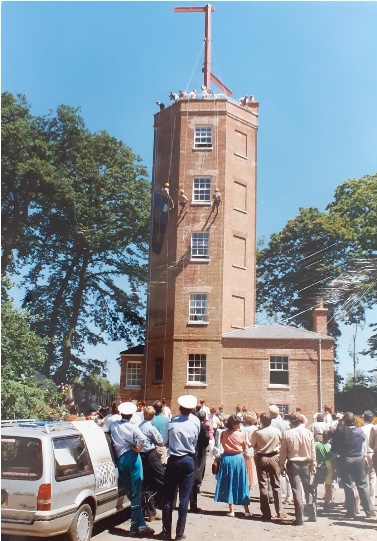
The reopening of the newly restored tower in 1988 saw sea cadets abseiling down from the roof as well as demonstrations of the semaphore.
