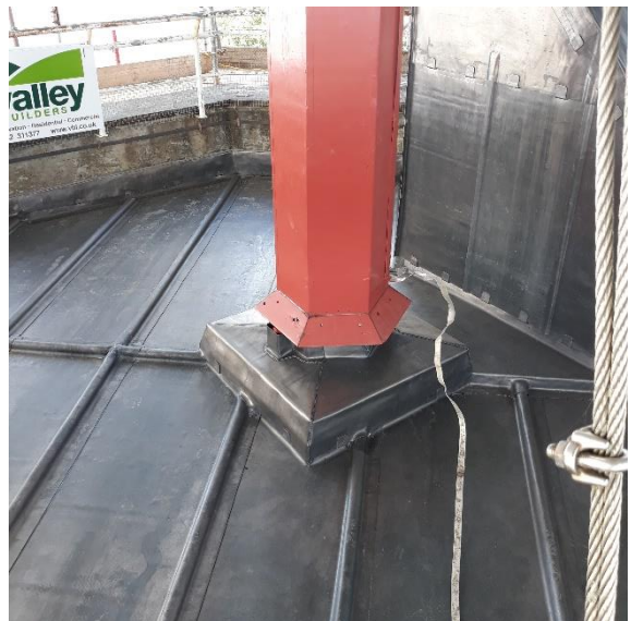
Mast repairs: left to right from top: base on roof before repair; corroded iron from base; scarf repair to arm; repaired base in kitchen; fully repaired top arm; re-leaded
