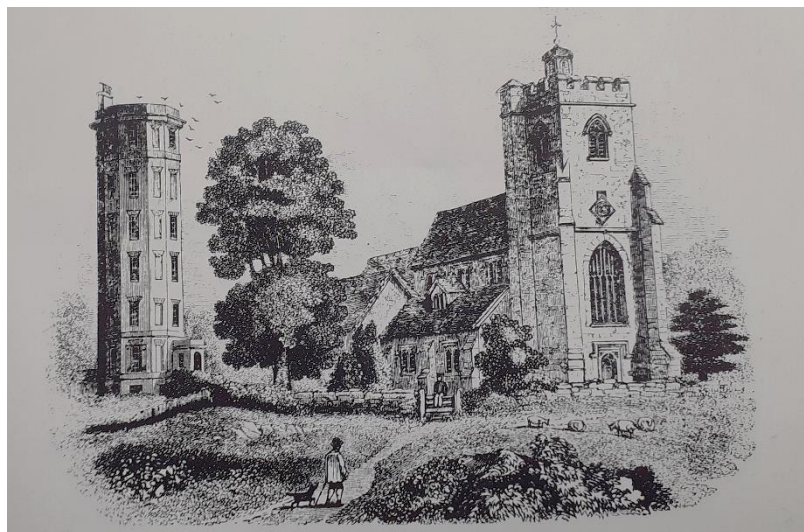
Worplesdon Glebe Station, another five-storey tower nearby on the projected Plymouth line, demolished in 1851. (The unknown artist wrongly depicted six
