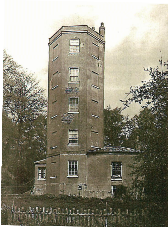
The Semaphore Tower in 1962. The mast had long been dismantled and the tower was clad in an ill-advised cementitious render. (Historic England Archive)
