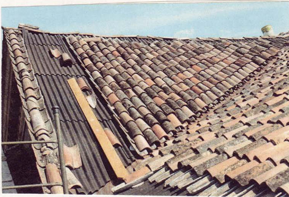
North pediment: cornice and valley.
