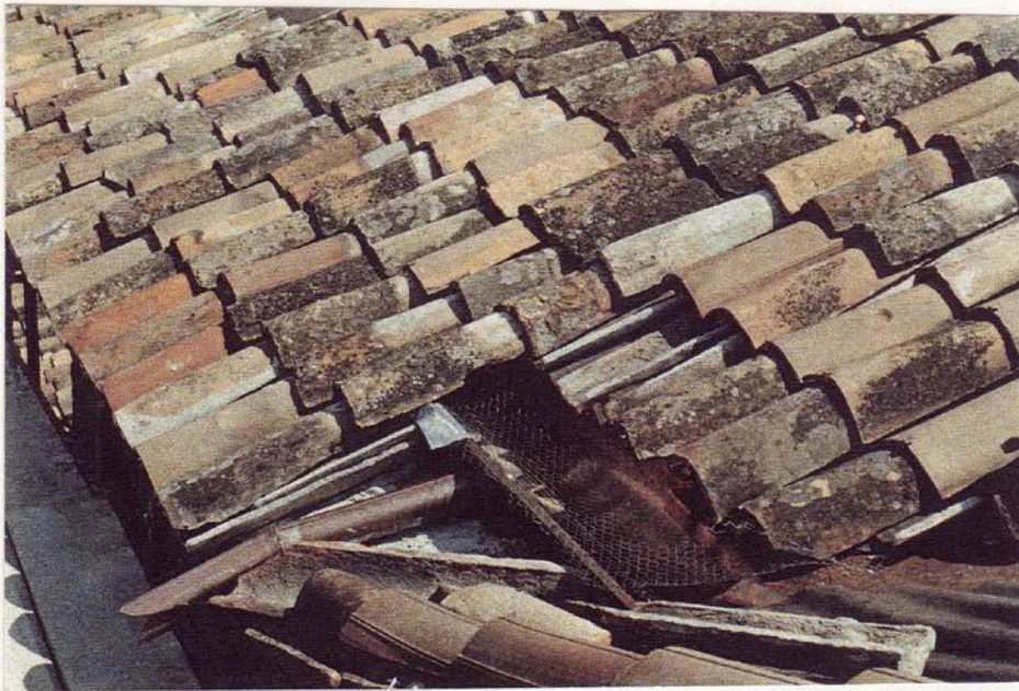
Making the secret gutters and rain-water spouts.
