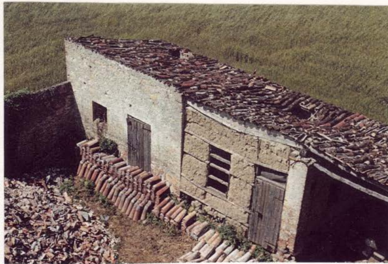
chicken houses in the north-west corner of the estate, demolished 1992.
