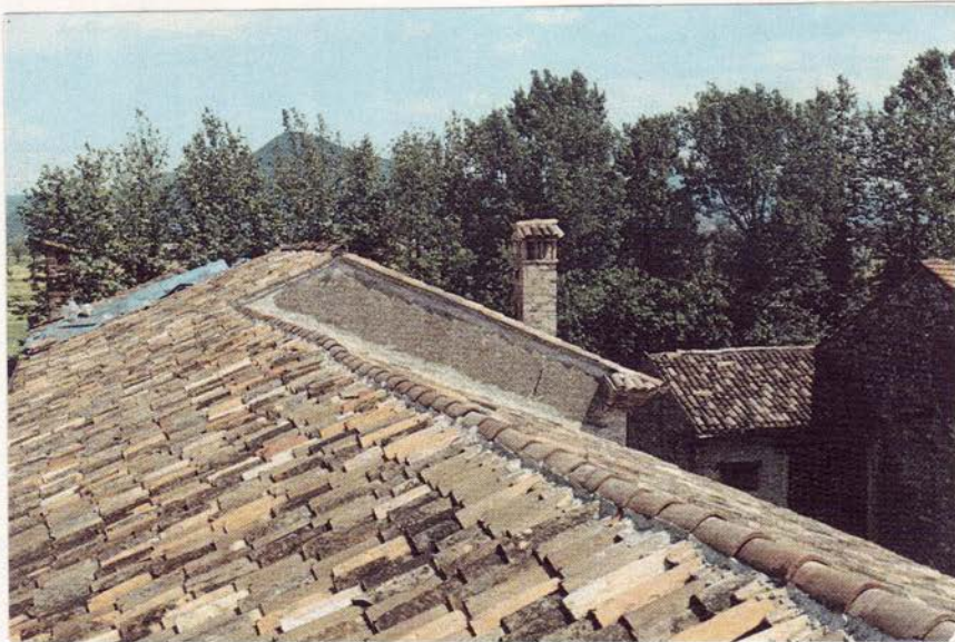
Re Carchessa roof seen from above.
