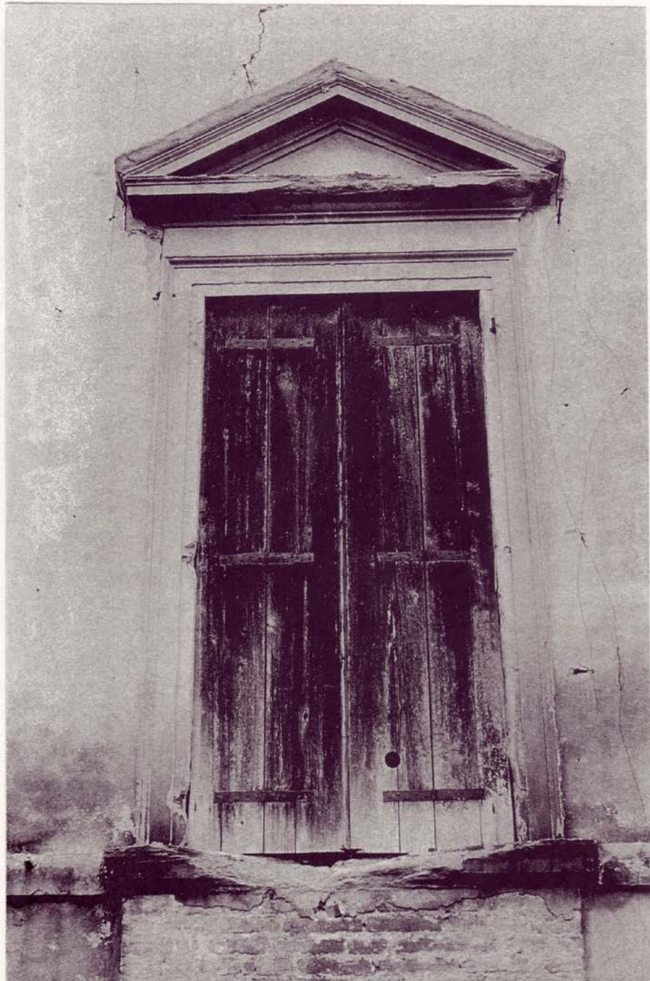
best window of south front, with 19 th century shutters.
