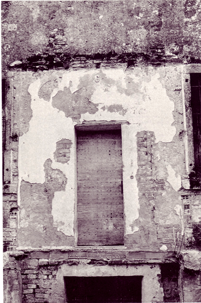
East window of north front after removal of pantry.
