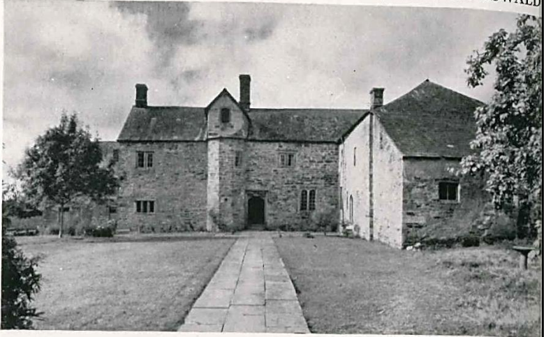
1.—FROM THE SOUTH: THE BACK OF THE HOUSE AND THE EAST WING
