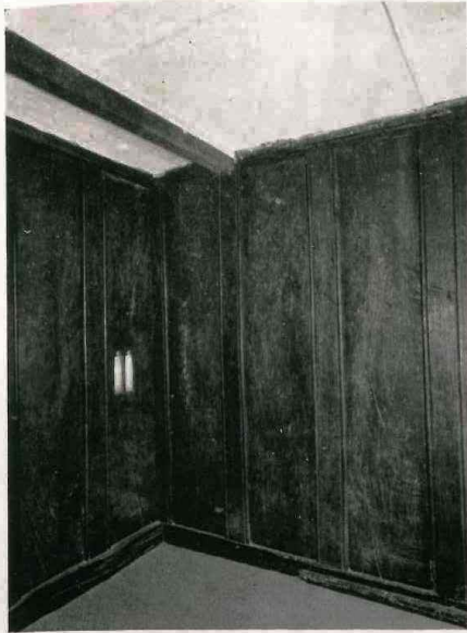
9.—POST-AND-PANEL PARTITIONING IN THE CLOSET WEST OF THE HALL CHAMBER, WITH A LITTLE WINDOW CUT IN ONE OF THE PANELS
