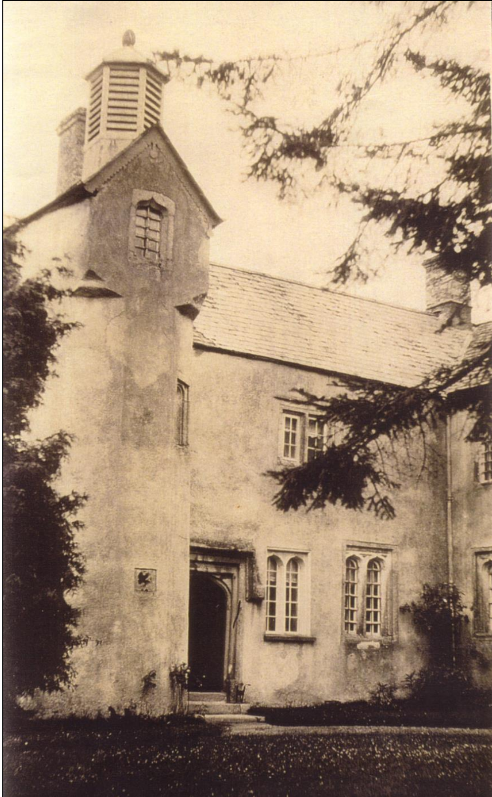
The south elevation, which is again shown rendered. The window to the right of the doorway no longer exists; nor does the lantern on top of the stair turret.
