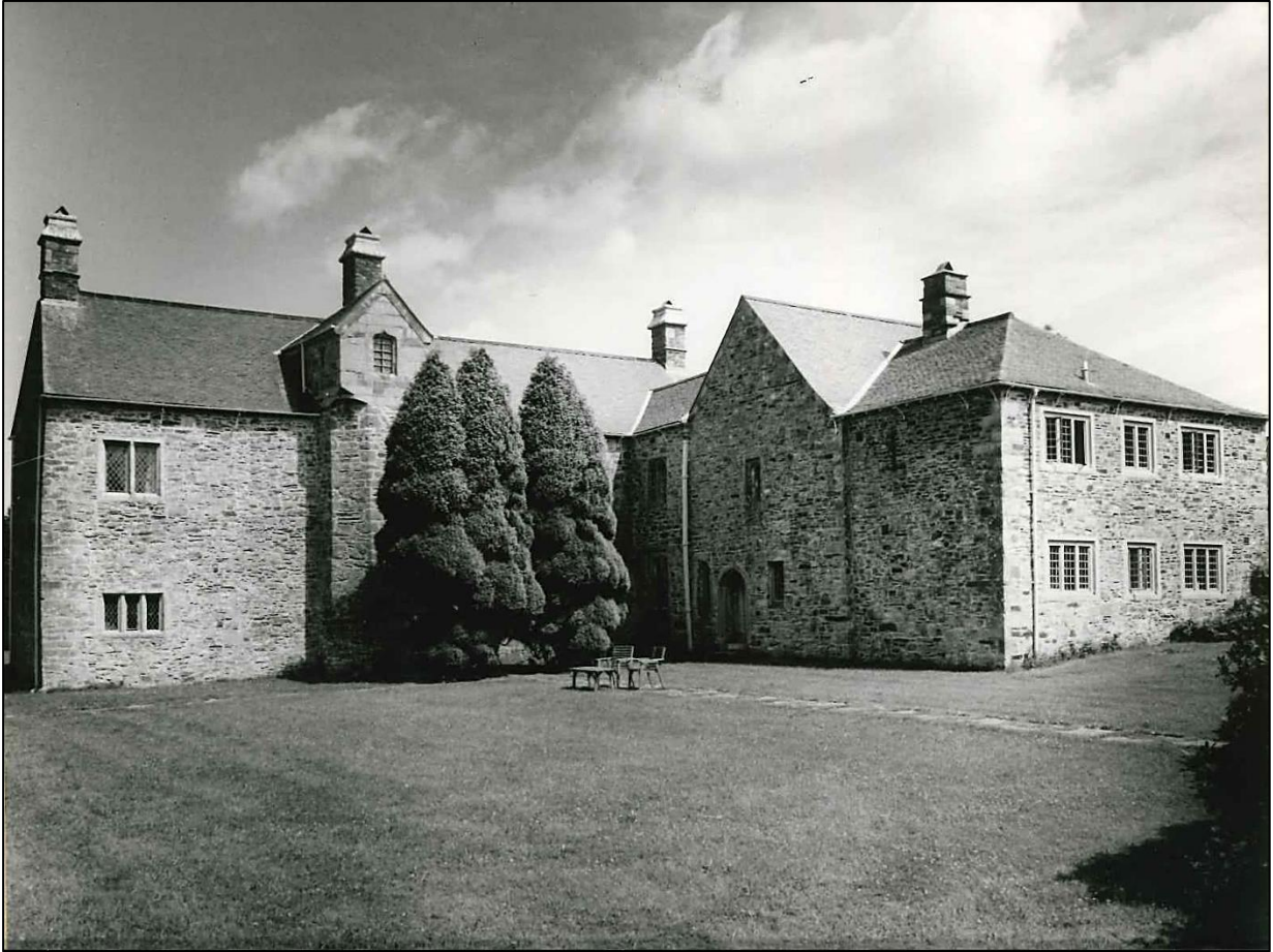
Cypresses Leylandii flourishing outside the south screens door.
