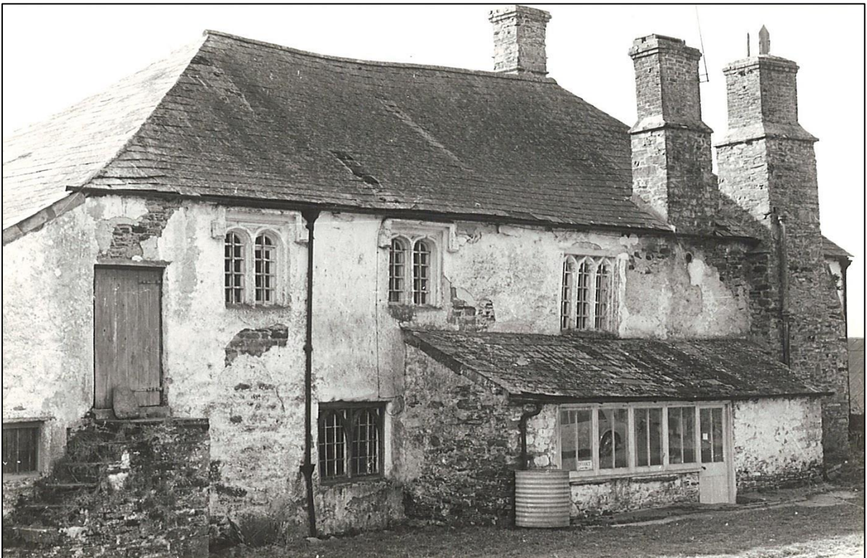
The east elevation before restoration.
