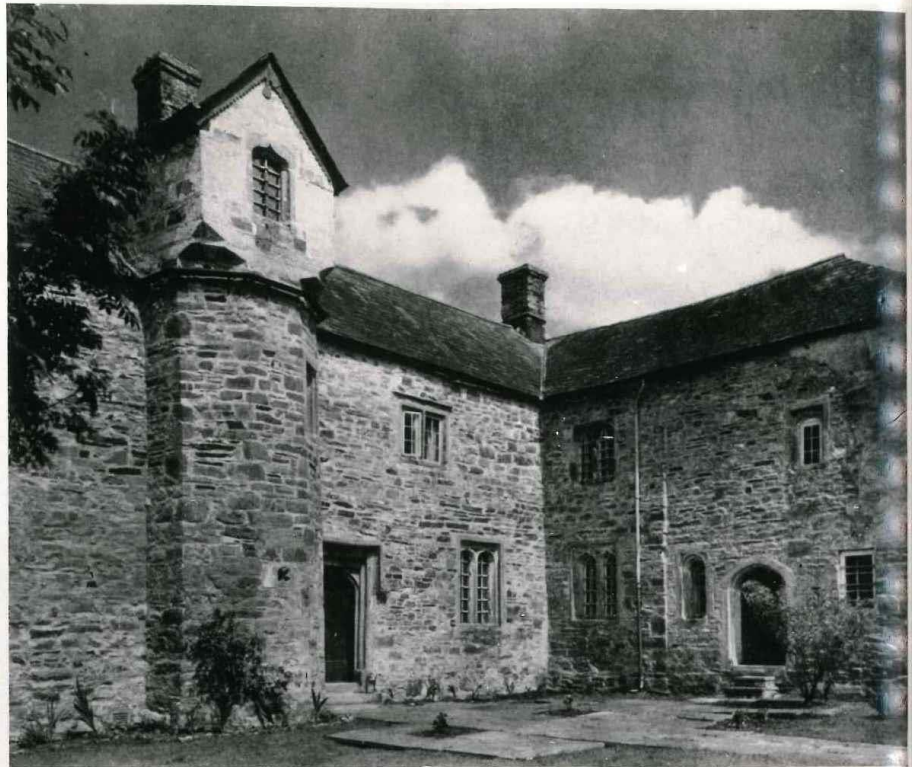
3.—FROM THE SOUTH-WEST. THE EAST WING ( right ) WAS EXTENDED FROM THE BREAK IN THE WALL EARLY IN THE 16th CENTURY
