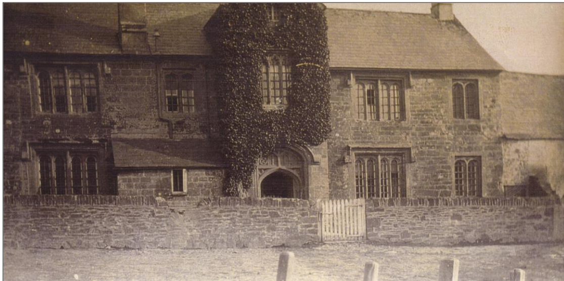
North elevation. The lean-to to the left of the entrance and the outbuildings to the right of the house no longer remain.
