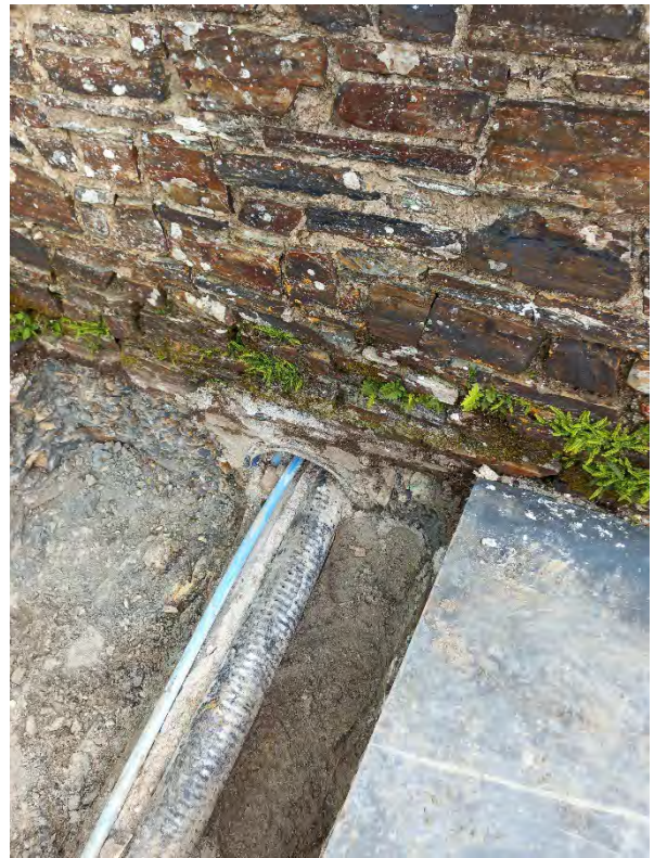
Spring/summer 2024: drilling the boreholes and laying the pipes for the new GSHP heating and hot water was a major undertaking.
