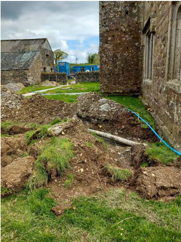
Spring/summer 2024: drilling the boreholes and laying the pipes for the new GSHP heating and hot water was a major undertaking.
