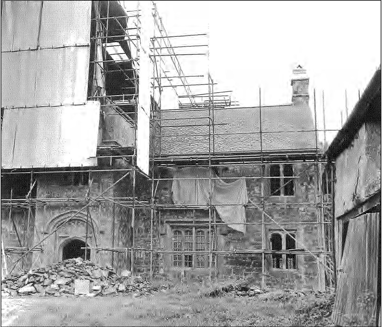
Wortham under repair, February 1974. From ' The Western Morning News .'
