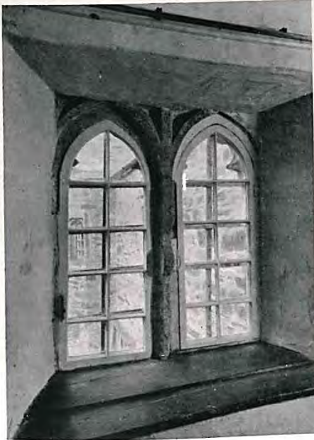
10.—A 15th-CENTURY WINDOW REBATED FOR WOODEN SHUTTERS. (Right) 11.—POST-AND-PANEL PARTITION IN THE EAST WING
