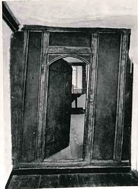
10.—A 15th-CENTURY WINDOW REBATED FOR WOODEN SHUTTERS. (Right) 11.—POST-AND-PANEL PARTITION IN THE EAST WING
