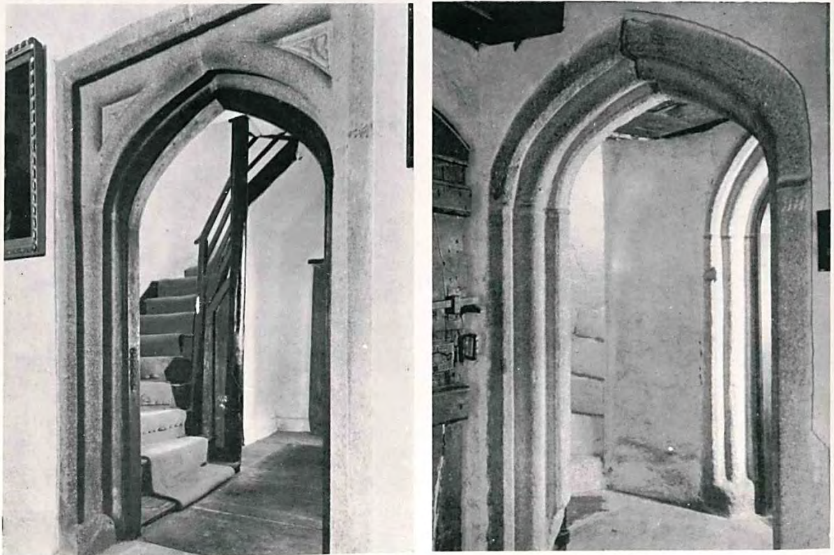
4.—A 15th-CENTURY GRANITE DOORWAY IN THE SOUTH WALL AT THE EAST END OF THE HALL. (Right) 5.—EARLY-16th-CENTURY DOORWAY IN THE WEST WALL OF THE HALL OPENING TO THE NEWEL STAIR AND THE PARLOUR
