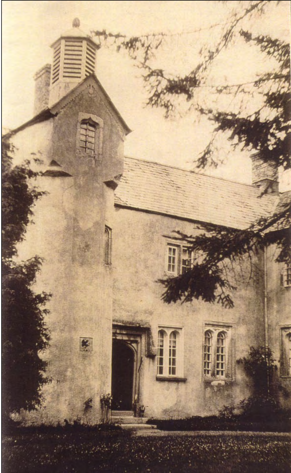
The south elevation, which is again shown rendered. The window to the right of the doorway no longer exists; nor does the louvered lantern on top of the stair turret.
