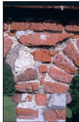
Eroded bricks and poor repairs to the parapet before work began.
