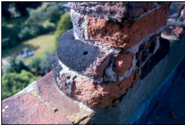
Eroded bricks and poor repairs to the parapet before work began.
