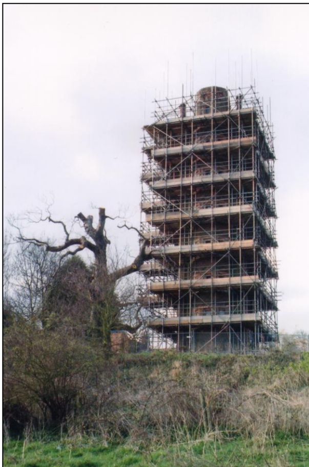
Early spring 2003: scaffolding up...
