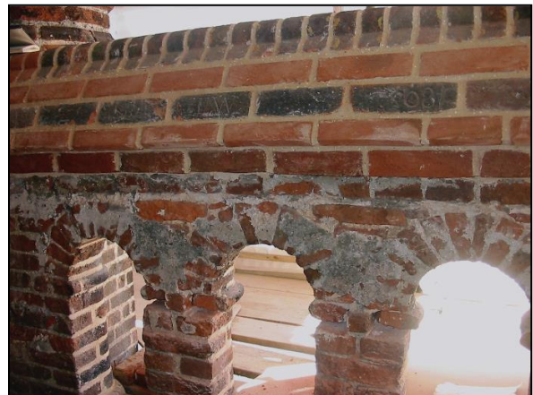
The finished job, old bricks carefully reused with clumsy former repairs also apparent
