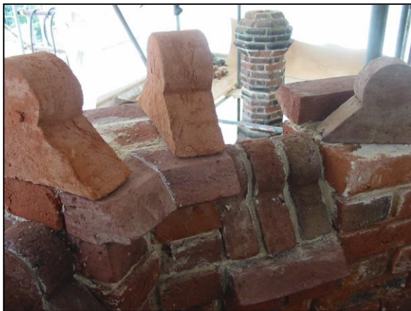
Coping stones waiting to be set.
