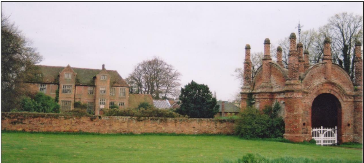
The idiosyncratic gatehouse at Erwarnton, probably built by a contemporary of Thomas Gooding though dated by Pevsner to 1549 on heraldic grounds.
