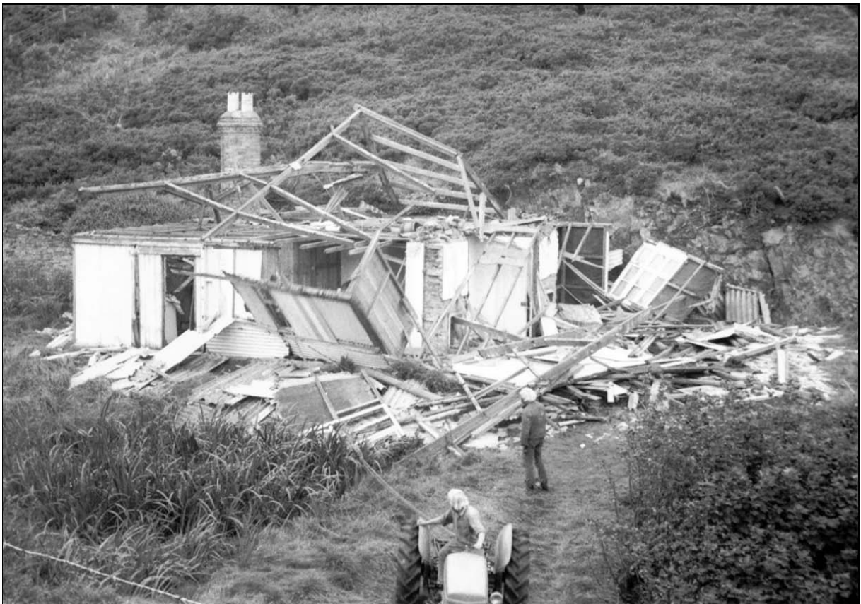
Brambles being demolished
