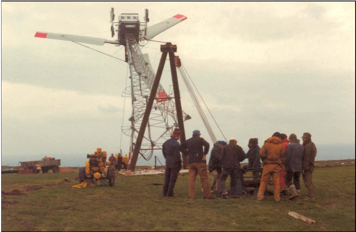
Raising the aerogenerator in 1982
