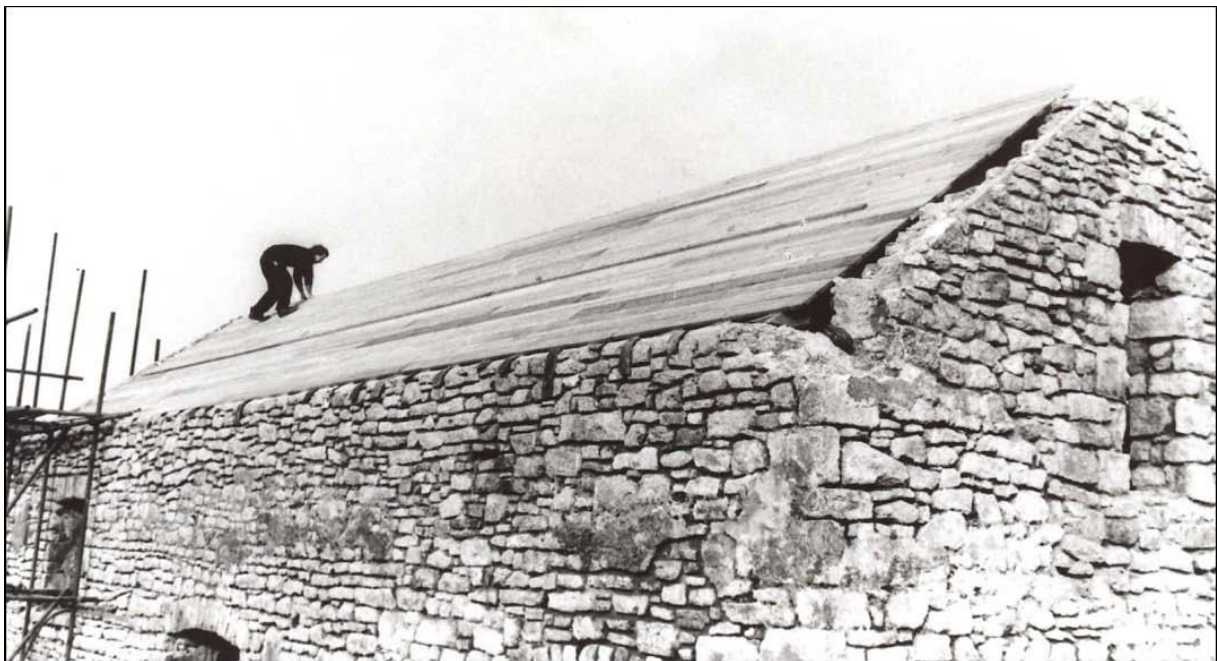
Renewing the Barn roof
