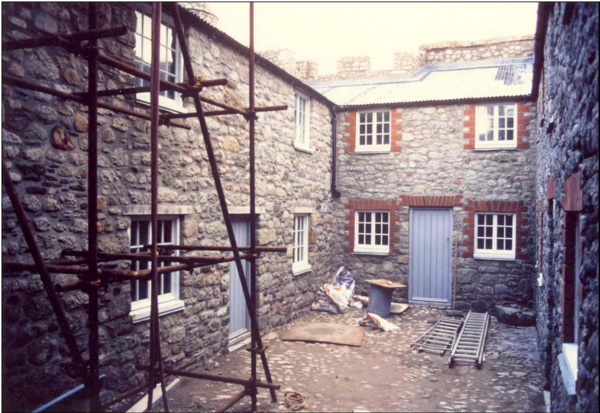
The interior of the Castle being restored in 1980
