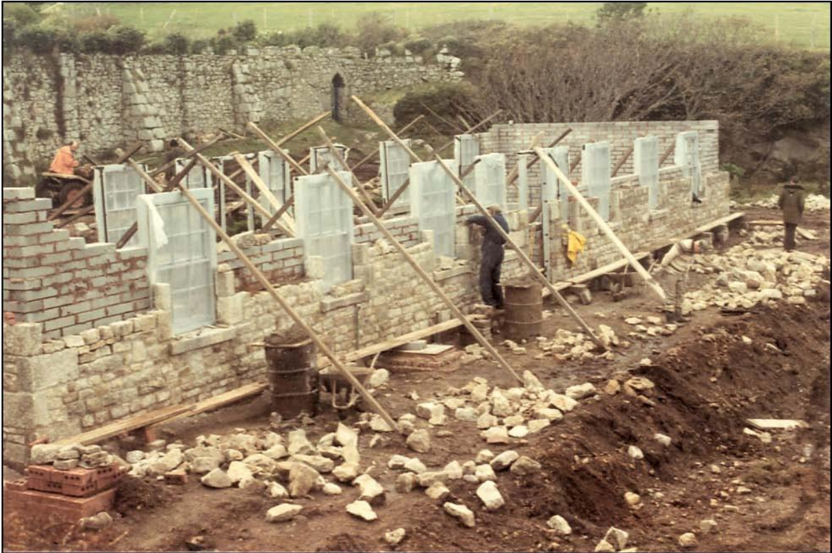
Raising the walls
