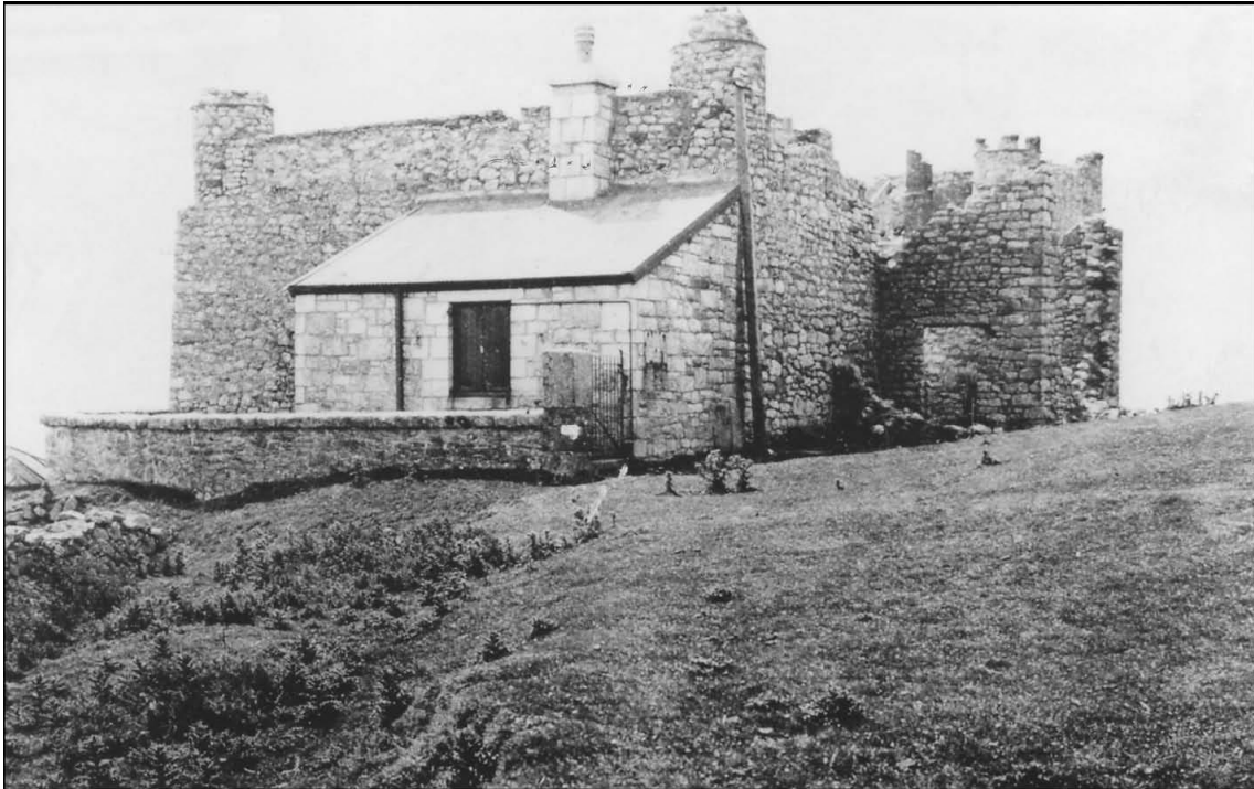
The Cable Hut
