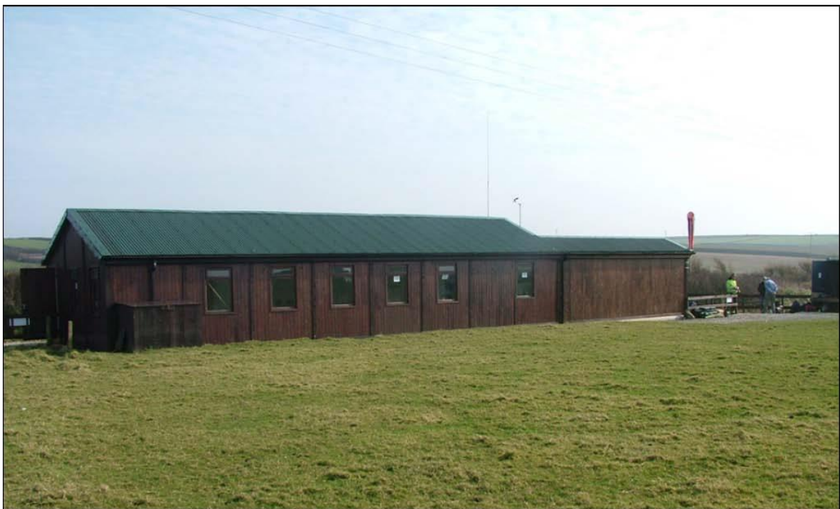
The improved terminal building at Hartland Point heliport
