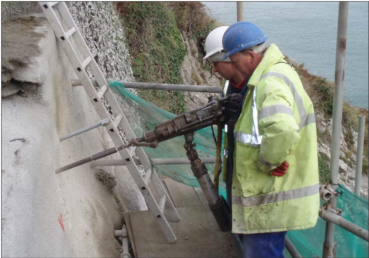
Stabilization work on the Beach Road
