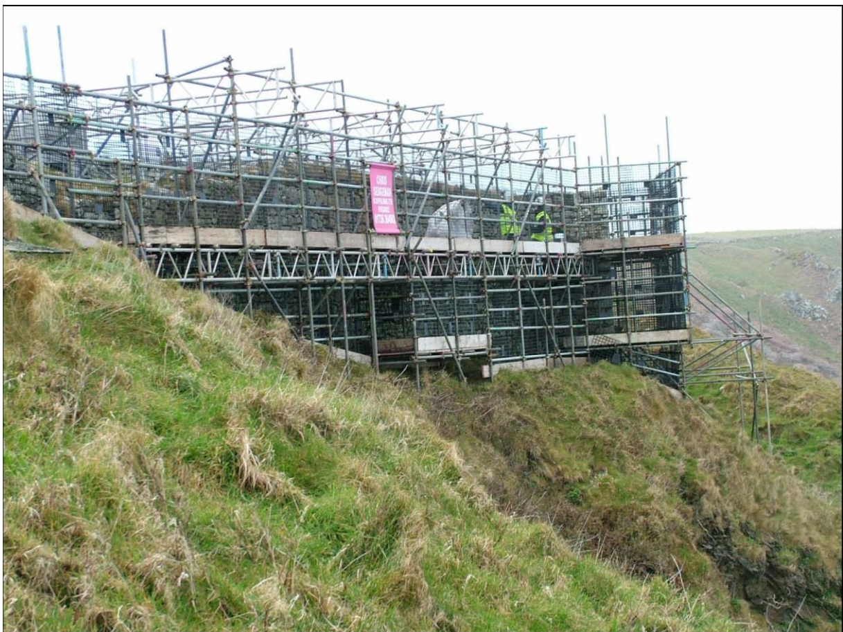
Repairing and re-pointing the exterior bailey wall in May 2013
