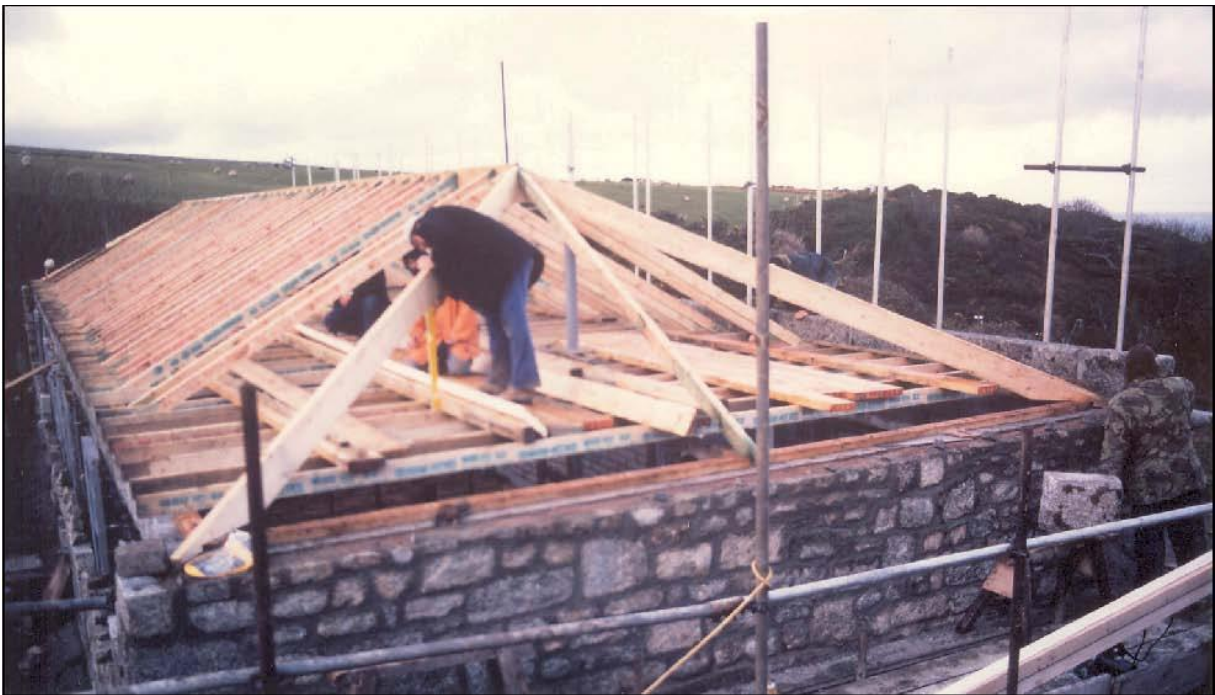
Building the roof
