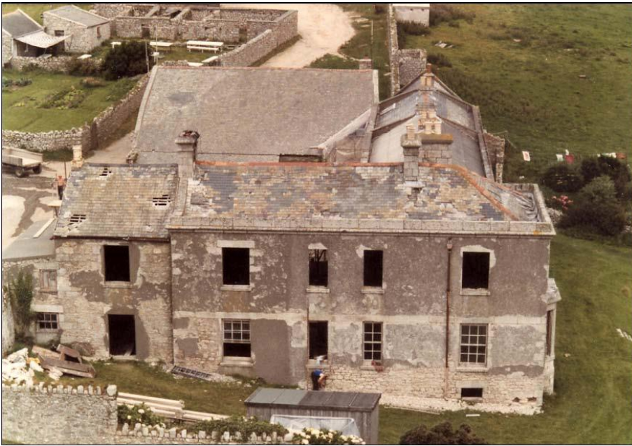
The Big House stripped and ready for demolition
