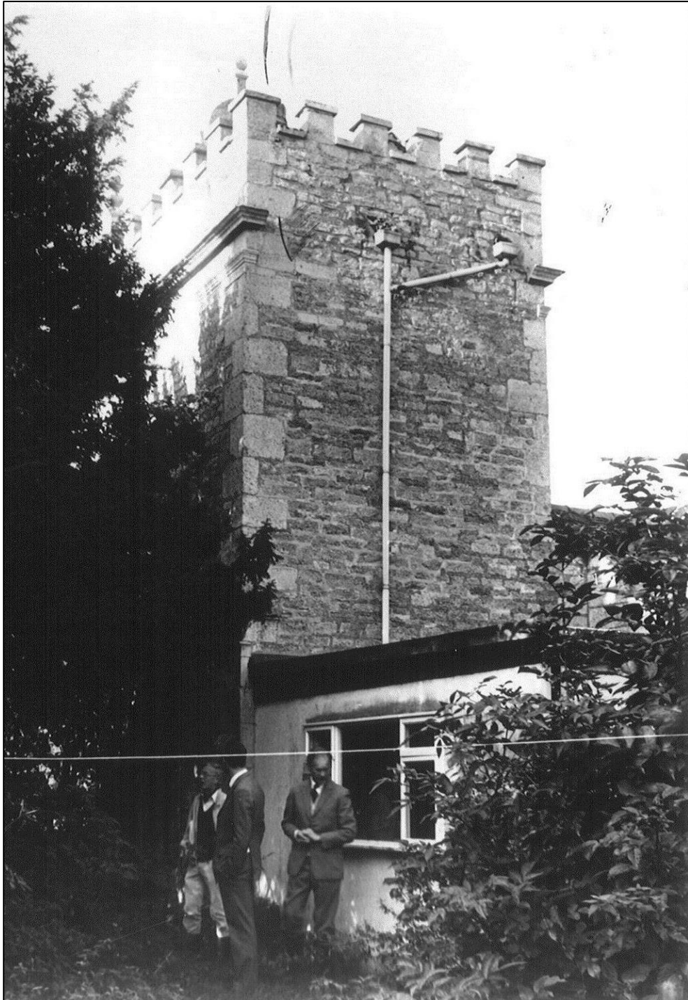
An early reccy around 1981 by Landmark's founder Sir John Smith (right) of the back of the Lodge showing the flat-roofed extension removed by Landmark.
