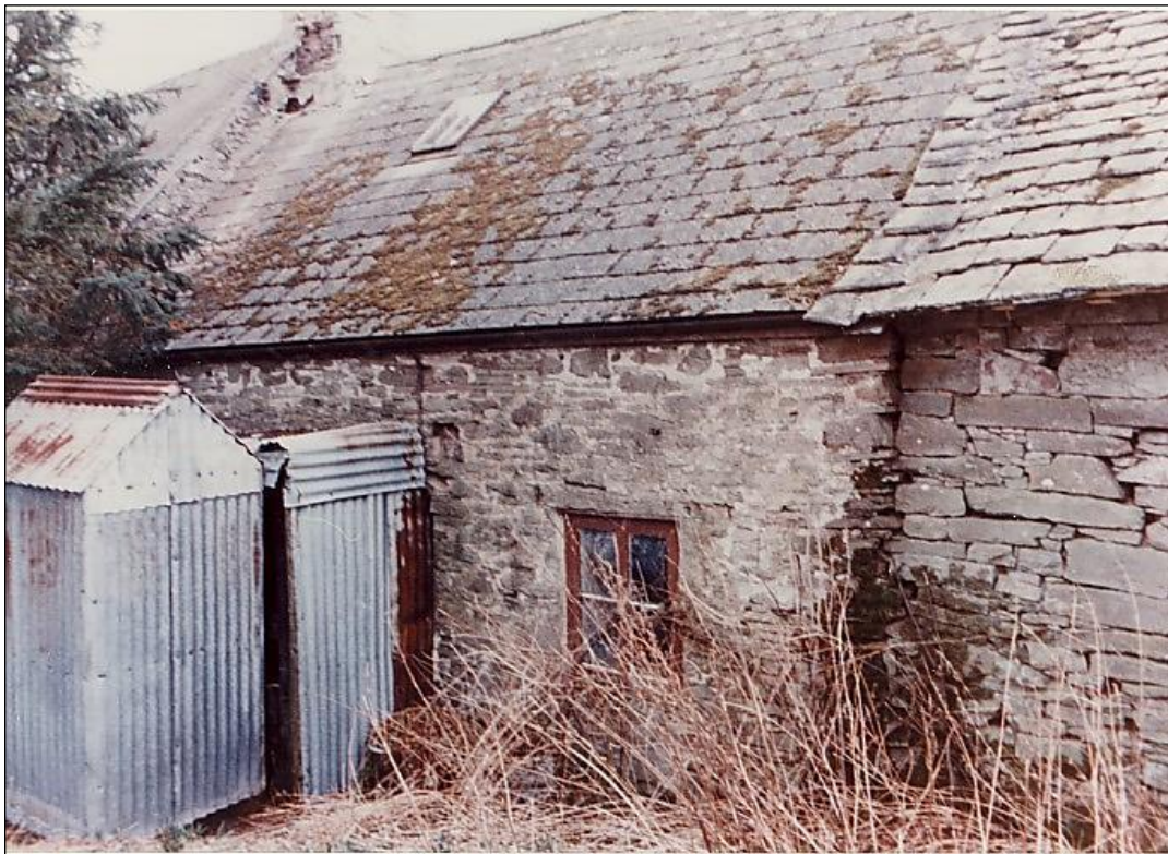
Lean-to sheds at the back before removal.
