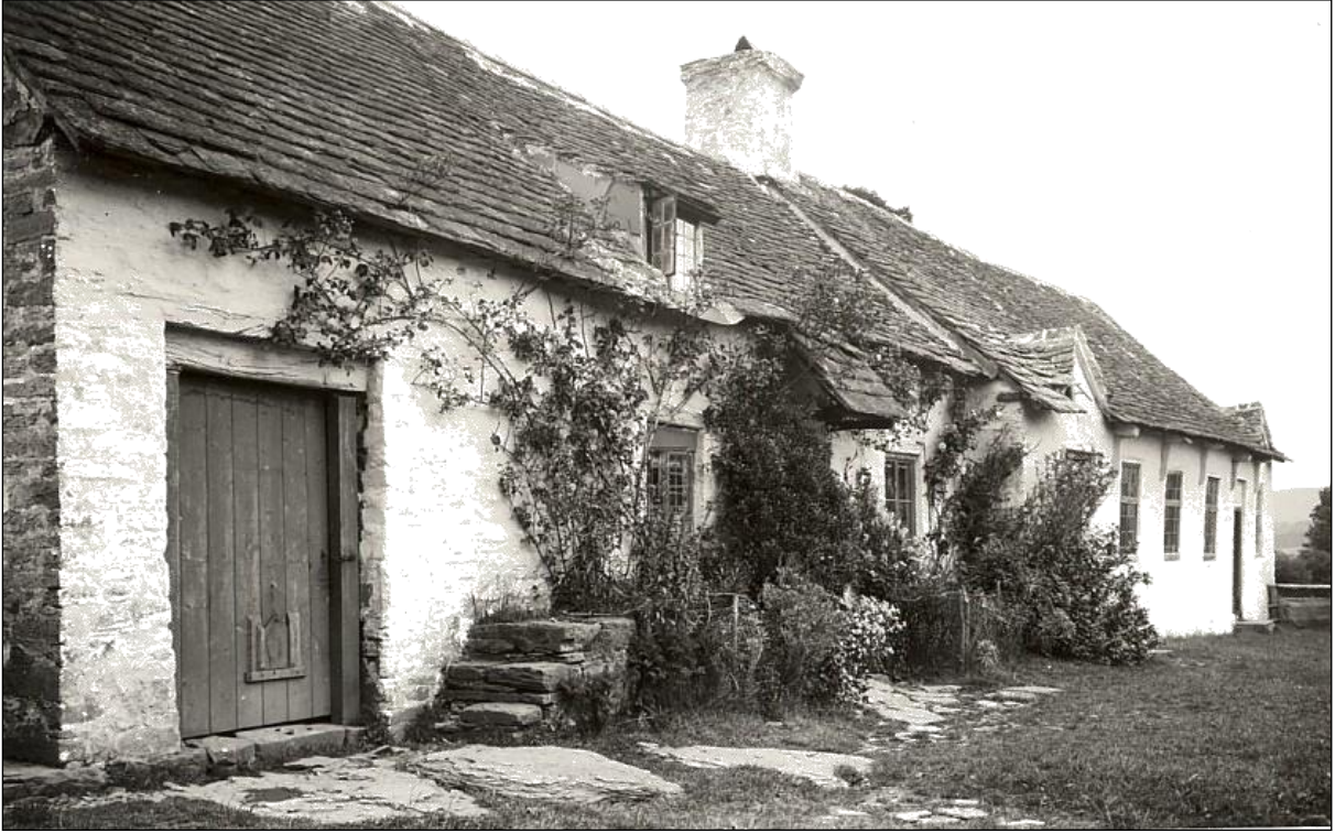
Maesyronnen Chapel and cottage before restoration by Landmark.
