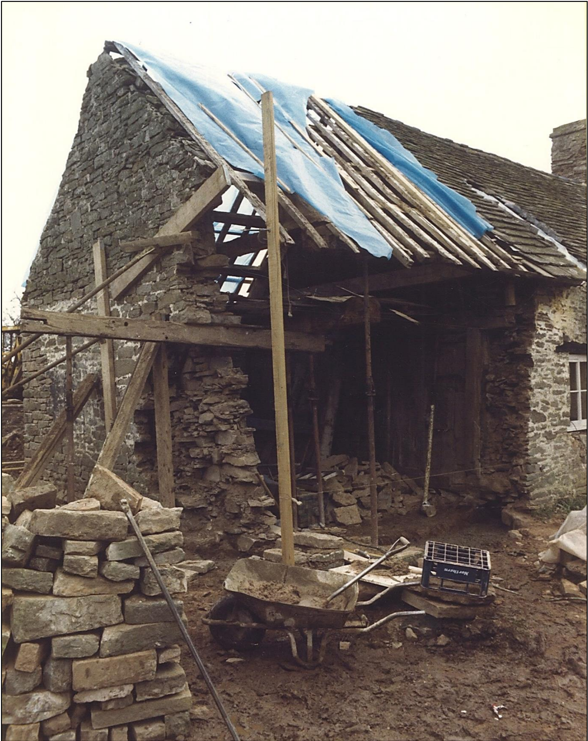
Repairs to the roof and front elevation of the stable/store room.
