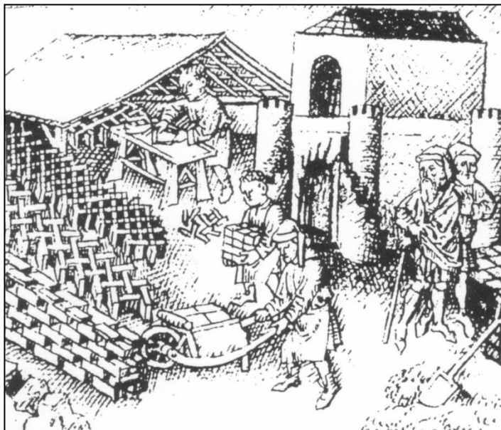
An illumination from 1425, theoretically showing exiled Jews brick making in Egypt, but actually of contemporary practice.
