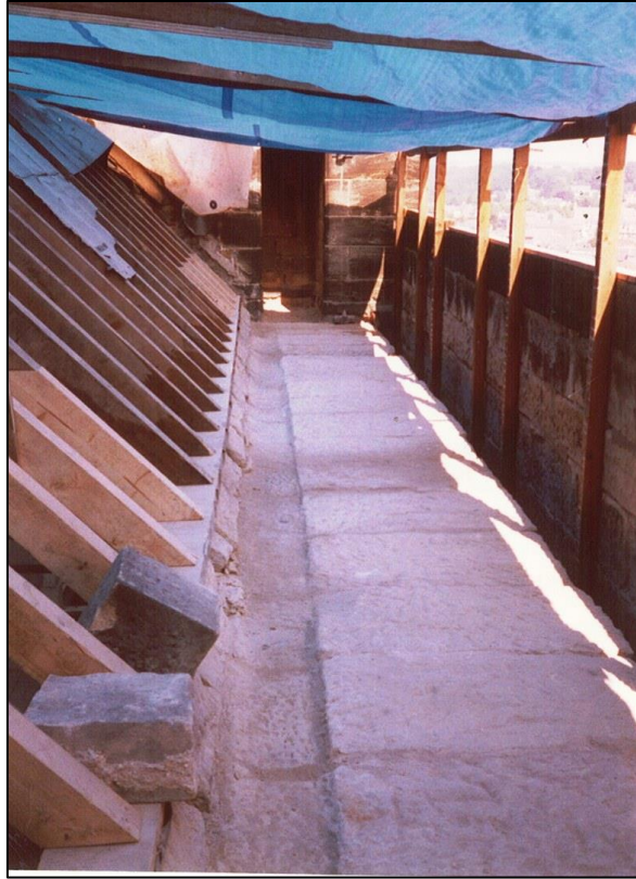
Open day, summer 1990, with roof stripped
