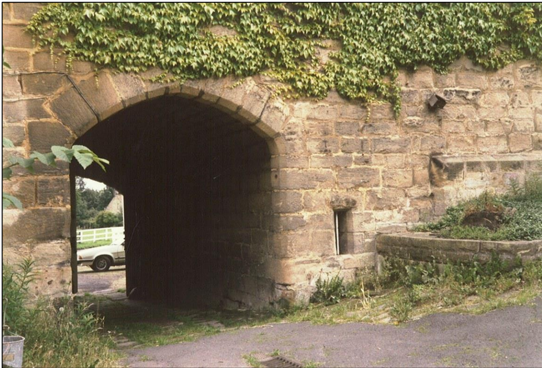
The archway showing the asphalt in the courtyard. 1986
