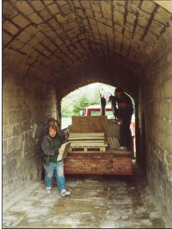
The stone slates for the roof arriving in October 1990
