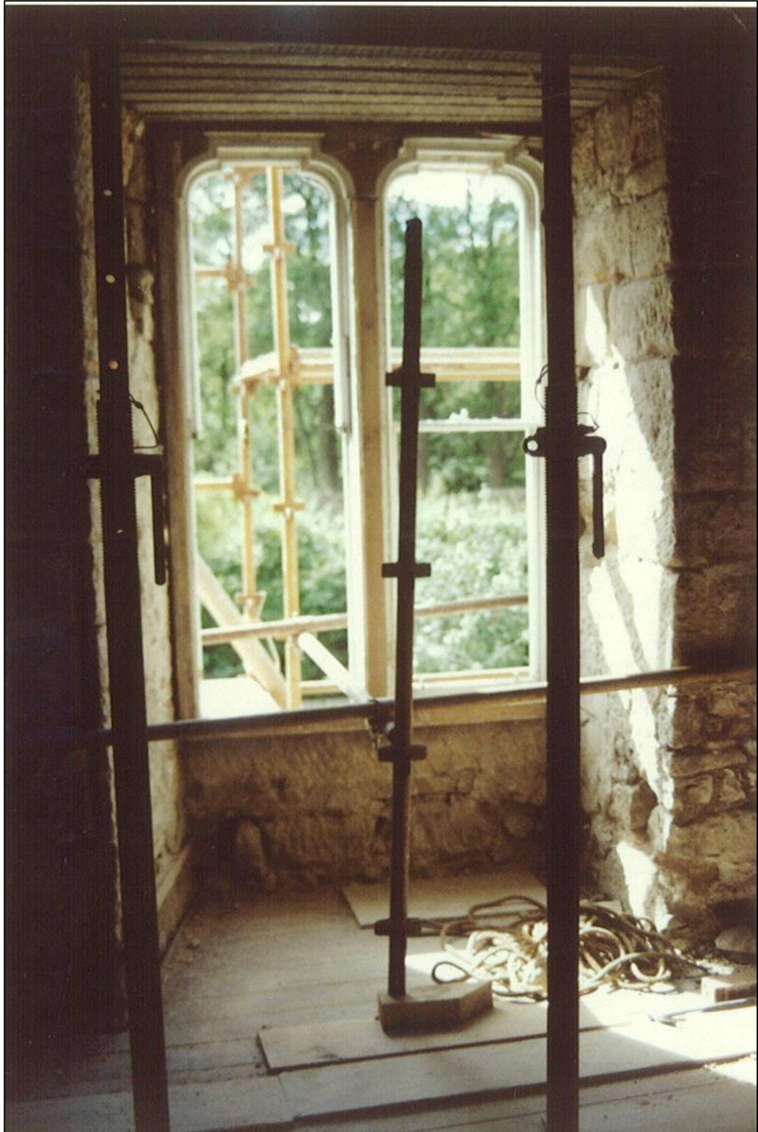
Window onto the second floor passage. The level of the original floor is shown by gaps in the stone work.
