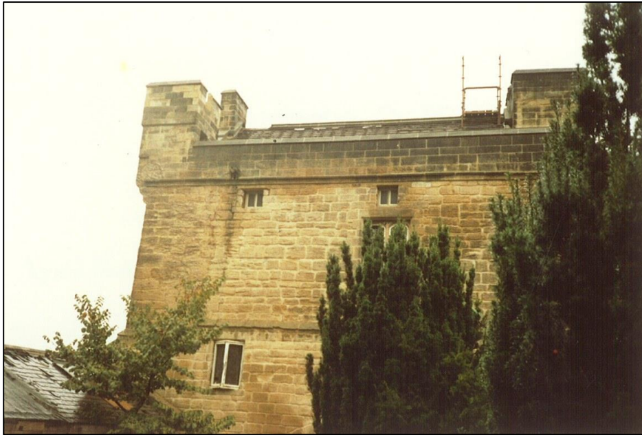
The 17 th century windows as they must have looked. Here they are mock-ups made of cardboard.
