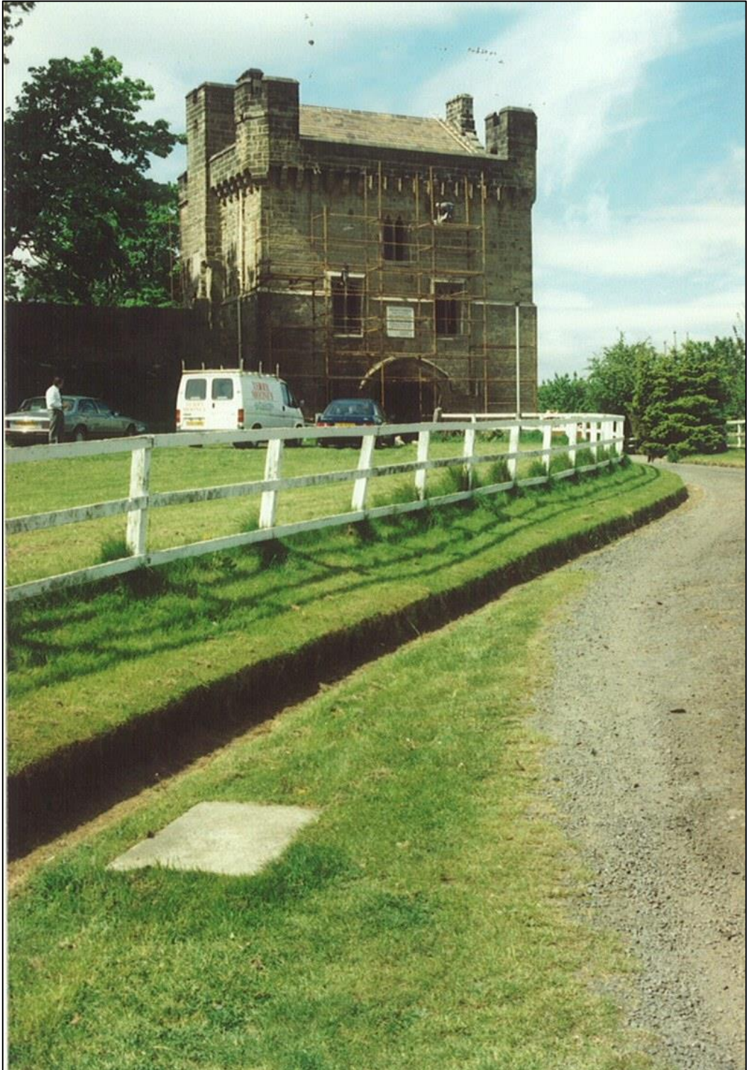
The last of the scaffolding coming down.
