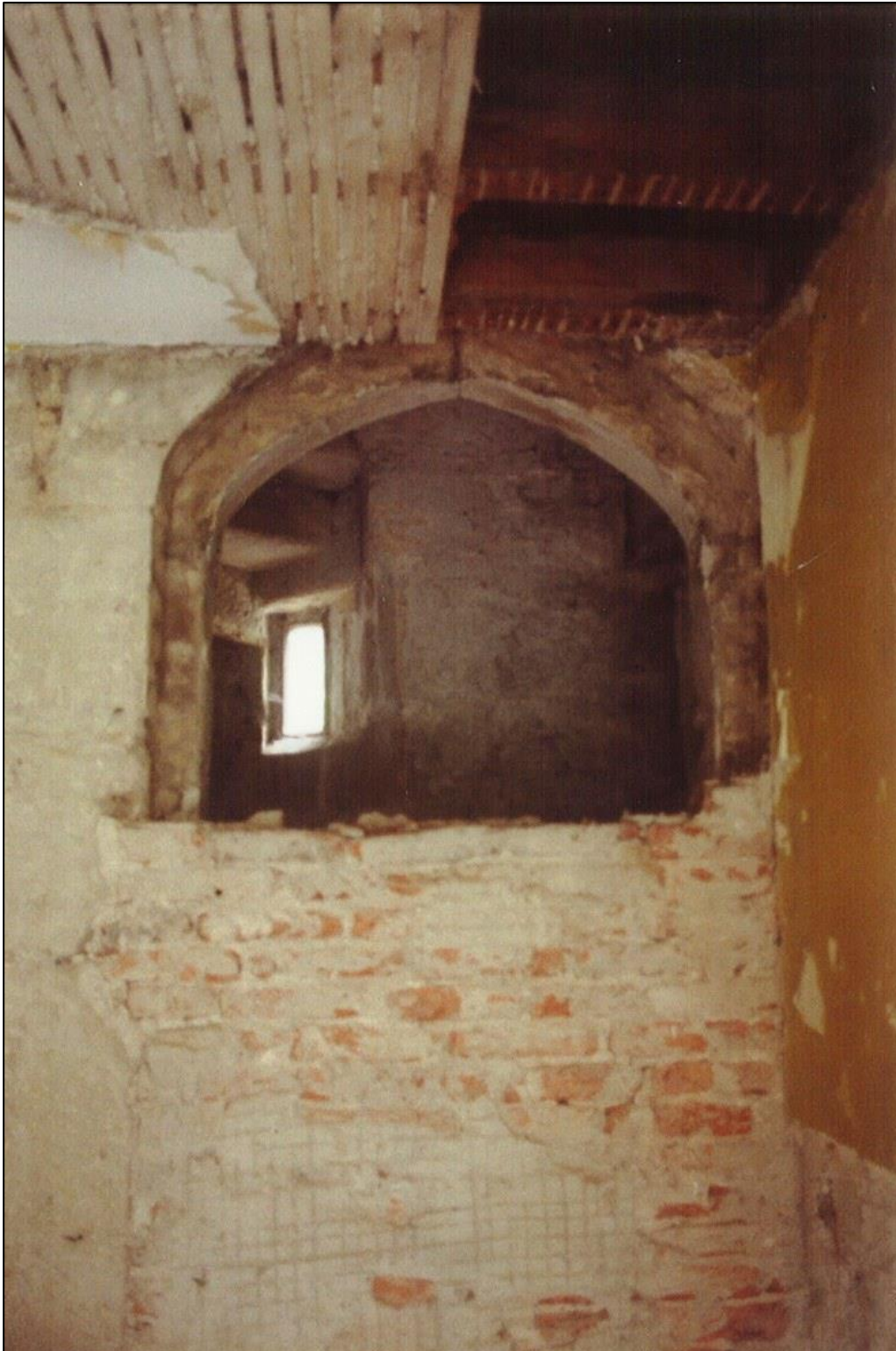
Opening the original doorway from the spiral stairs to the second floor, December 1990.
