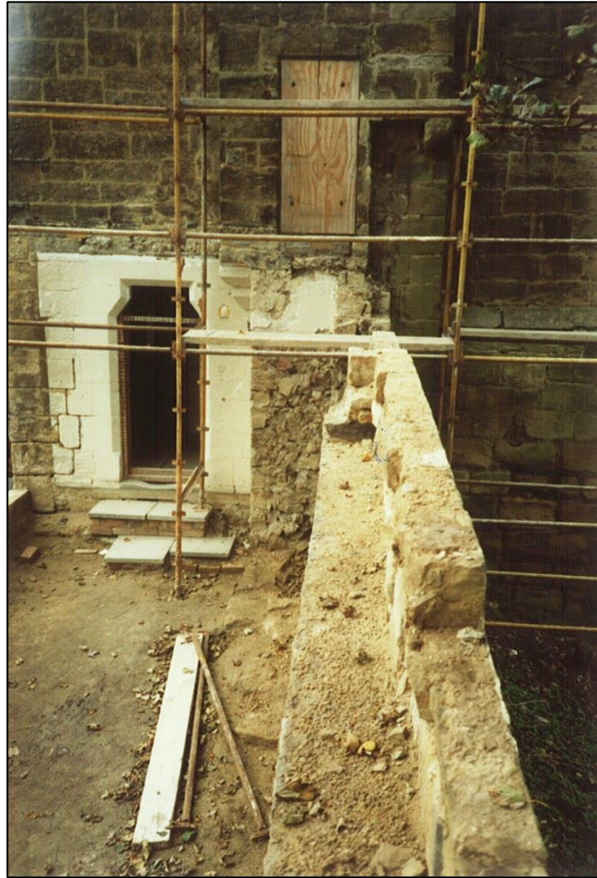
The south extension being removed
