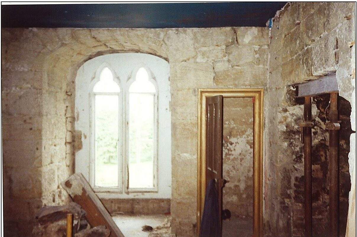
Kitchen end during restoration
