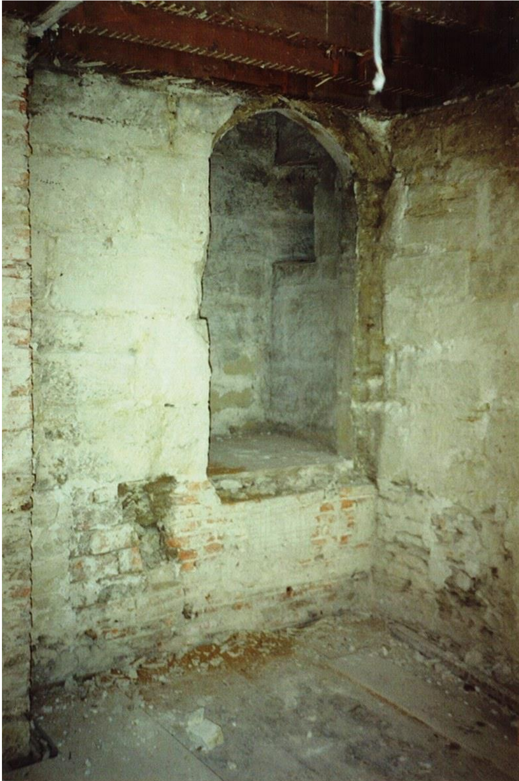
The spiral stair doorway completely open. This is where the shoes were found hidden in the threshold.
