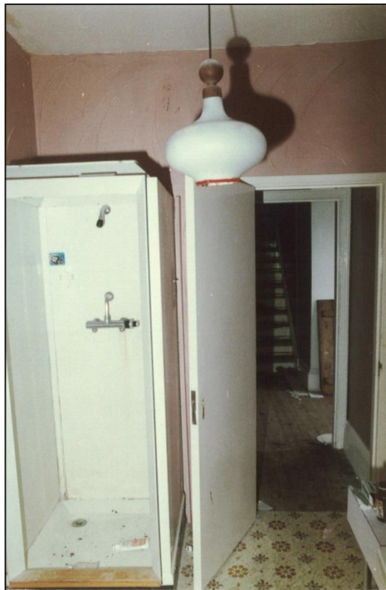
Shows cabinet in present bathroom and old stair (19 th C) up to attic.
