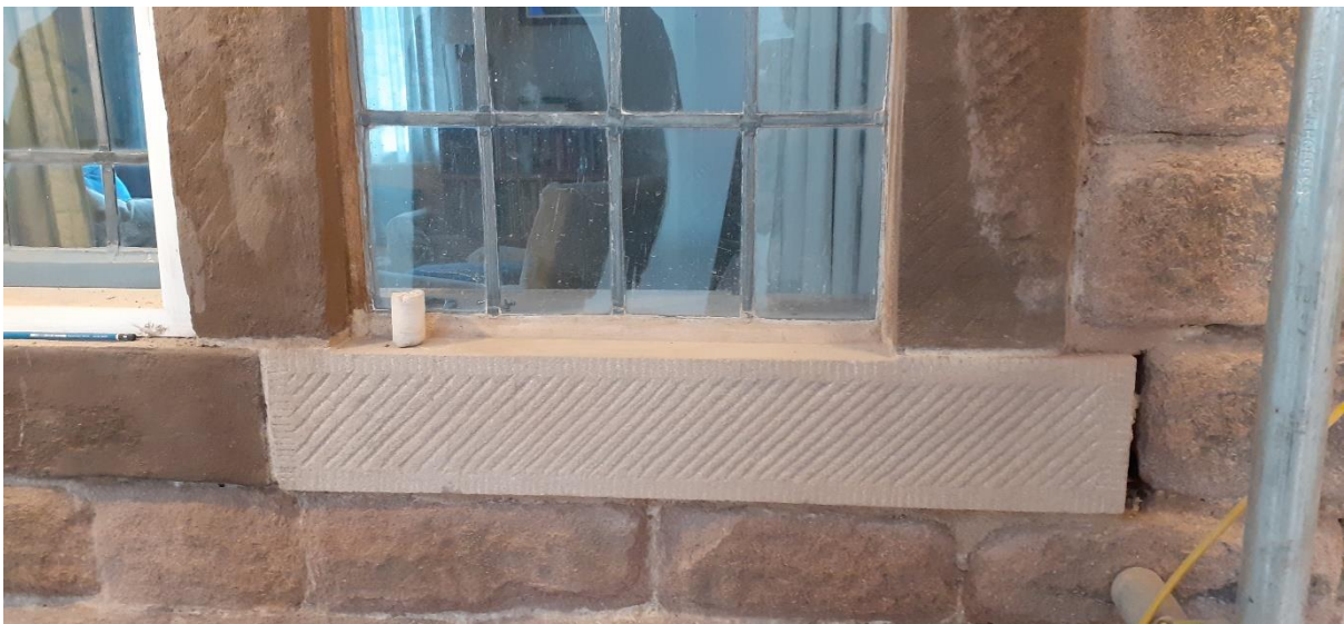
Replaced window sill, with plastic repairs visible as the as yet darker areas in the eroded jambs just above the sill. As they dry, they will be hardly visible.
