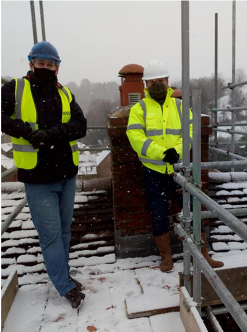
Outside works meant that the project could continue despite lockdown, but the winter of 2020/21 saw some very cold conditions, as here in February 2021 when film maker Mark Todd (left) visited to film the works for Historic England.
