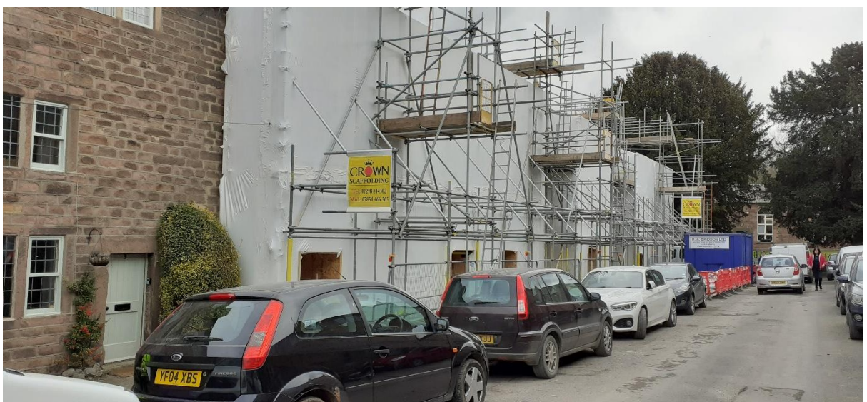
Half the north side of the street had to be swathed in scaffolding from October to March.
