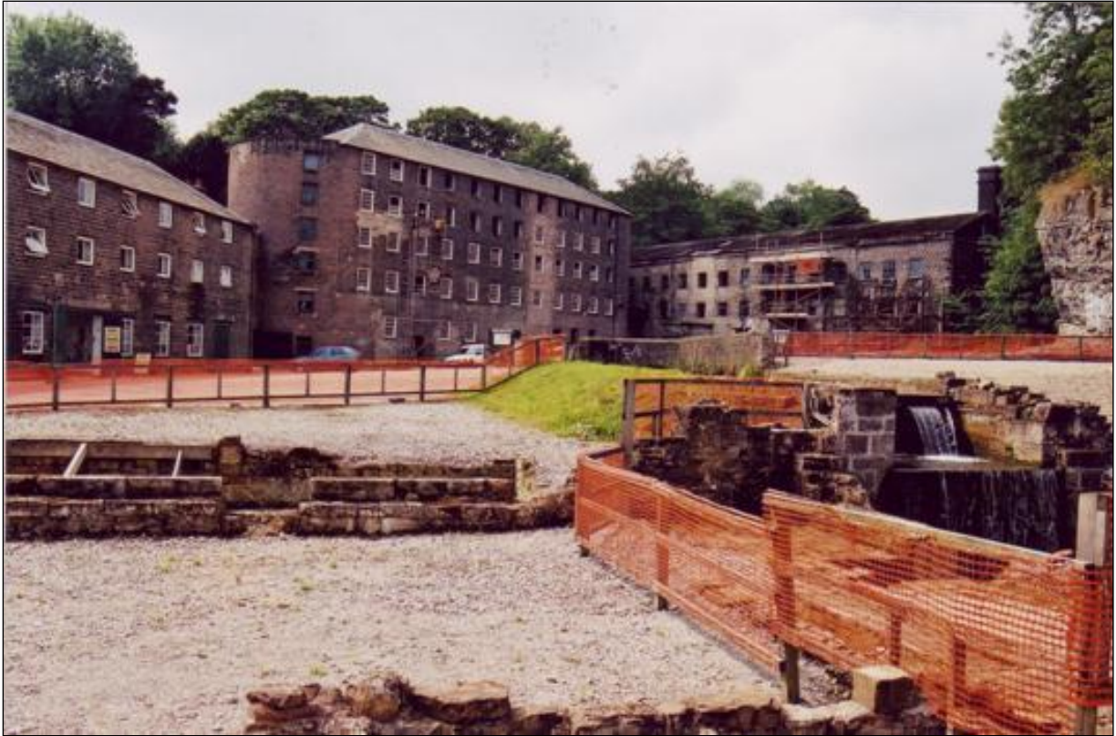
Figure 14: View across all that remains of the second mill, built in 1776, destroyed by fire in 1890. The wheel pit lies to the right, the Bonsall Brook still flowing through. The old packhorse bridge lies between the wheel-pit, with the first mill immediately behind. The later mills run to the left. Facing inwards across the yard, these do not present the same windowless, fortress-like aspect found on the Mill Road Elevations.
