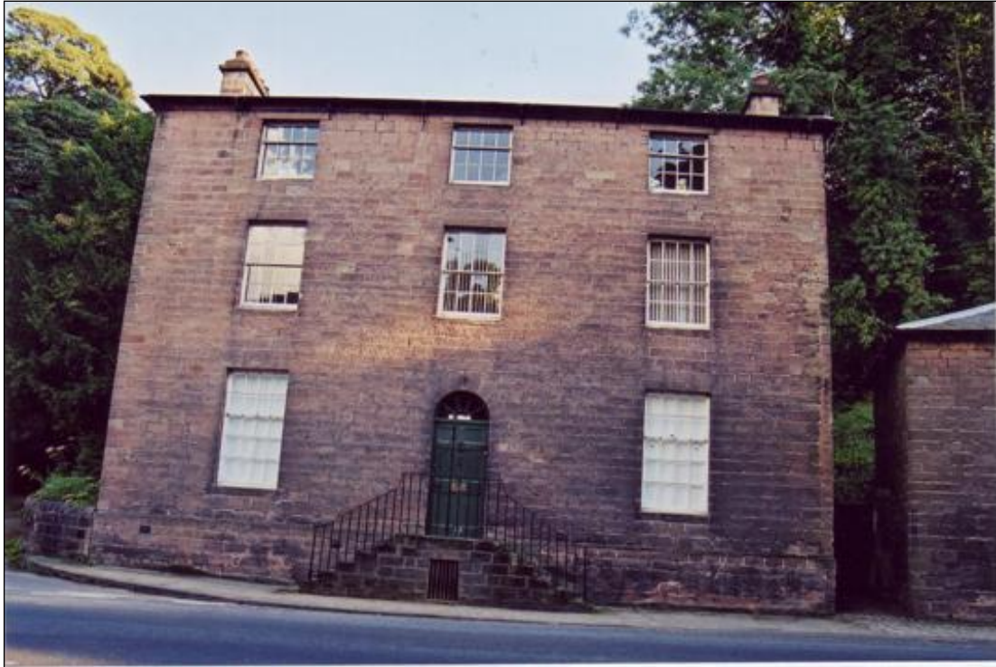
Figure 15: The mill manager's house on Mill Road. It was perhaps here that Thomas Smalley and his family lived before he fell out with Arkwright.
