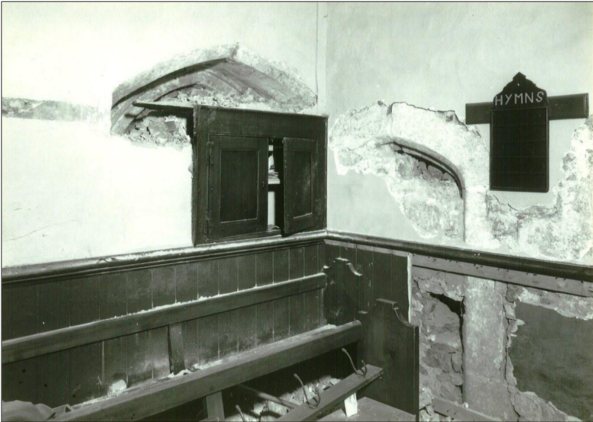
The blocked doorway at the south end of the hall and the staircase door
