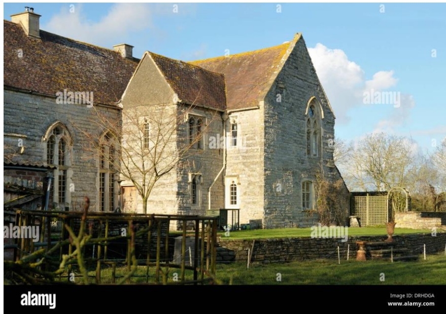
Ashleworth Court, Glos. Hall with oriel projection and solar wing; before 1463. The oriel and solar wing at Croscombe was probably very similar to this house in Gloucestershire. The window tracery is also very like that of Old Hall.
