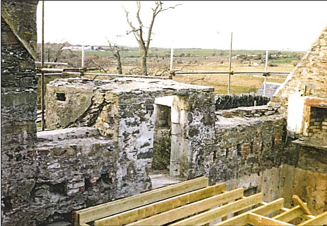
The top of the spiral staircase without its roof, and the first floor ceiling being replaced at its original level; it had been raised in the 19th century.
