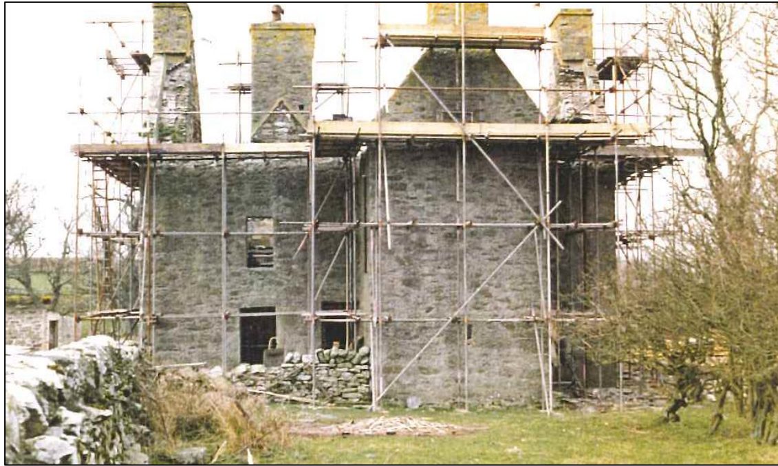
The roof timbers were beyond repair and are new, but the slates were either re-used or replaced by old slates from the steading.
