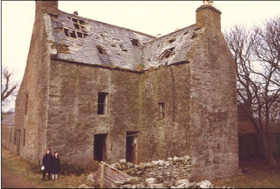
The original dormer windows were removed in the 19th century and replaced by skylights, but their bases could still be seen in the external masonry and they have been rebuilt in stone, in as similar a style as possible to the originals.
