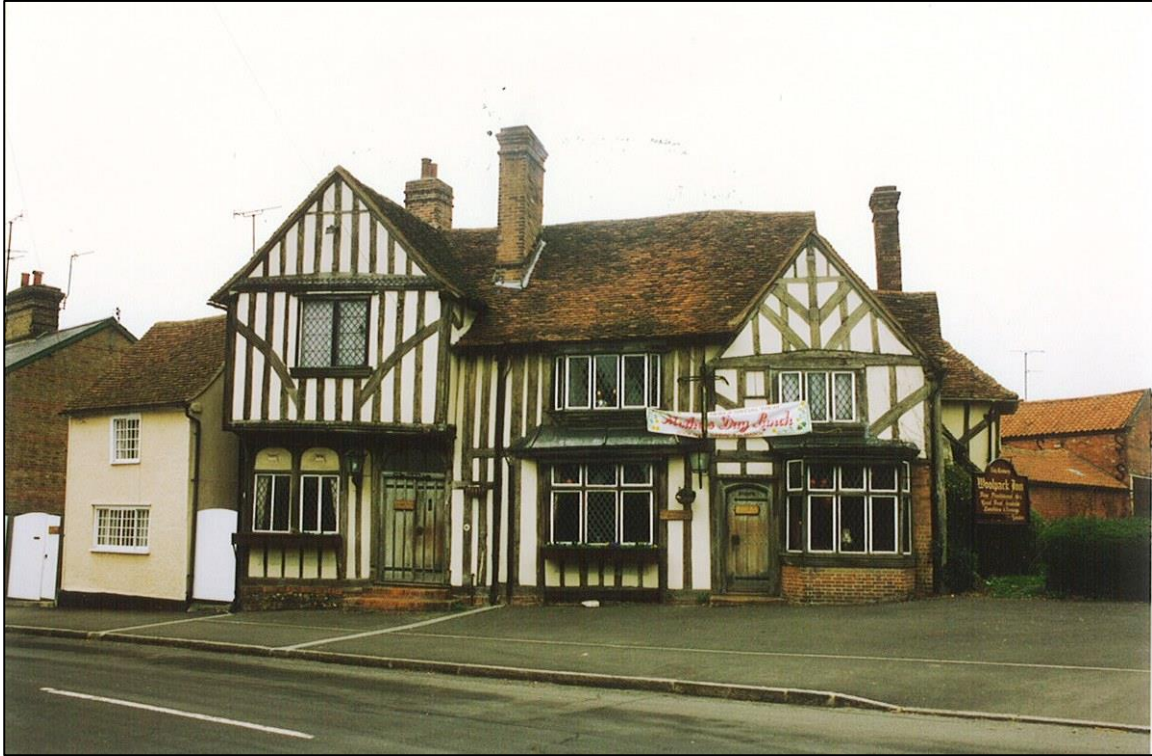
The Woolpack Inn, Coggeshall – the ground floor on the left hand side shows two shop windows and then the narrow coffin door.
