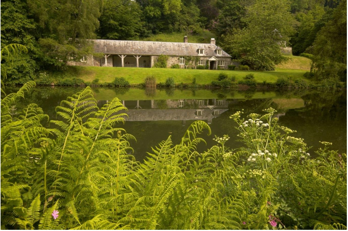
Dairy Dell: Pond Cottage with the Dairy behind.
