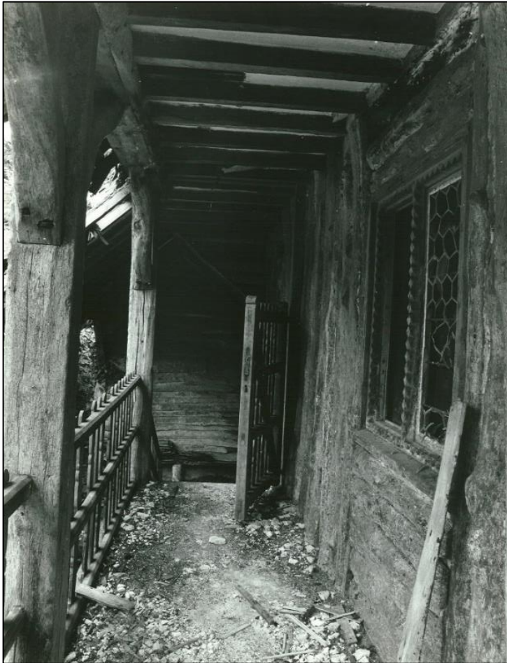
The top of the external stairs in 1977.
