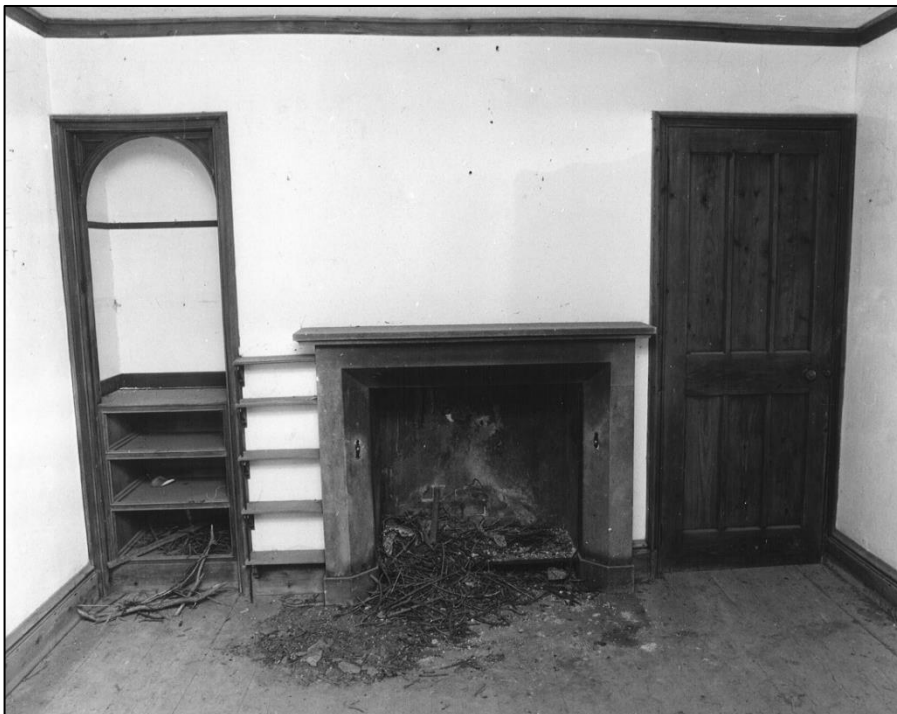
The attic bedroom before restoration
