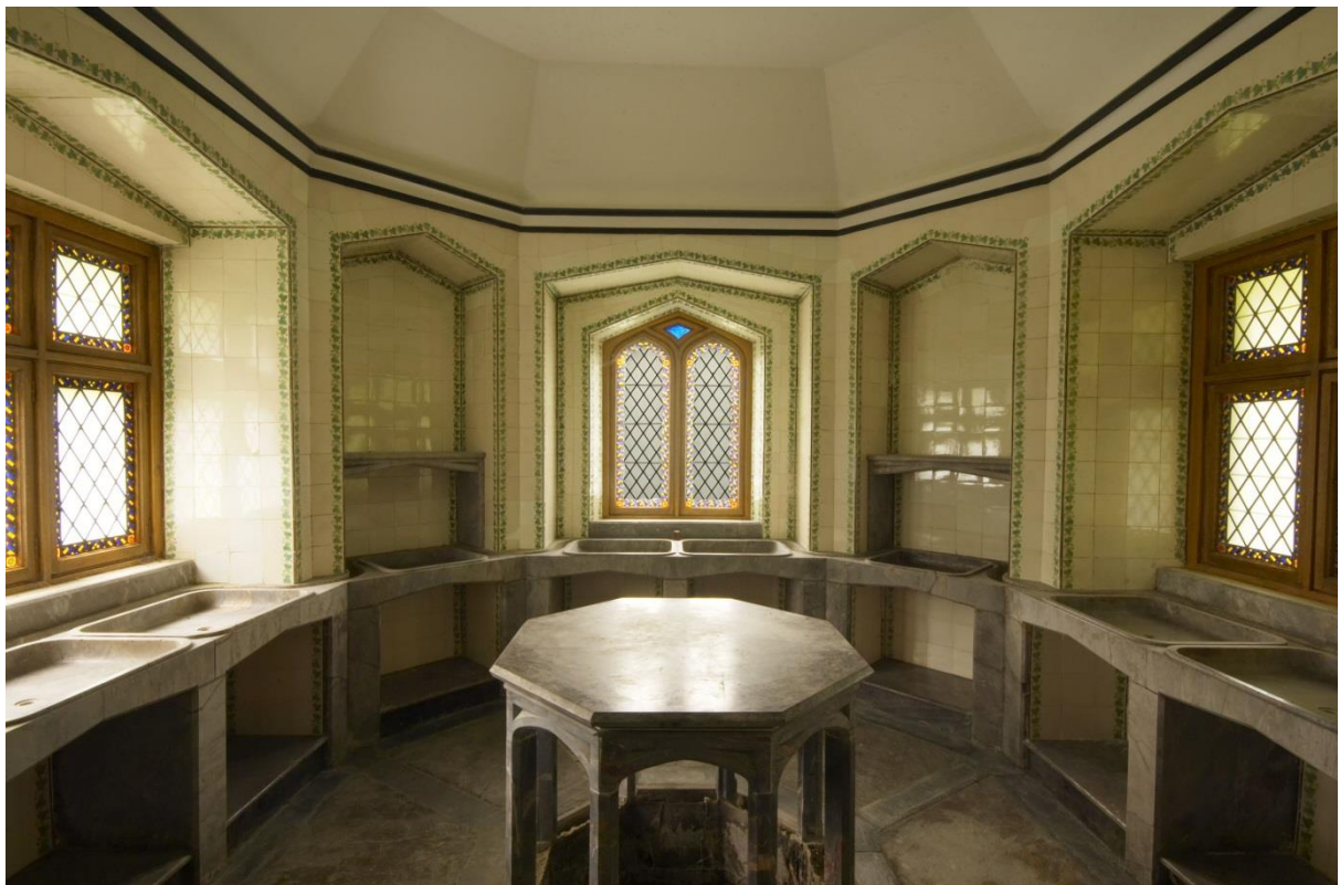
Inside the Endsleigh Dairy, before and after restoration. Note the ivy leaf pattern tiles edging the windows and alcoves.
