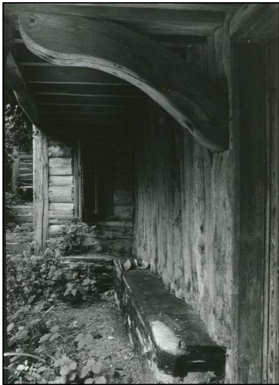
The fixed external bench during restoration
