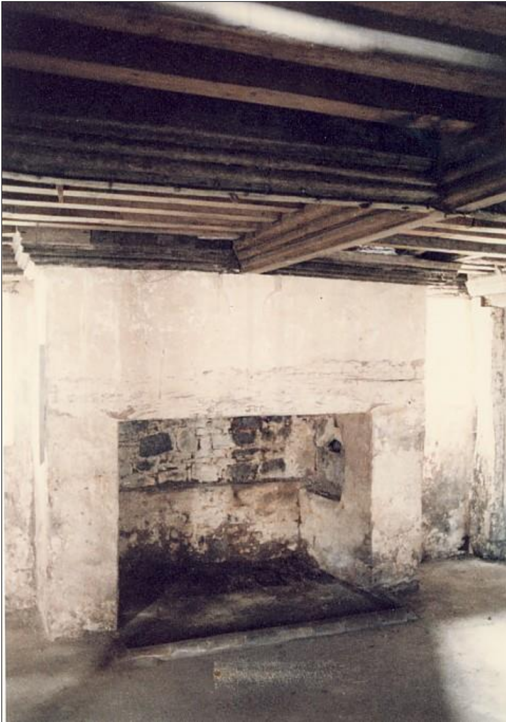
The ground floor 'parlour' fireplace in 1983 (today's sitting room). This would have heated a relatively high status meeting room (note the moulded ceiling timbers).
