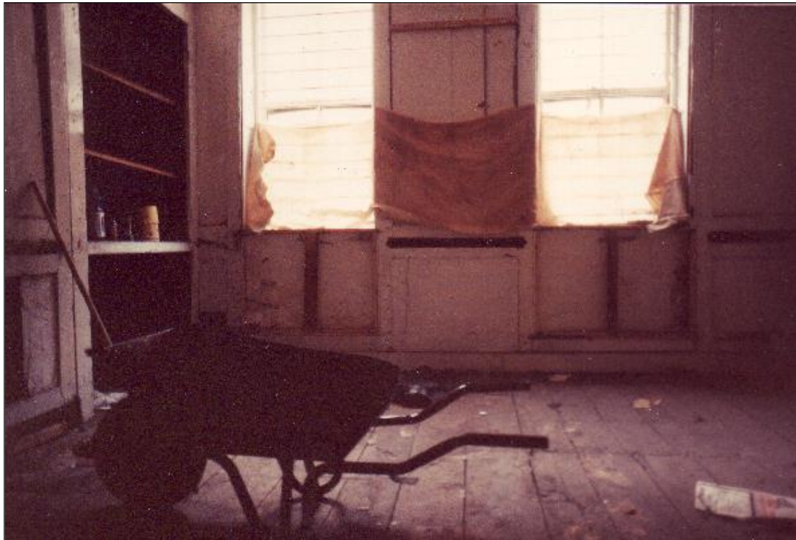
Ground floor, front room before restoration.
